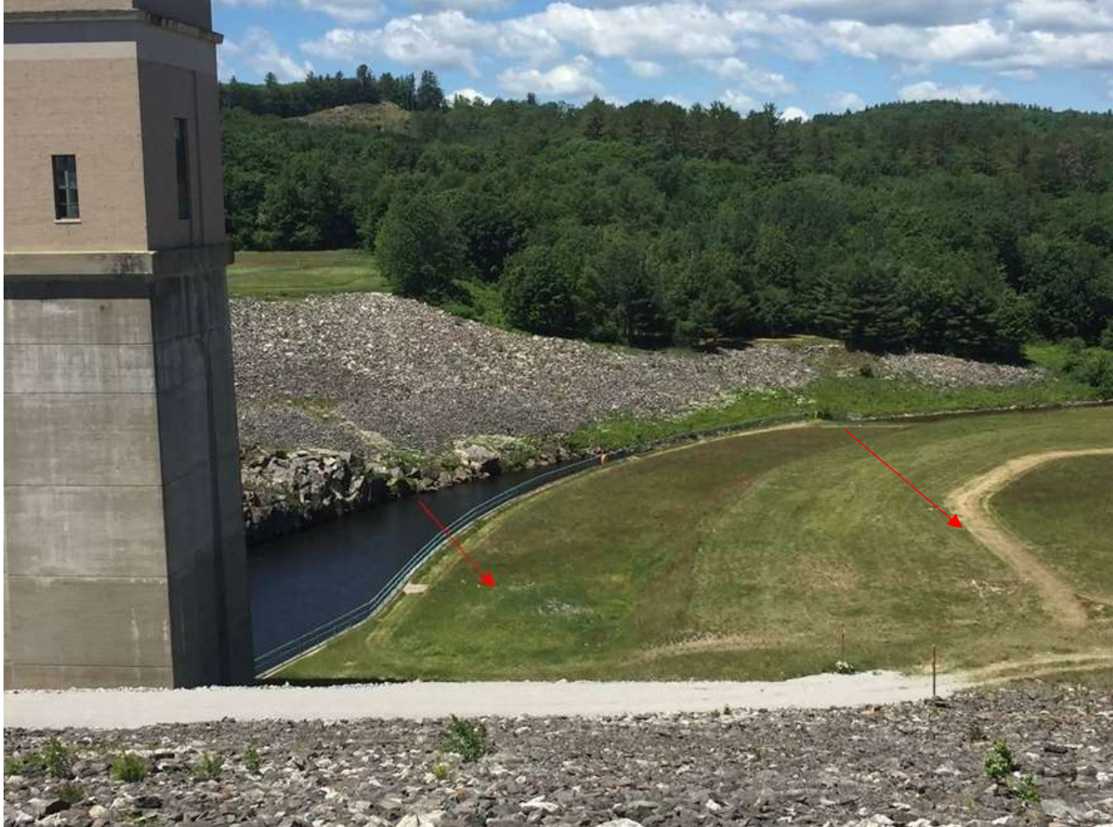
Photo #2: Crane set up pads are located on the east river bank right below the gatehouse. The red arrow is an approximate location. The photo is intended to provide context to the nature of the work. Arrow closest to the dam indicates crane set with maximum 110-ton capacity. Arrow in the upper portion indicates approximate crane set up if crane is larger than 110-capacity crane.
