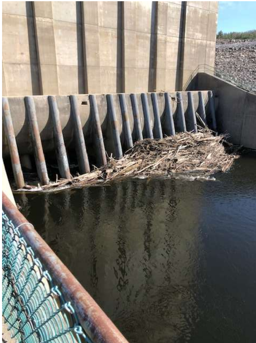
Photo #1: Debris at the Franklin Falls Dam trash rack on May 8, 2019. Pool level is 313.64' elevation, concrete bib is at 300' elevation. The photo is intended to provide general idea of what is in the trash rack. Any estimate of quantity or type of material should be determined during a site visit prior to the submission of a quote.
