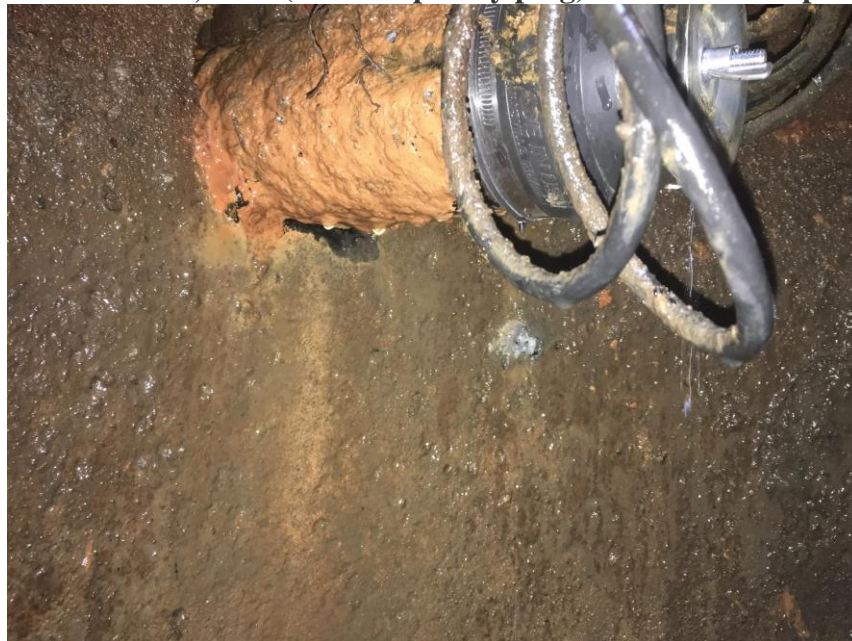
Informational Photo #5, Inlet (with temporary plug, note rocks at top side of pipe)
