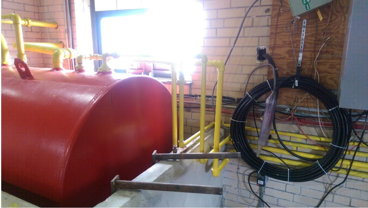
Informational Photo Number 2: Fuel pipe connections
