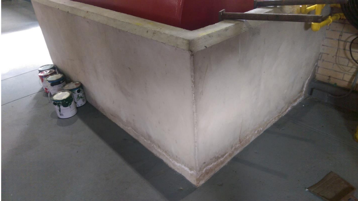
Informational Photo Number 3: Secondary containment wall.
