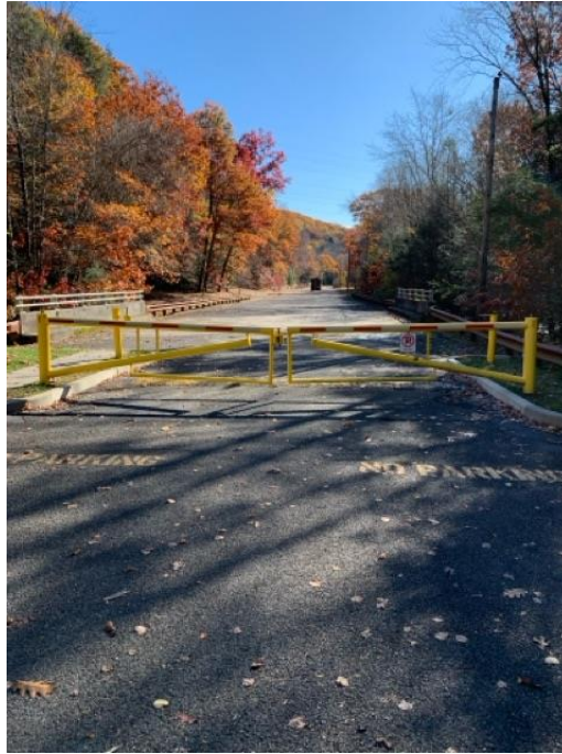
Informational Photo 7: Example of gate to be installed at Black Rock Four Corners.
