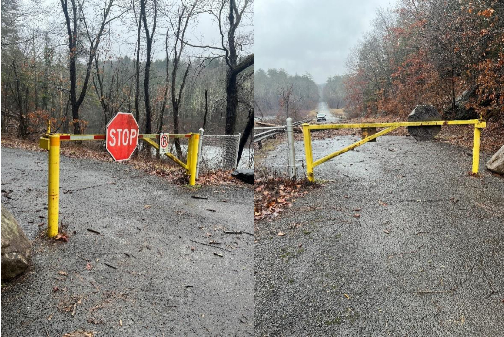
Informational Photo 6: Existing Gate at Black Rock Dam Outlet.
