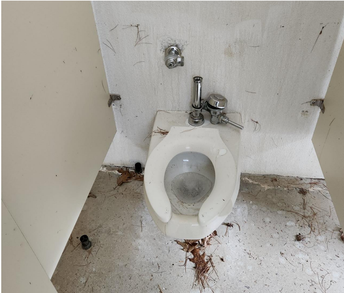
Exhibit 2: Example of a toilet flushometer and flush valve assembly to be reconnected during the de-winterization service and disconnected during the winterization service.
