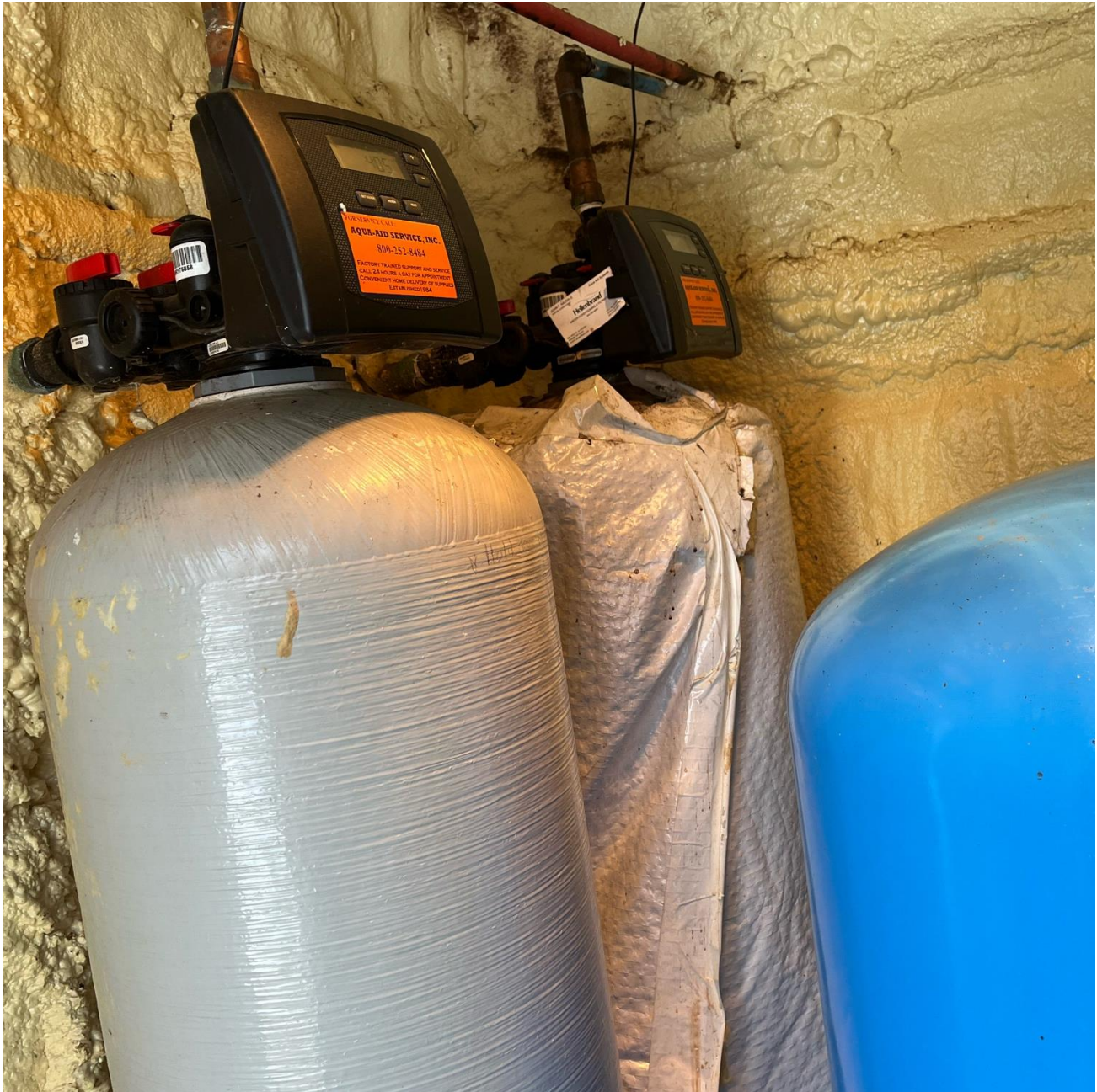
Exhibit 4: Existing water sediment filtration systems located in the well pump house.
