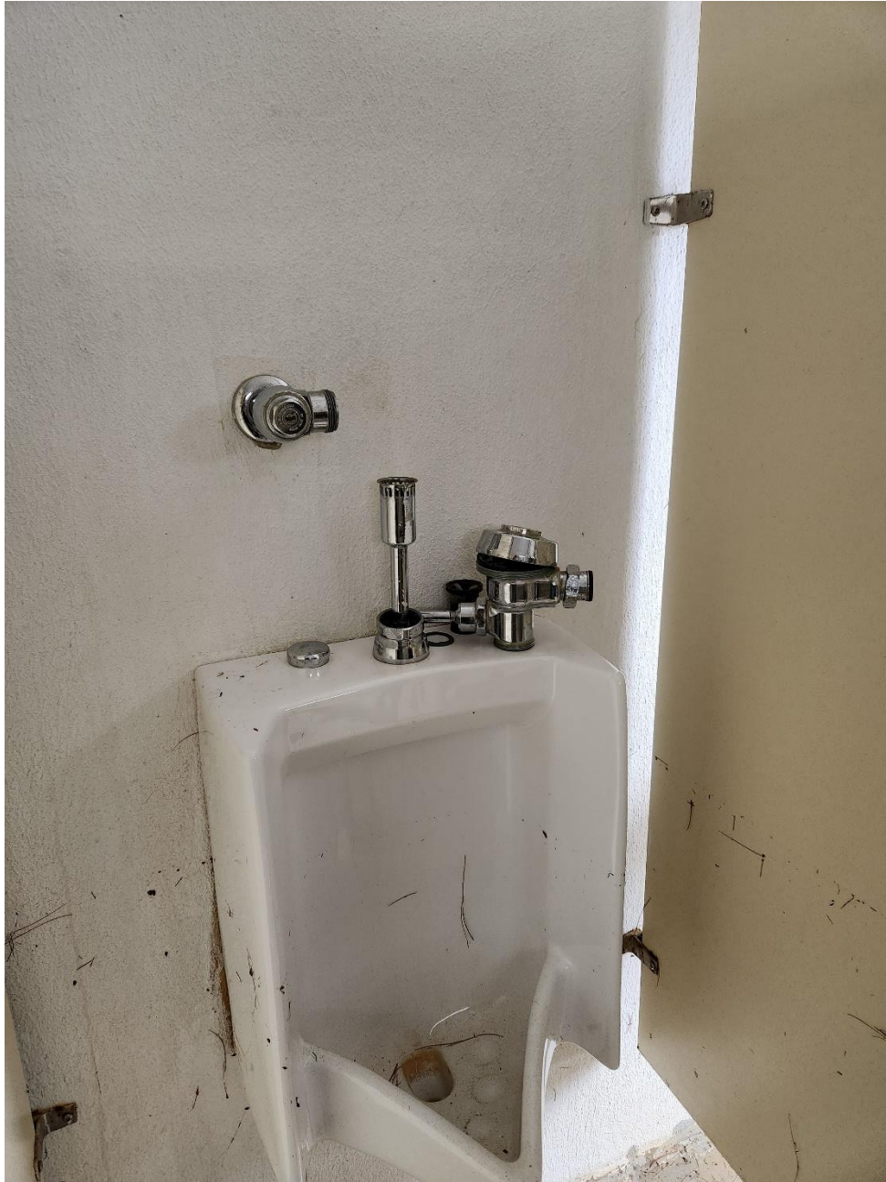
Exhibit 3: Example of a urinal flushometer and flush valve assembly to be reconnected during the de-winterization service and disconnected during the winterization service.
