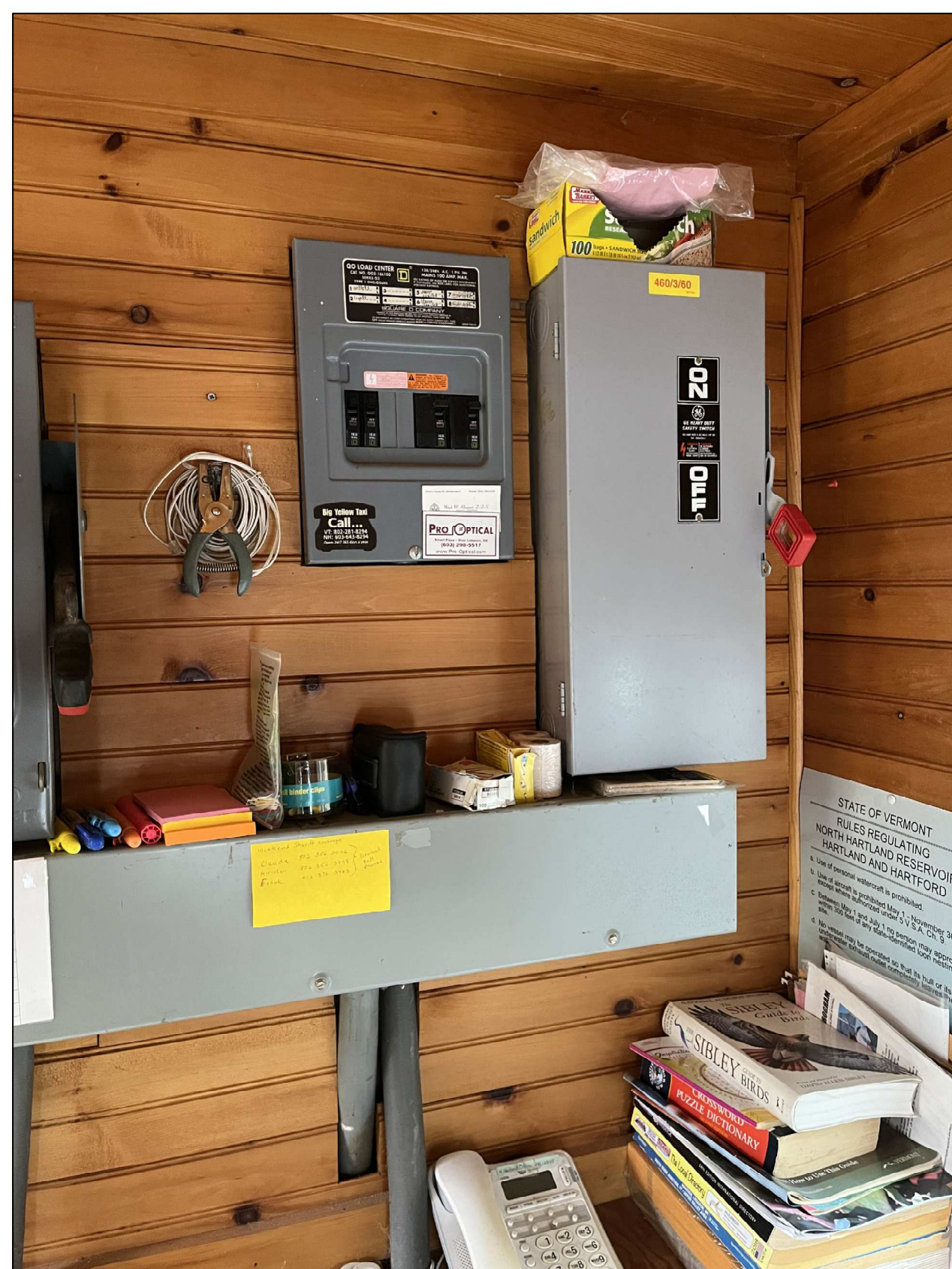
EXISTING WIREWAY, PANELBOARD & RV SITE DISCONNECT (GUARD BOOTH)
