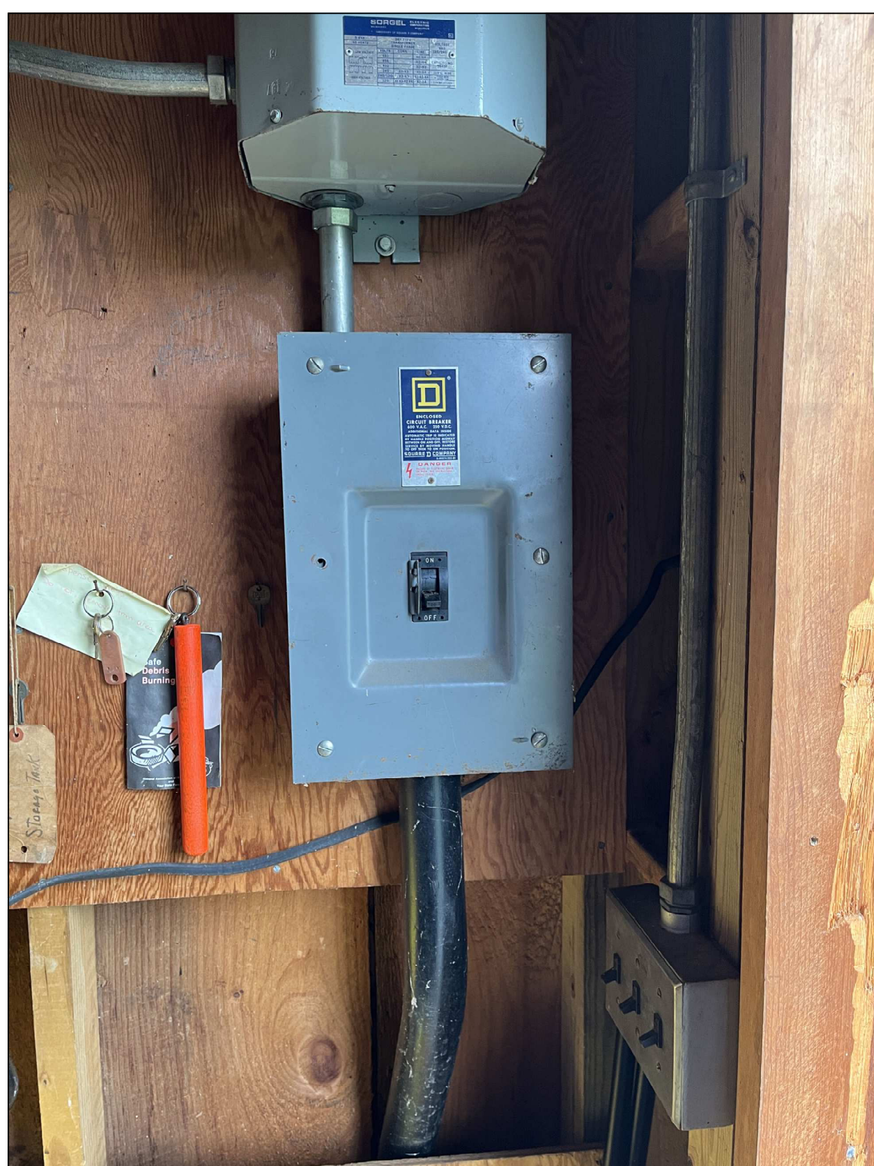
H8 EXISTING TRANSFORMER PRIMARY DISCONNECT (REST ROOM) SCALE: N.T.S
