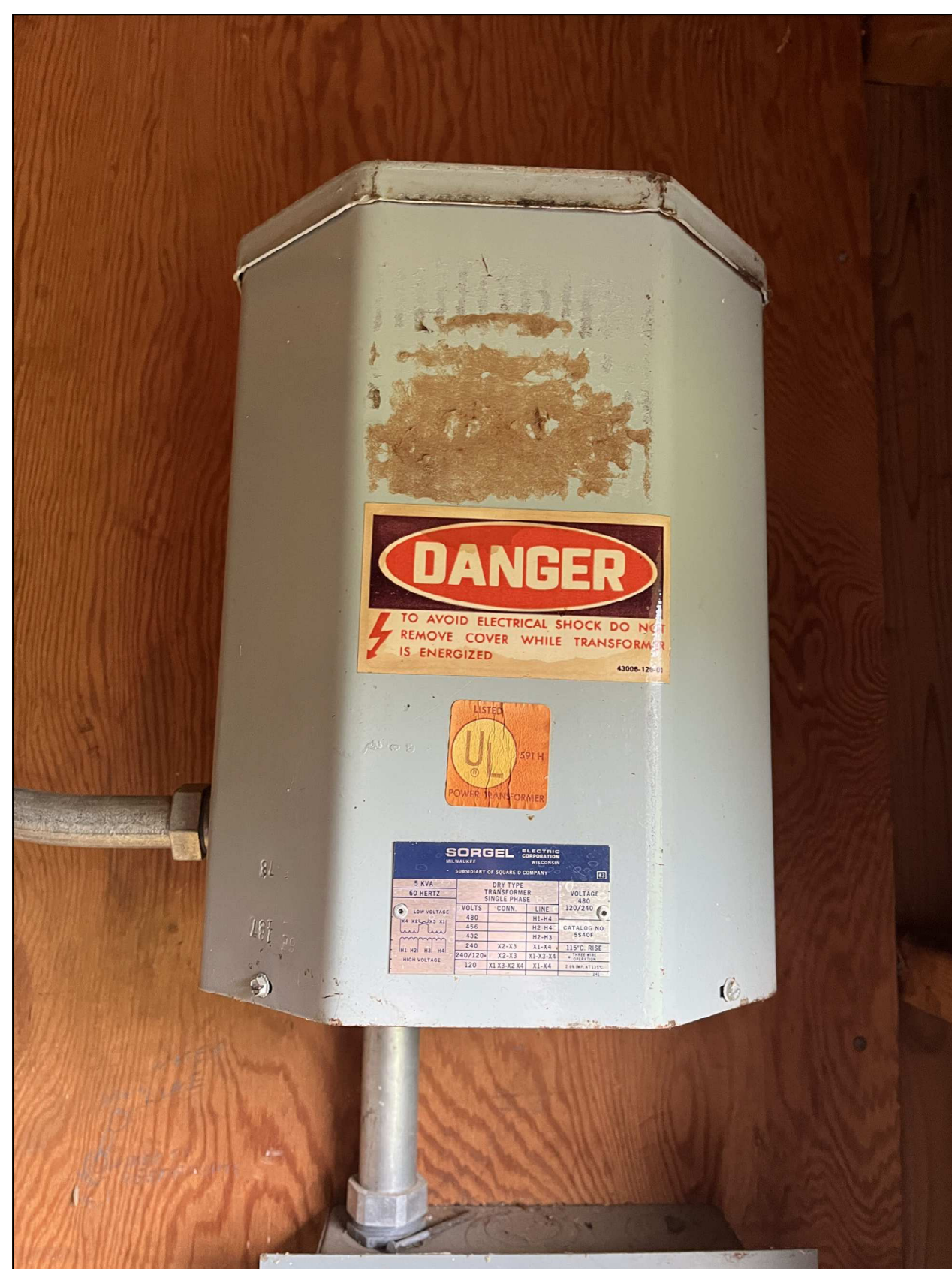
EXISTING 5KVA TRANSFORMER (REST ROOM)
