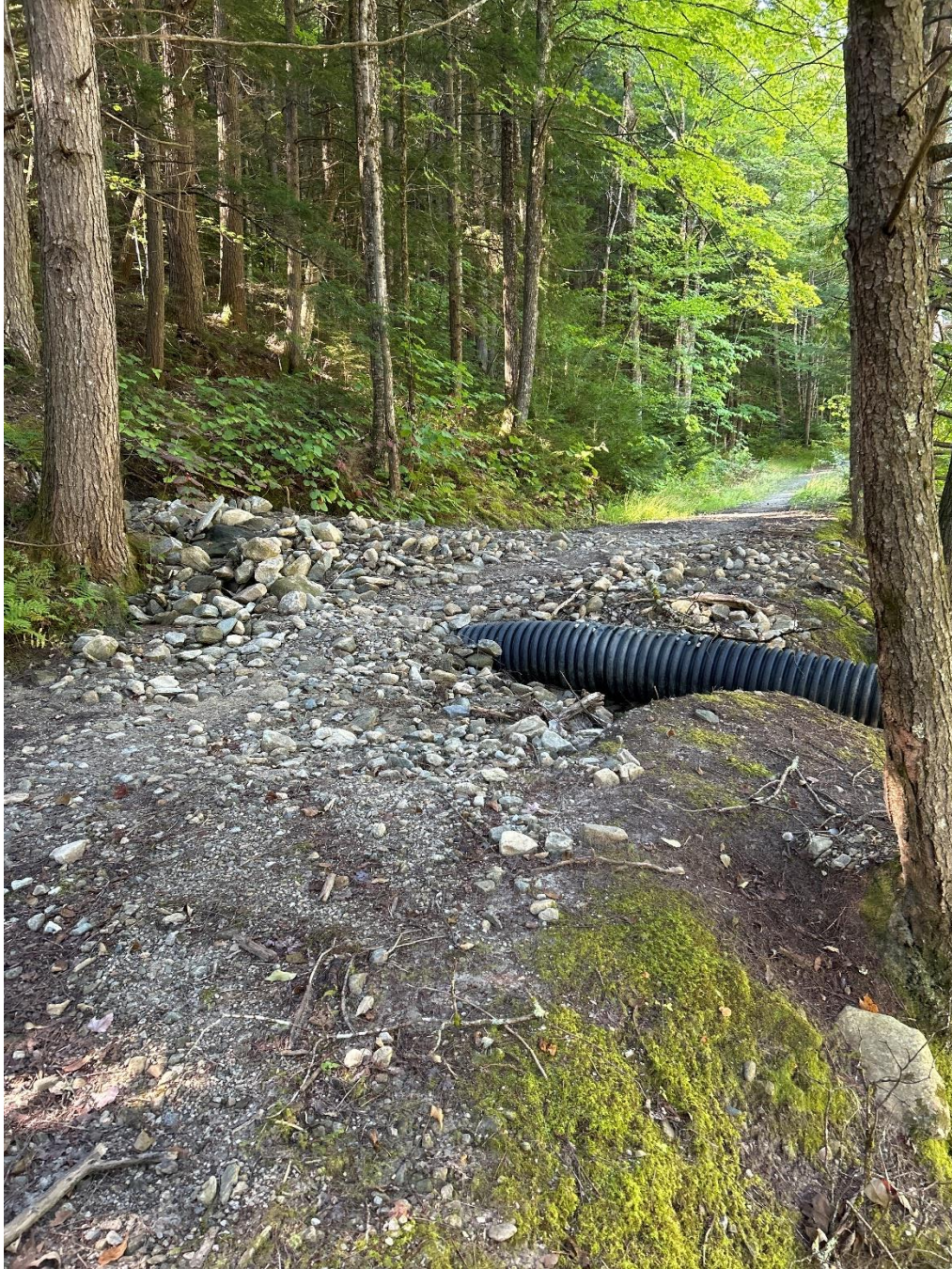
Informational Photo 7: Site #2- Cohen Road clogged culvert.
