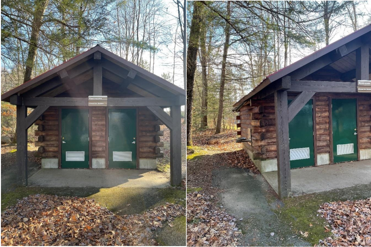
Informational Photo 4: Log Cabin Restroom and Drinking Fountain.
