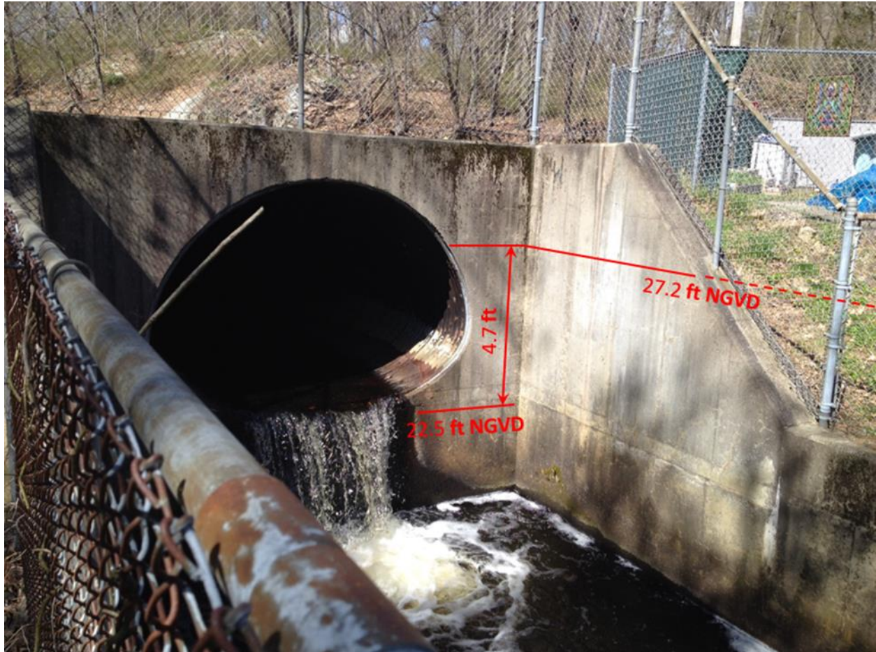
Figure 1: Expected Water Level in the Stilling Basin Under Alternative 2, with a Flow of 600 cfs.
