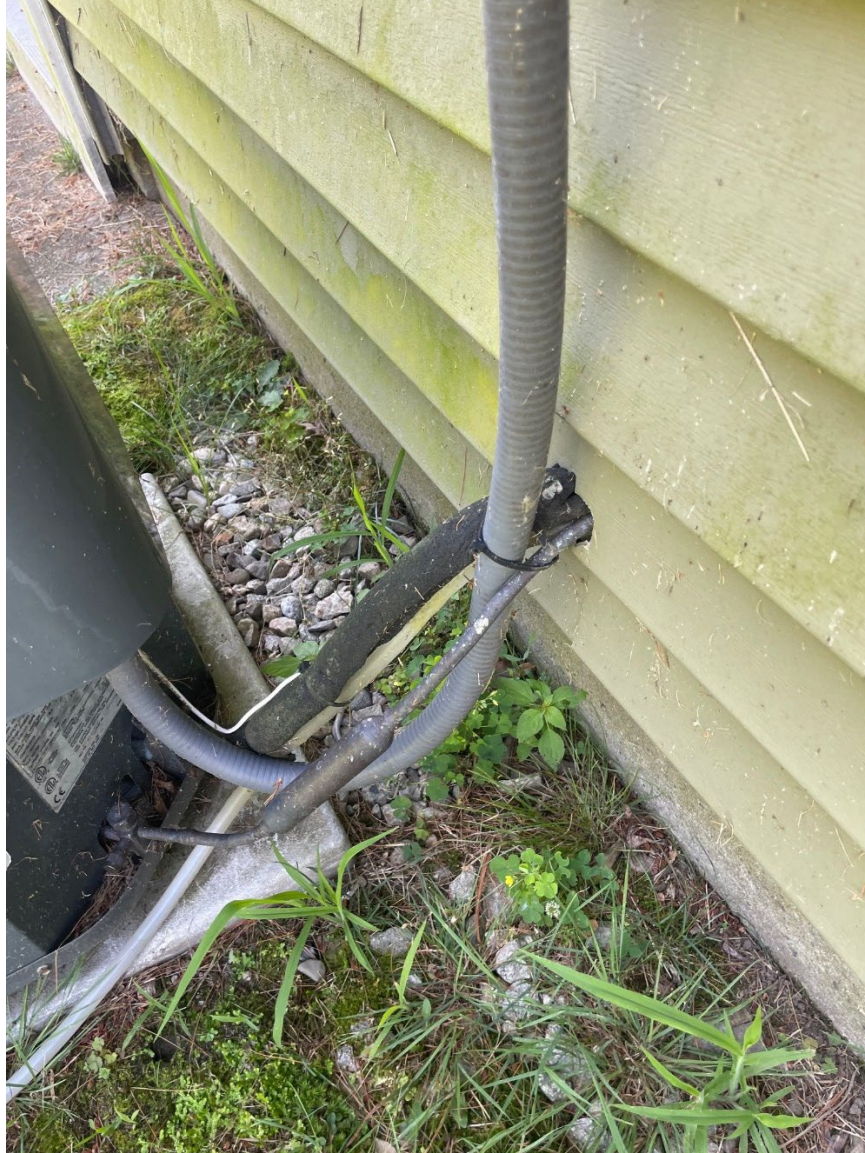
Image of AC Condenser lines where they enter the building.
