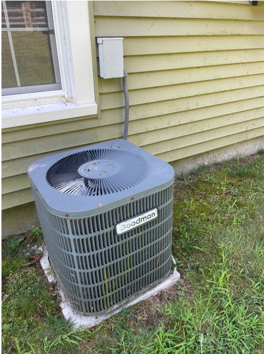
Image of current Goodman AC condenser and pad.
