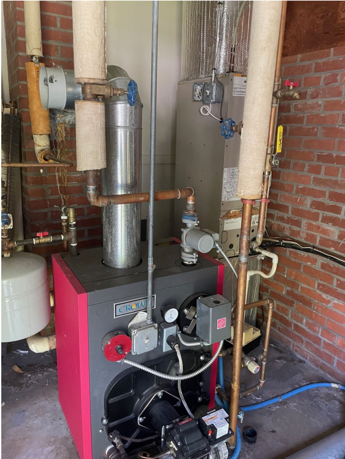
Image of current Oil boiler
