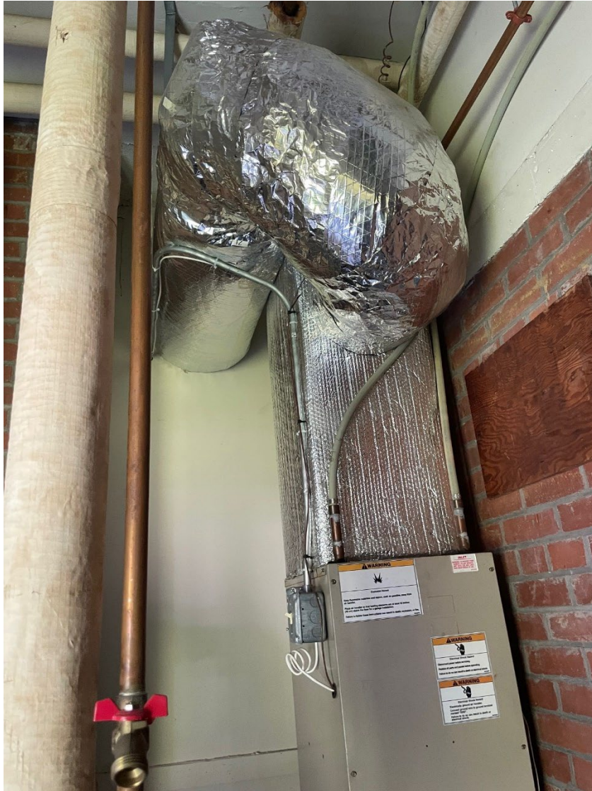
Image of existing air handler and duct work
