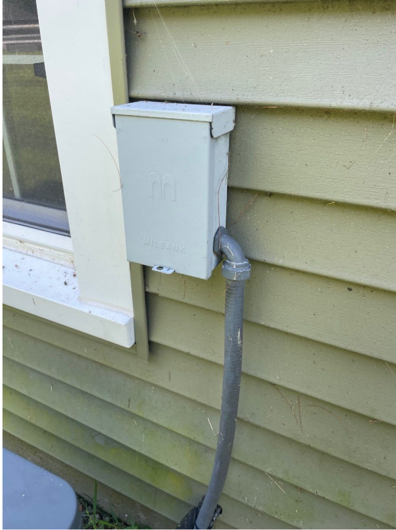
Image of the exterior wiring locking disconnection box.
