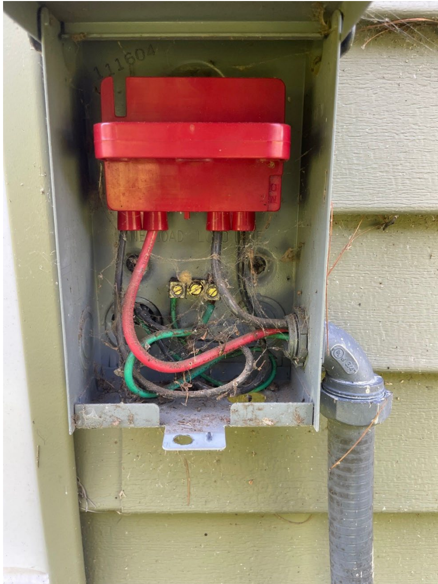
Image of inside of exterior wiring disconnect.
