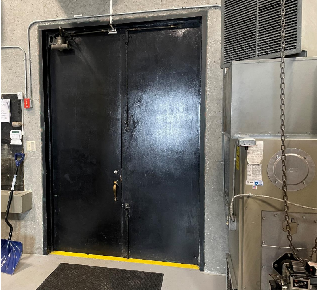
Photo 3: Image showing the backside of the gatehouse doors.
