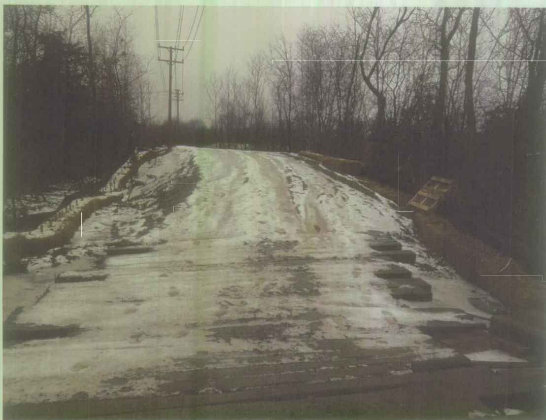
(4) Access crossing between Wetlands A & B, looking W from landfill edge.
