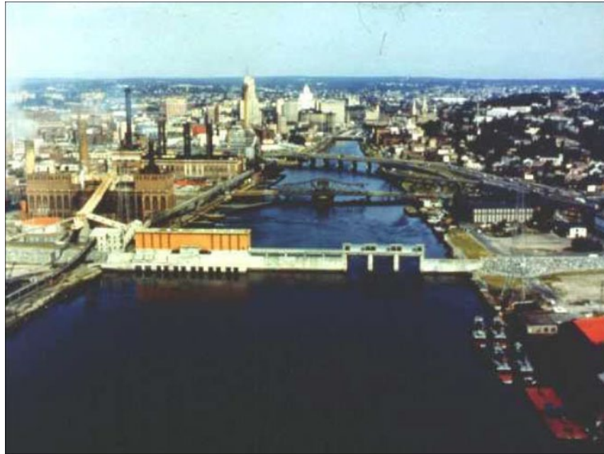
Figure 4. Fox Point storm surge barrier system with Providence in the background.
