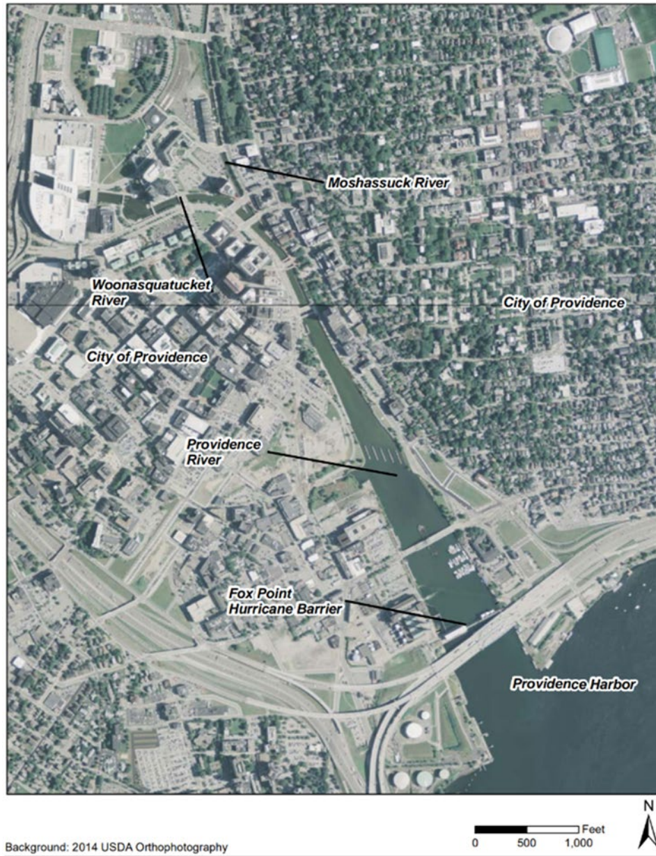
Figure 16. Fox Point storm surge barrier and vicinity.
