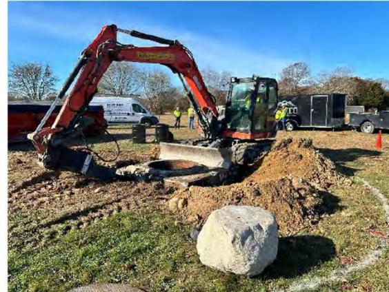
Removing the top of the vault using the mini-excavator.
