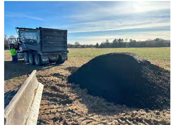
Imported clean loam used as backfill.
