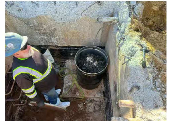
Placement of muck within base of vault into 55-gallon drum.
