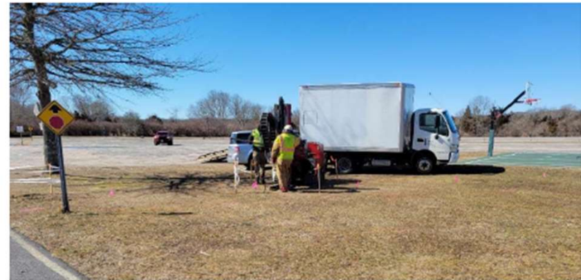
SCENE: View of Geoprobe Direct Push Technology activity at a Boiler House No. 3 (BH3) boring location. DATE: 02 March 2021
