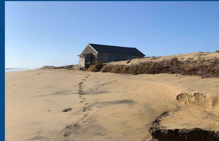
Structures Damaged December 2023
