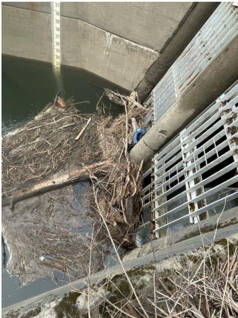
Informational Photo 3: Example of debris in the intake at Union Village Dam. For informational purposes.
