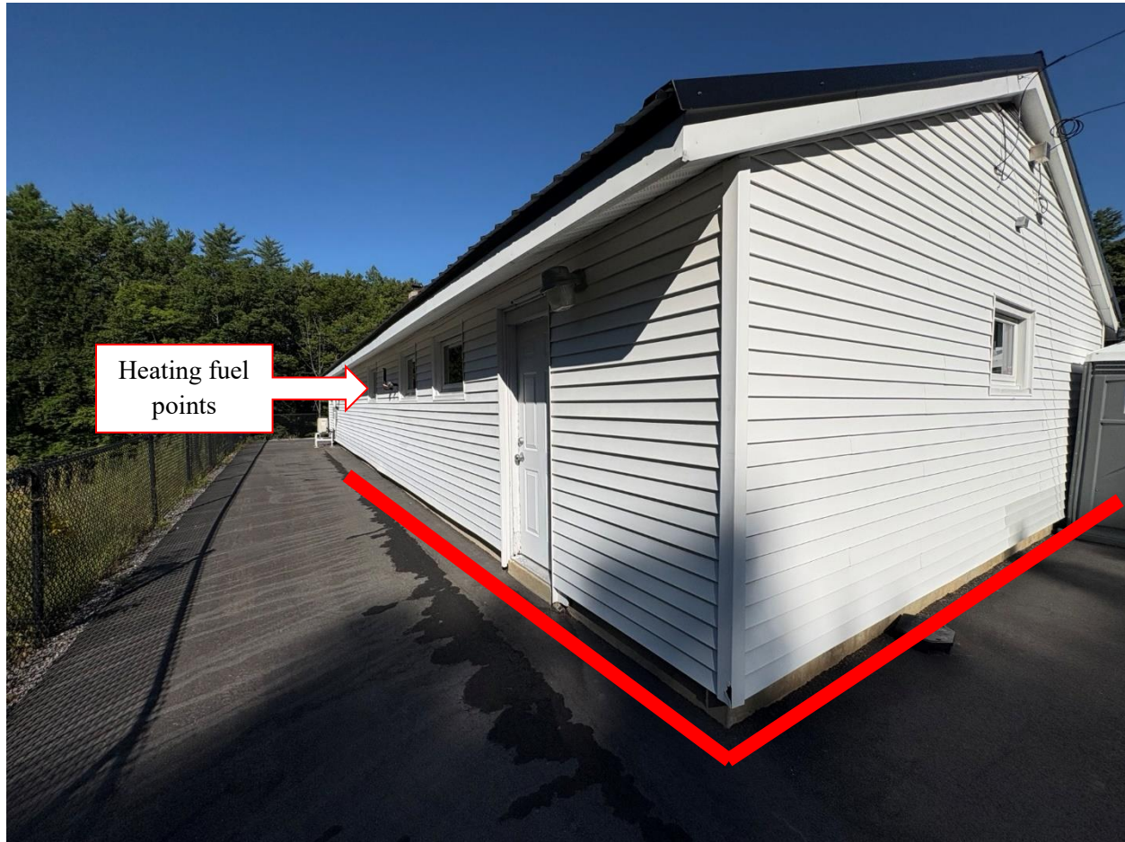
Informational Photo 2: Snow shoveling services are required in front of all buildings, including doors and in front of all heating fuel fill points at the maintenance building.
