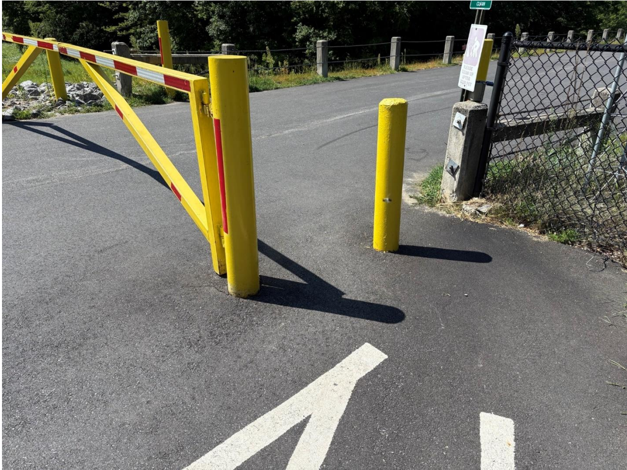
Informational Photo 3: Snow shoveling services are required around the front access gate posts and arms. A path shall be shoveled around the posts for safe public access.
