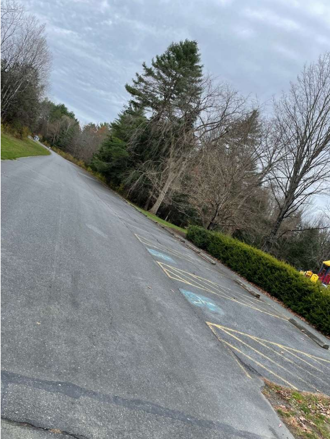
Photo 2: Upper Shelter Parking Lot.
