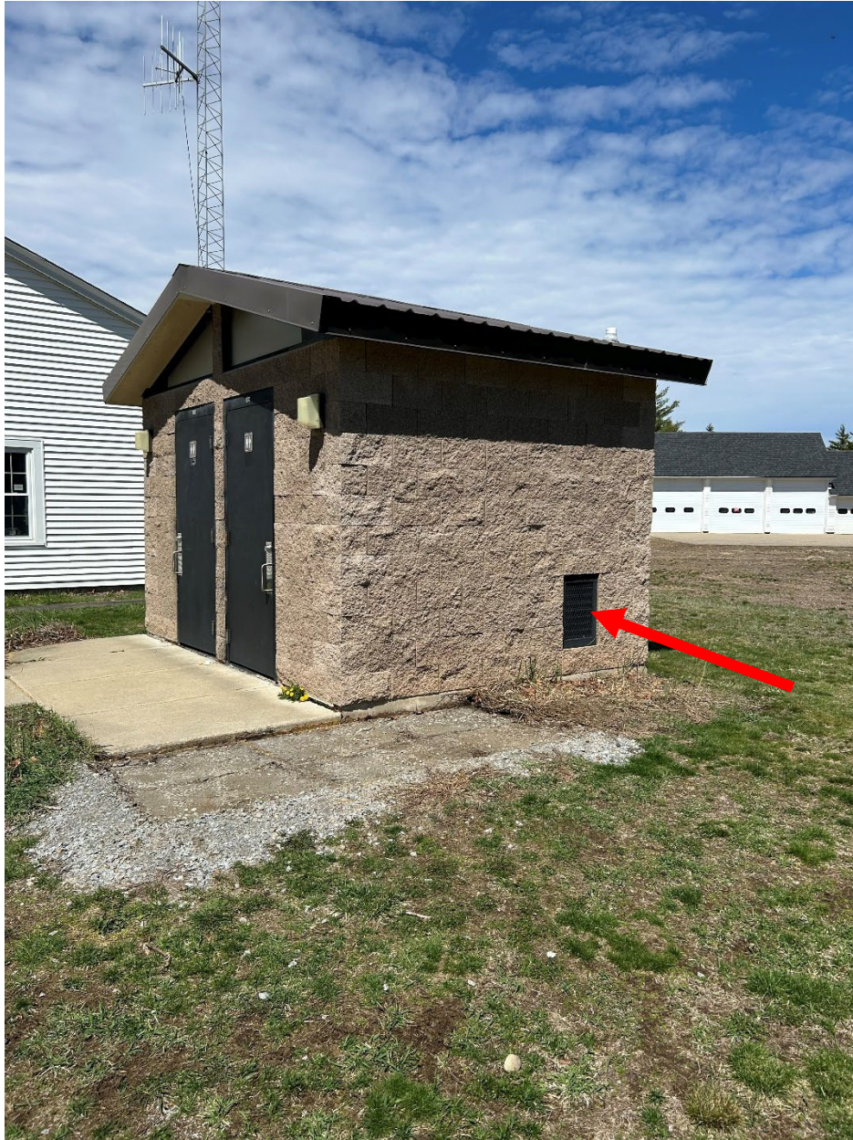
Informational Photo 2: East side of the restroom building with arrow pointing towards the vent that shall not be blocked. This is the side of building where the drinking fountain and walkway shall be installed.
