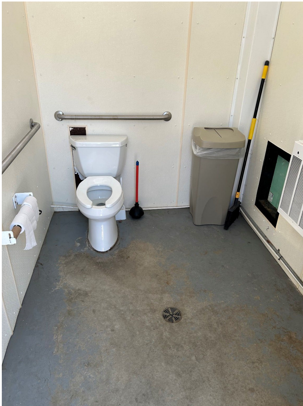
Informational Photo 5: Inside the Eastern restroom and facing the North side of the restroom. The existing water supply is the white pipe shown along the floor and extending through the wall behind the toilet.
