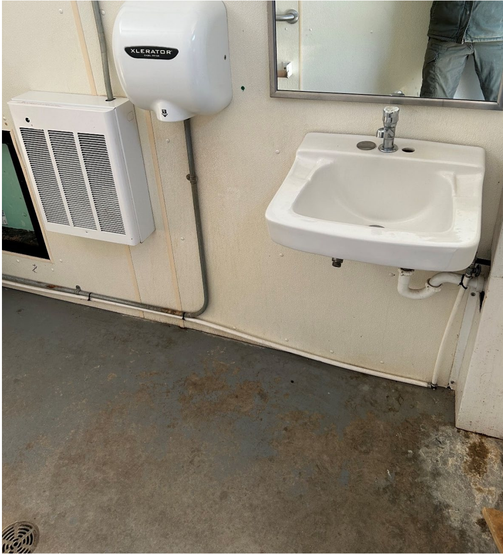
Informational Photo 4: Inside the Eastern restroom and facing the East side of the restroom. The existing water supply is the white pipe shown along the floor and terminating near the sink trap.
