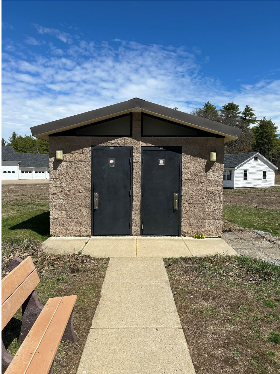
Informational Photo 1: Existing main approach walkway and front concrete apron with the two access doors to the restroom building facing North.
