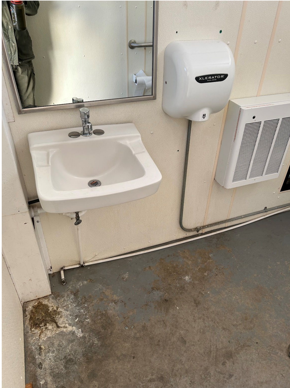
Informational Photo 7: Inside the Western restroom and facing the West side of the restroom. The existing water supply is the white pipe entering the building through the floor and is shown along the floor and running towards the North.
