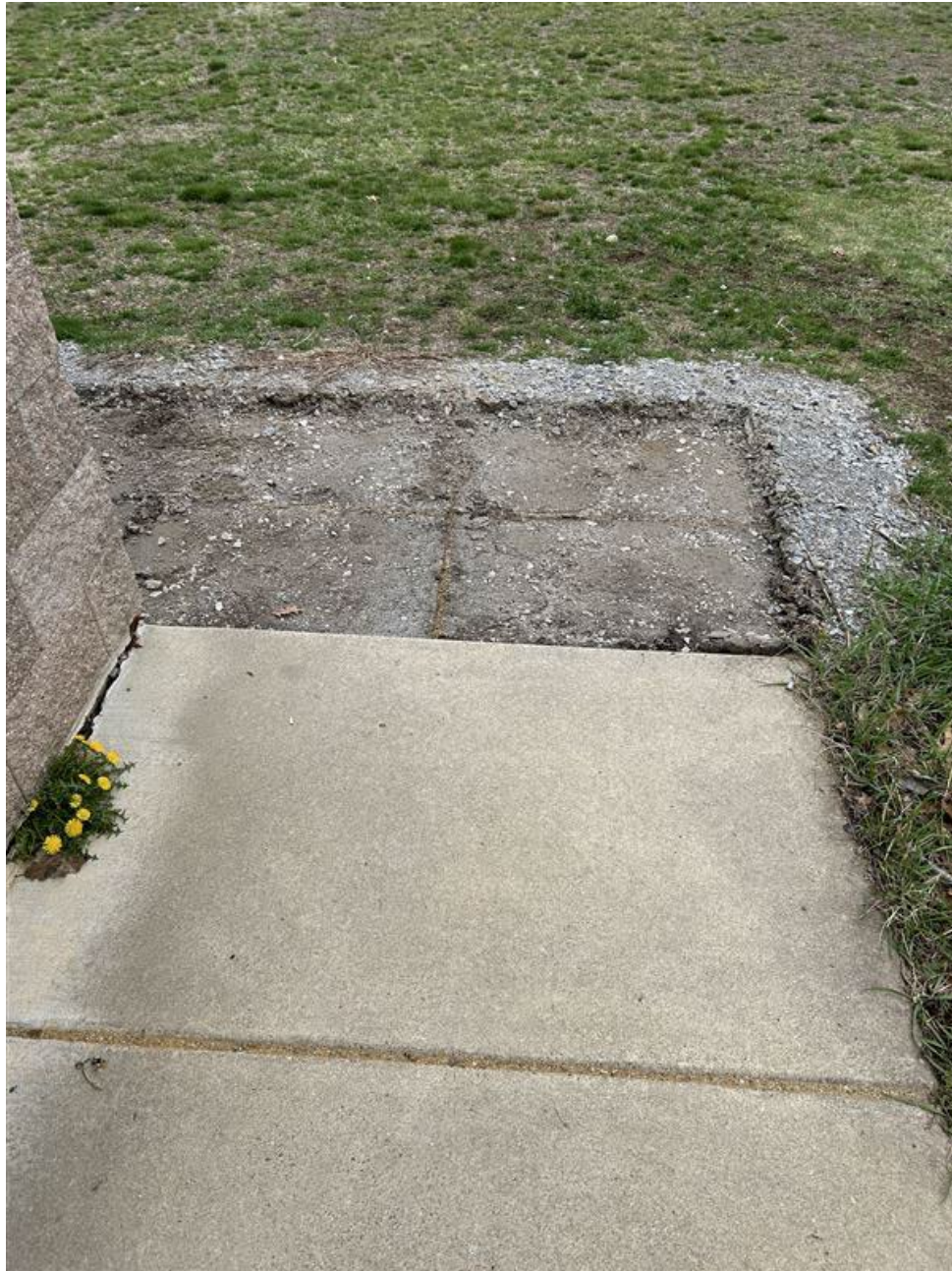
Informational Photo 3: Termination of the existing walkway facing towards the East side of the restroom building.
