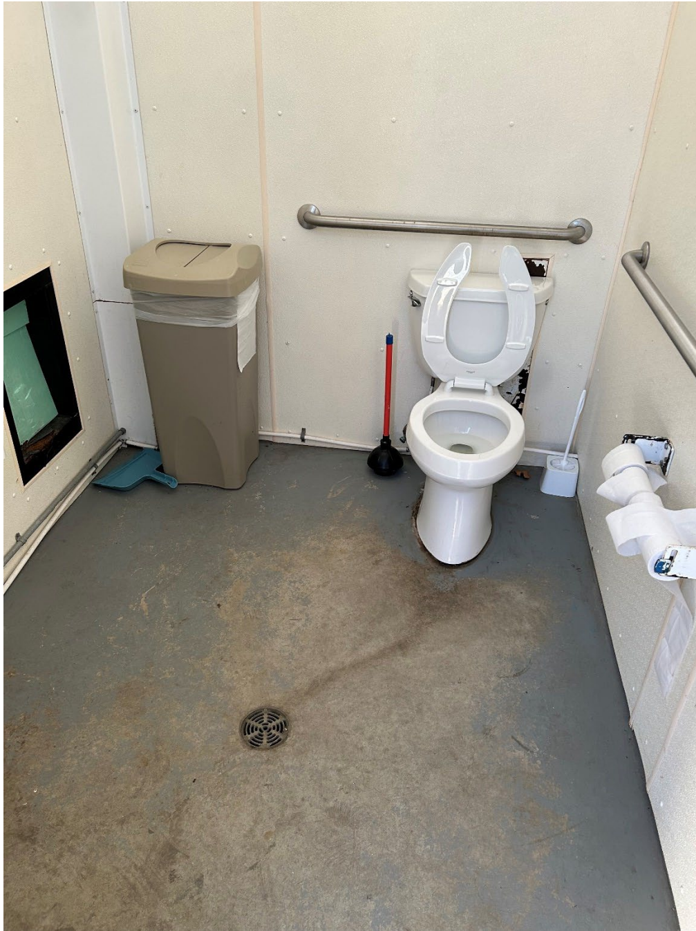
Informational Photo 6: Inside the Western restroom and facing the North side of the restroom. The existing water supply is the white pipe shown along the floor and extending from the right-side wall behind the toilet.
