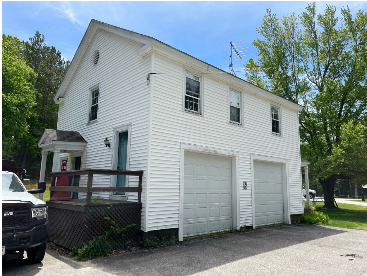
Informational Photo 1: Operator's Quarters Building showing personnel entry doors on the gable end of the building. The left door opens into the garage area; the right door opens to the stairwell to the second floor. Two large garage bay doors on the front of the building.
