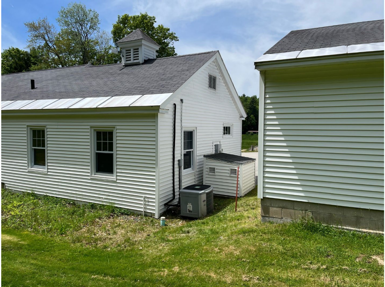
Informational Photo 15: Project Office Building (left building in the photo) showing the east facing gable end of the building with the air conditioning condenser and small utility shed.
