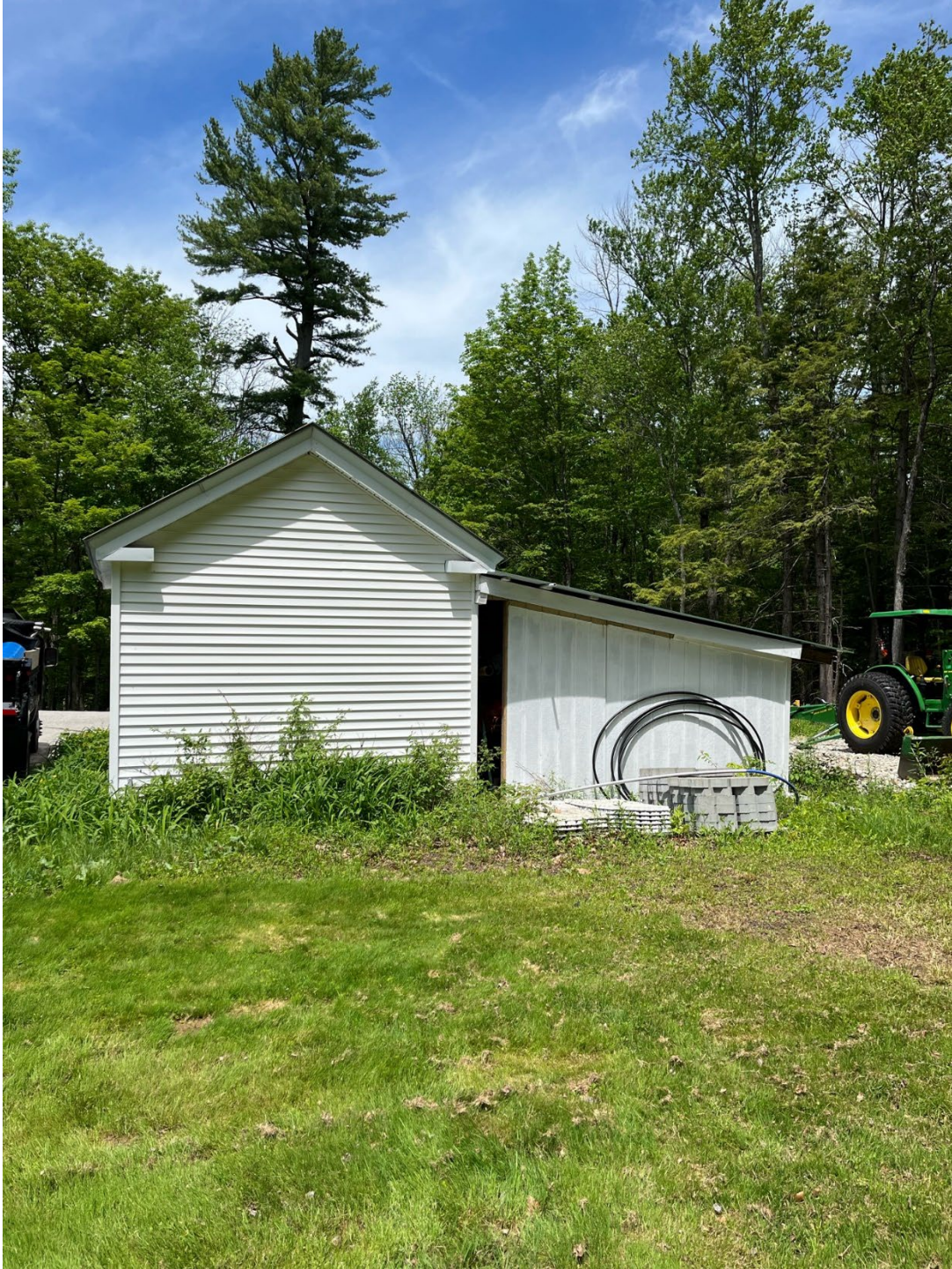
Informational Photo 29: Single Bay Garage Building showing the rear (south facing) side of the building with the attached lean-to type shed on the right side of the building.
