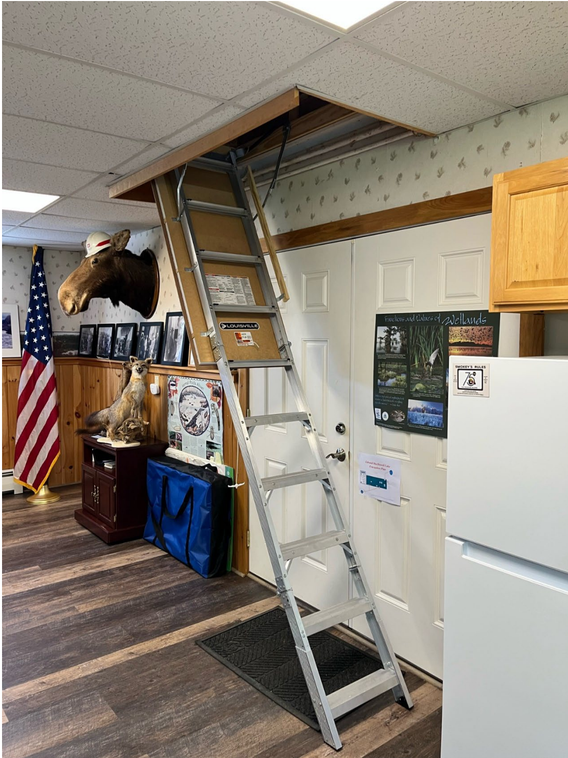
Informational Photo 24: Project Office Building showing the access door and ladder to the attic.
