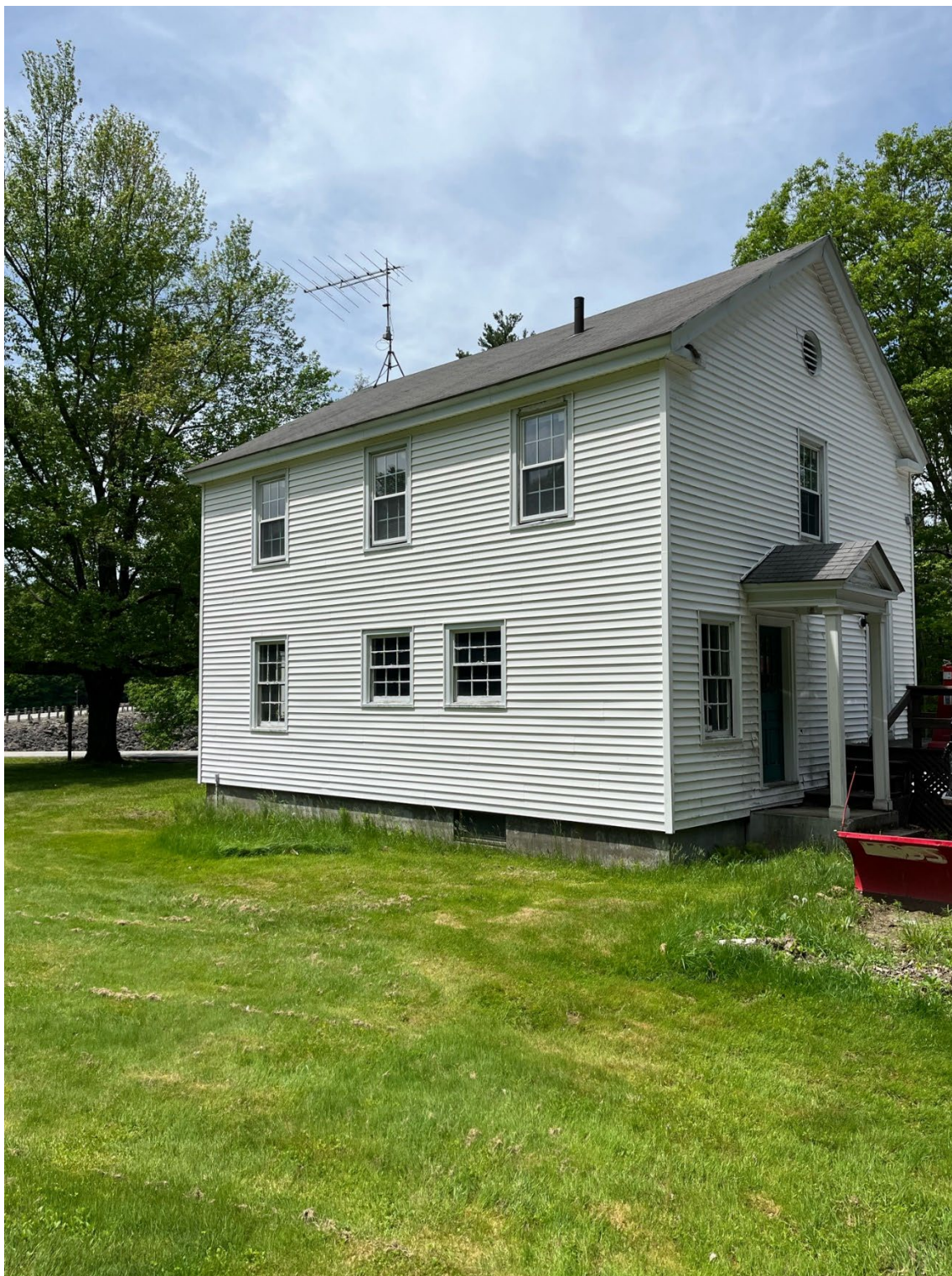
Informational Photo 2: Operator's Quarters Building showing personnel entry doors on the gable end and the rear side of the building.
