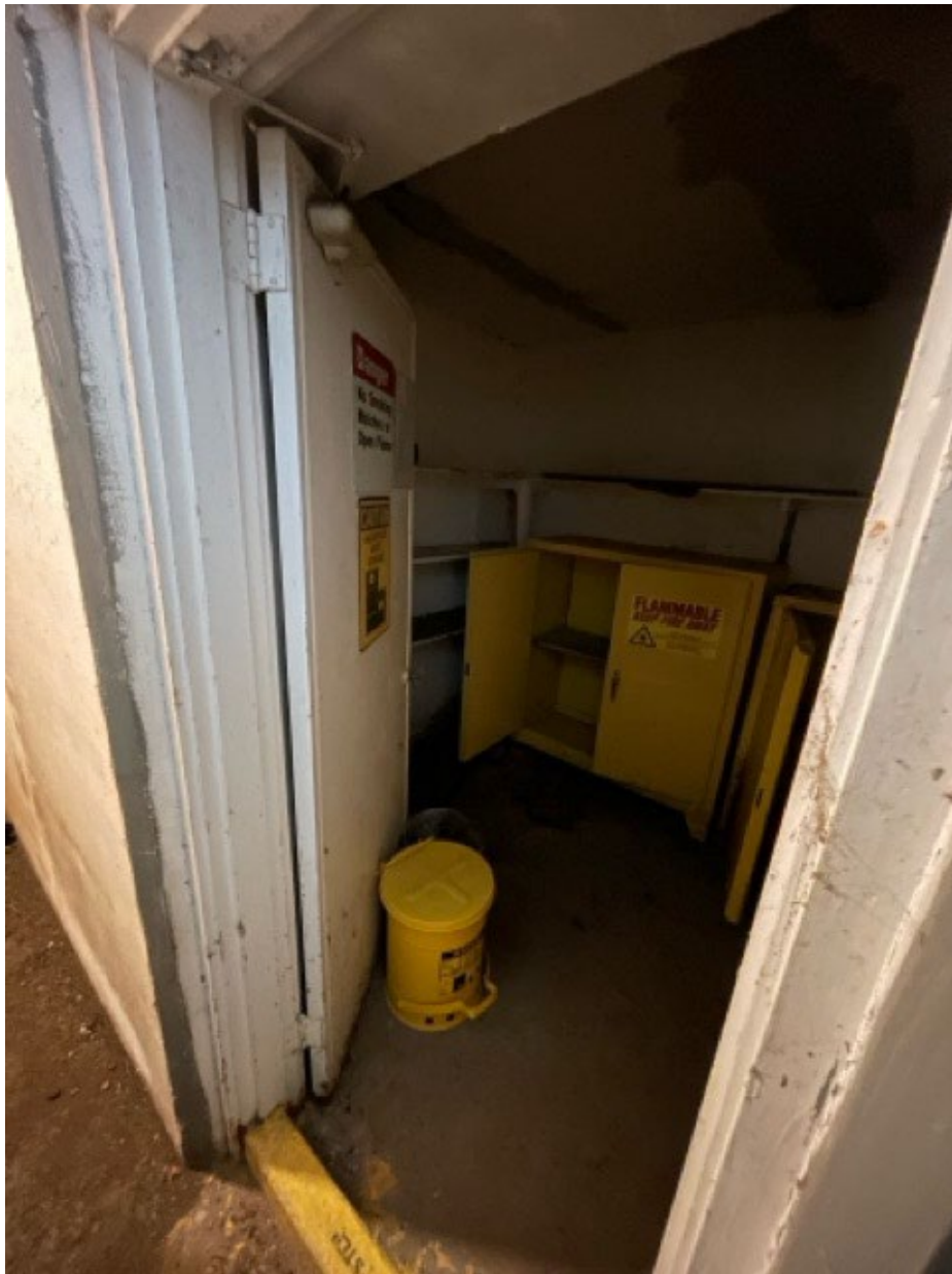
Informational Photo 7: Operator's Quarters Building showing the small cold storage room in the basement.
