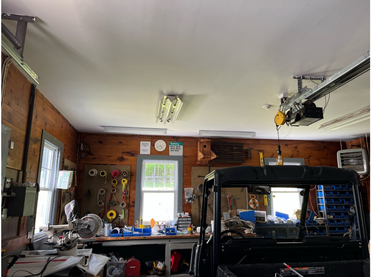
Informational Photo 27: Project Office Building showing the south wall of the garage opposite the overhead garage bay door.
