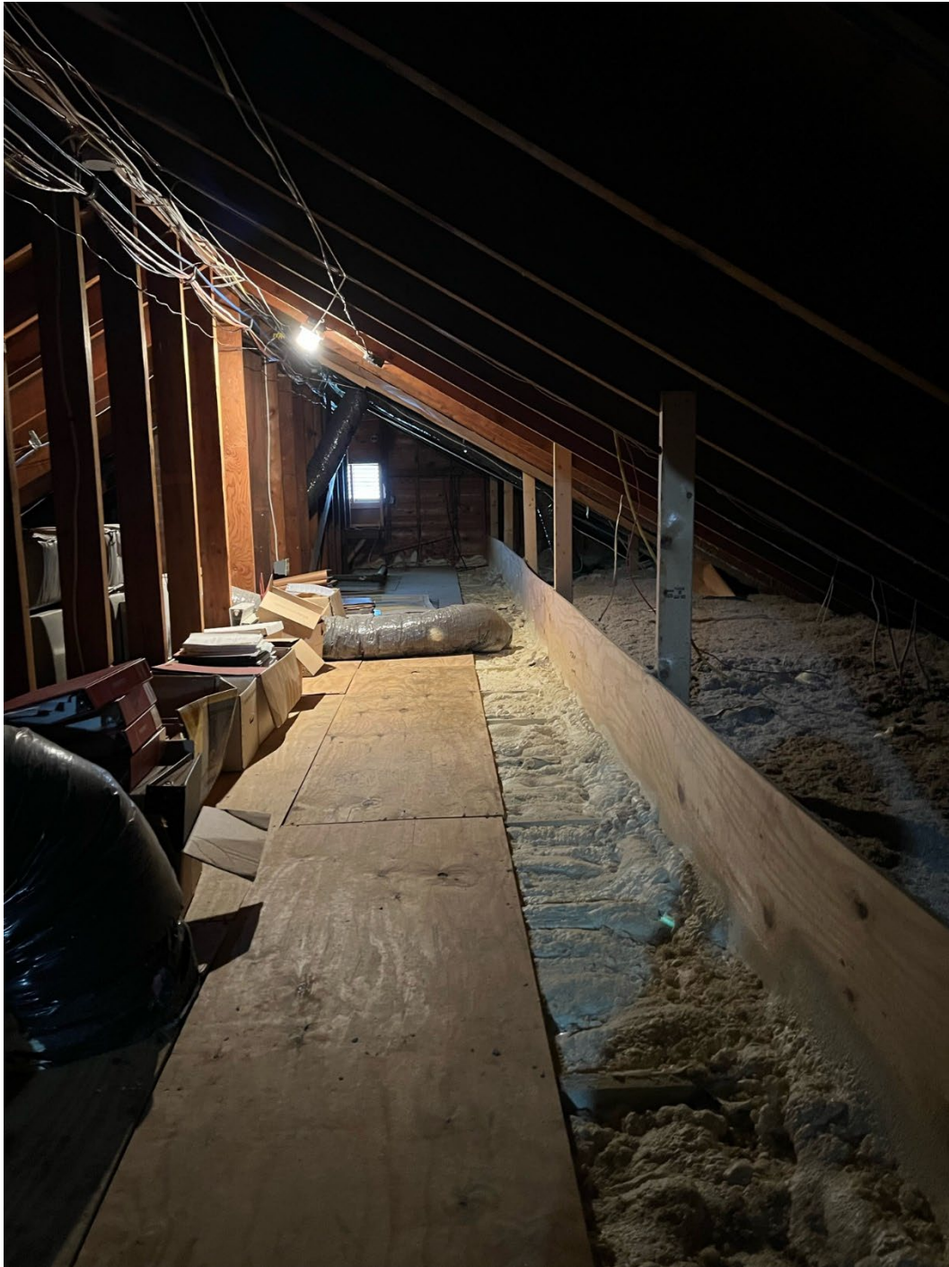
Informational Photo 25: Project Office Building showing the general condition of the attic space looking from the access ladder towards the West gable end of the building.
