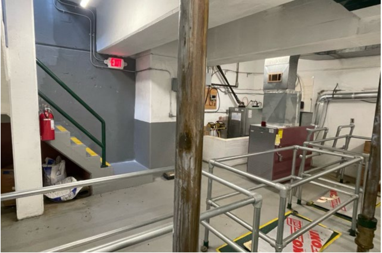
Informational Photo 38: Gatehouse Building showing the Heater Room Floor level looking at the stairs.
