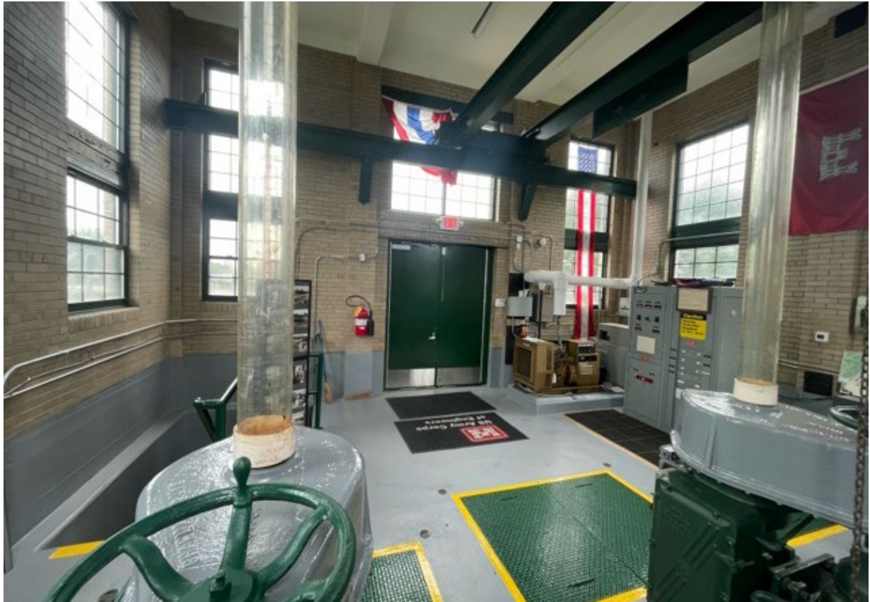
Informational Photo 32: Gatehouse Building showing the Operating Floor level looking back at the entry doors.
