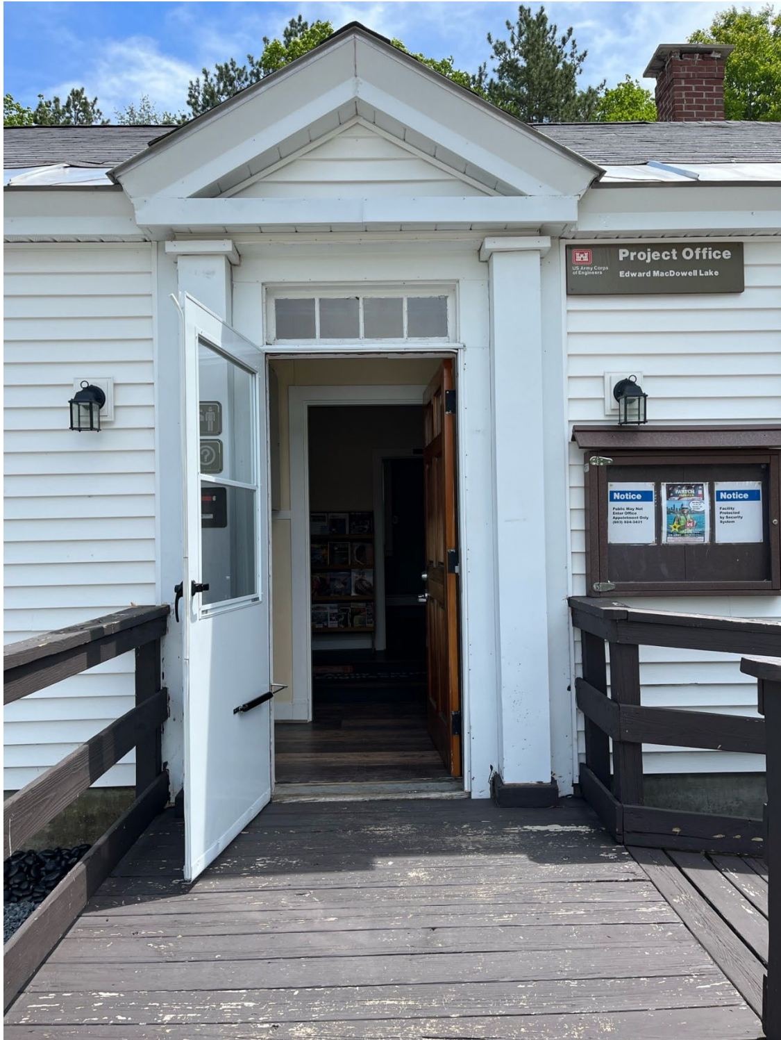
Informational Photo 16: Project Office Building showing the original 4 lite grid window above the entry door.
