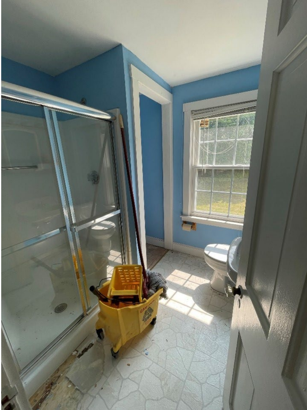
Informational Photo 9: Operator's Quarters Building showing second floor bathroom.
