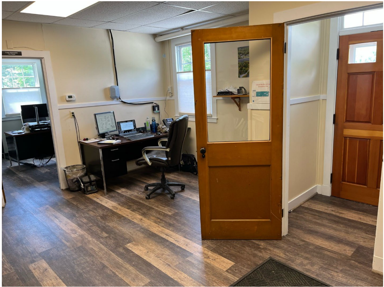
Informational Photo 17: Project Office Building showing the entry way, an office space, a hung ceiling, and an insulated water pipe.
