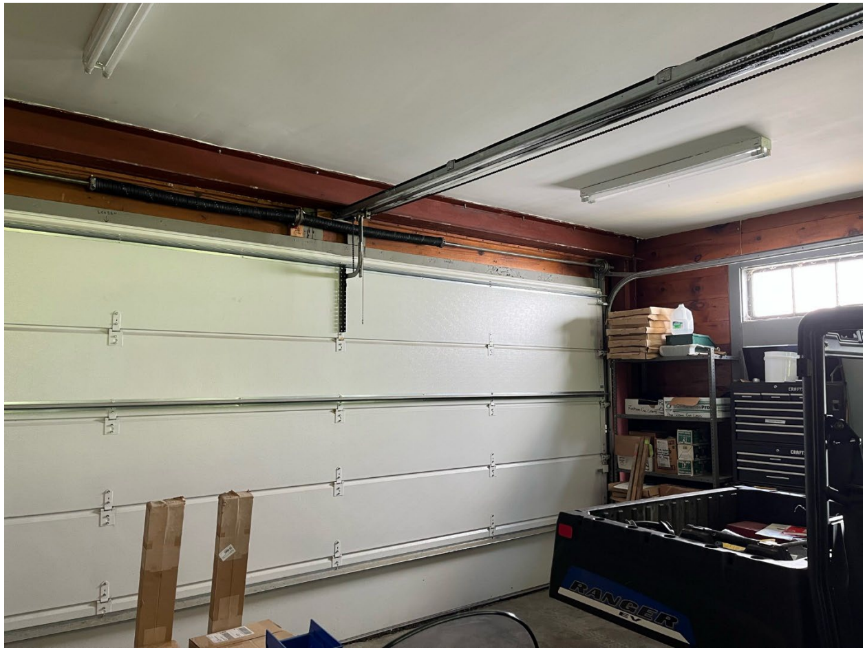
Informational Photo 26: Project Office Building showing the single overhead garage bay door, the reinforcing steel beam above the door, and an original 4 lite grid window on the right side of the photo.
