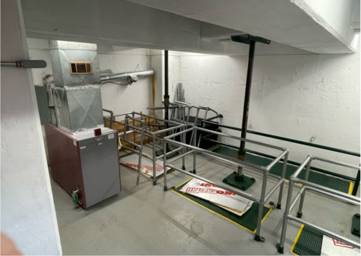
Informational Photo 37: Gatehouse Building showing the Heater Room Floor level from the stairs.
