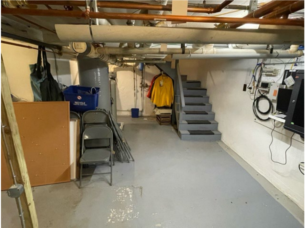
Informational Photo 21: Project Office Building showing the basement looking towards the stairs to the main floor.
