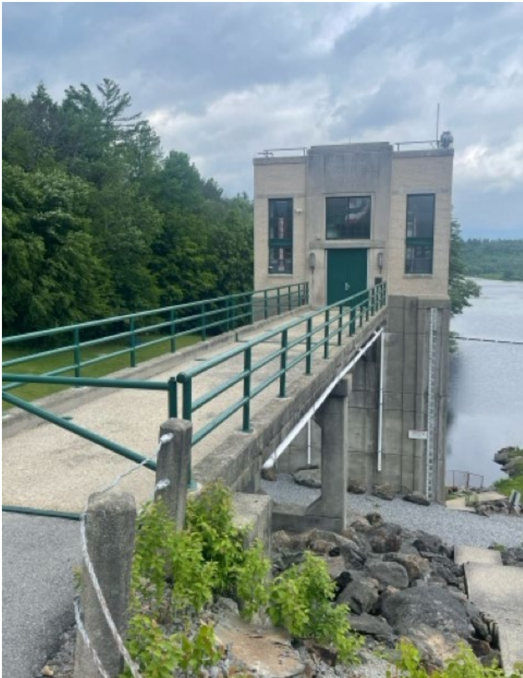
Informational Photo 30: Gatehouse Building showing the service bridge to the entry doors of the Operating Floor level.
