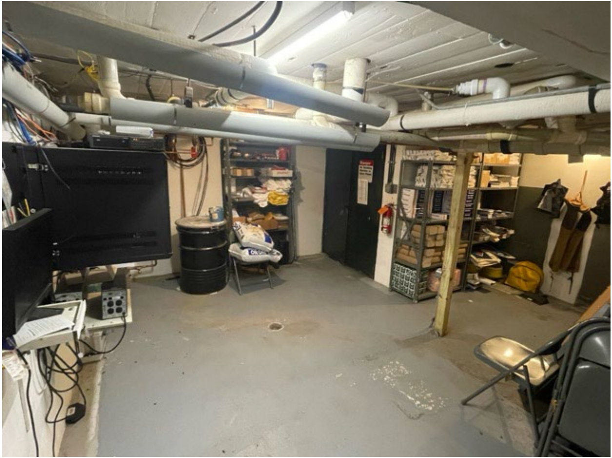
Informational Photo 20: Project Office Building showing the basement area from the landing of the stairs perspective.
