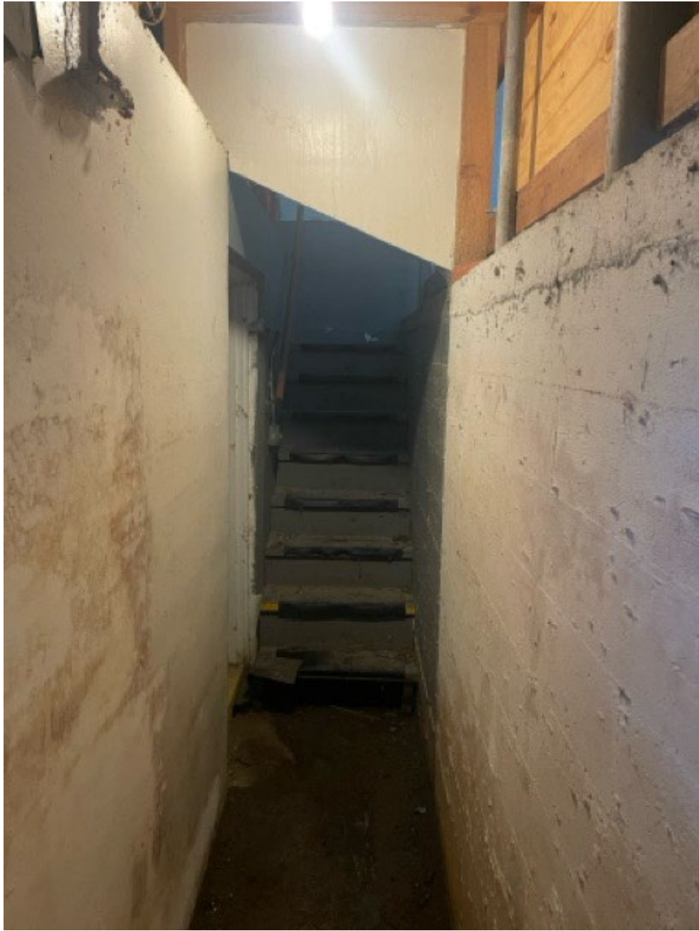
Informational Photo 5: Operator's Quarters Building showing the stairway in the basement hallway that leads to the garage level of the Operator's Quarters building.
