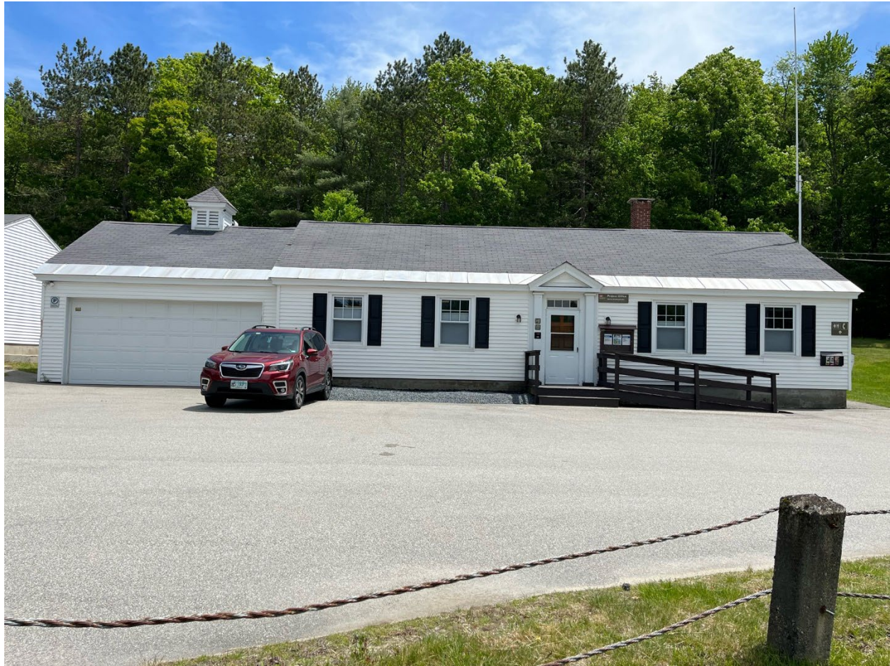
Informational Photo 12: Project Office Building showing the main (front) entry door and attached garage.
