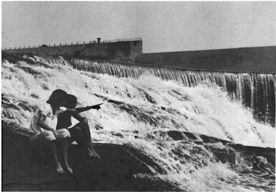
Downstream from Mansfield Hollow Dam
