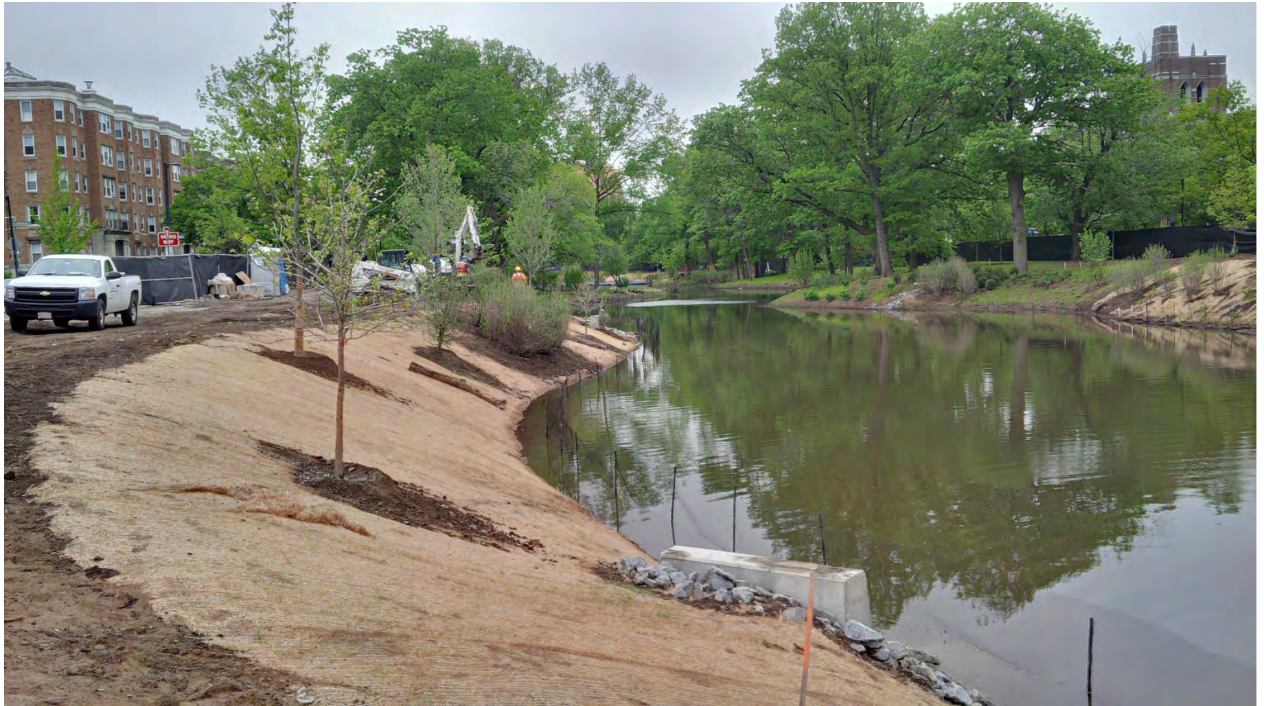
Former Jug Handle Roadway – area completely daylighted and river diversion sheeting extracted. Note the beginning of plantings on the left bank, looking downstream – late May 2016.
