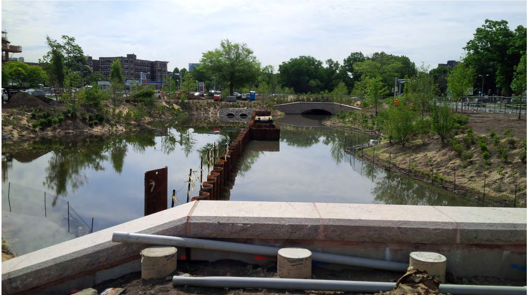
Former Sears Parking Lot – looking downstream at the new Brookline Avenue Culvert – filling of the left side (looking downstream) of the FRM channel is complete, awaiting the extraction of the river diversion sheeting. Note that both banks have been planted; and plantings will continue. Note also the footings for the permanent steel handrail at the culvert headwall – mid June 2016.
