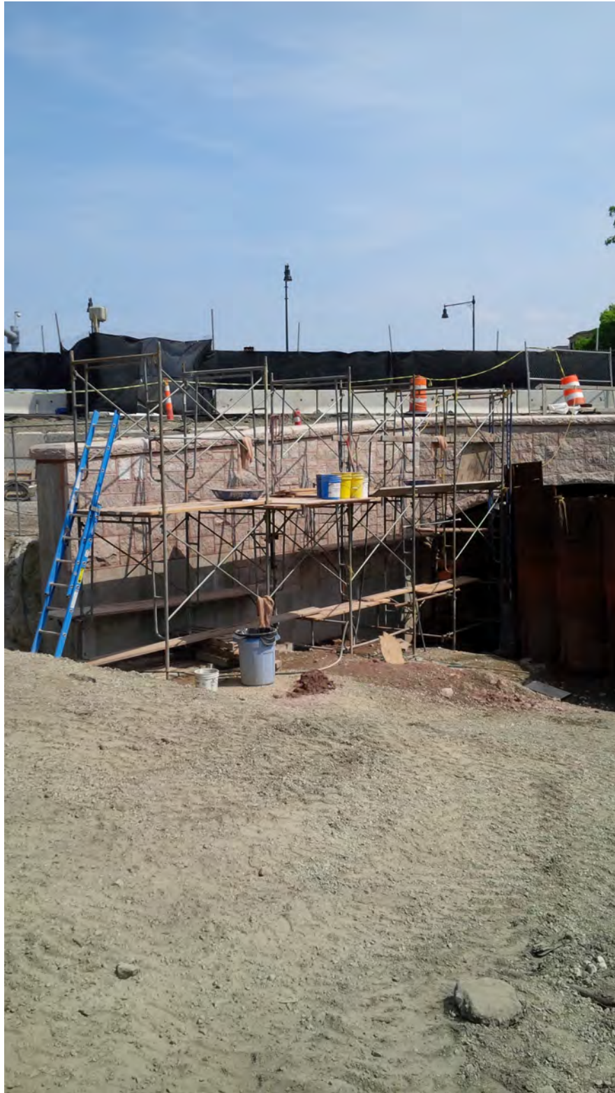
Upstream Riverway Culvert – Installing granite veneer on the northwest wing wall – late May 2016.
