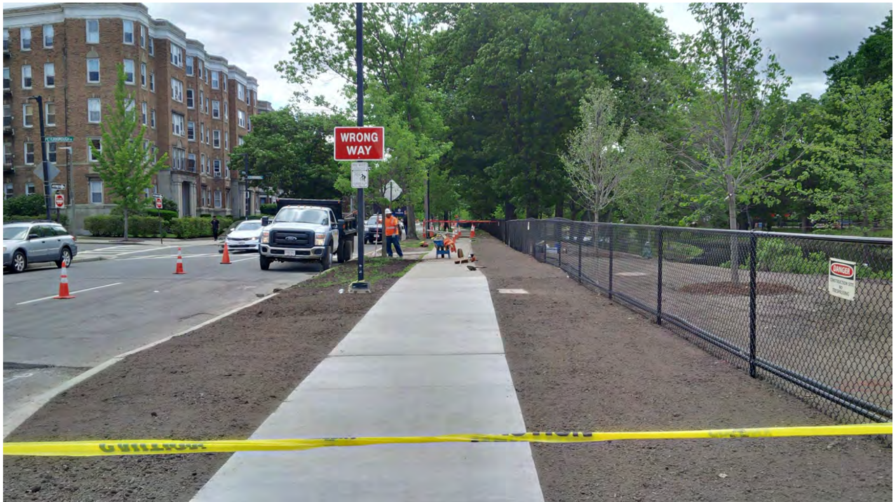
Construction of the end condition concrete sidewalk on Park Drive, in the vicinity of the former Jug Handle Roadway. Note the new loam on impacted landscaped areas, ready for hydroseed; and the installed temporary landscape protection fencing – early June 2016.
