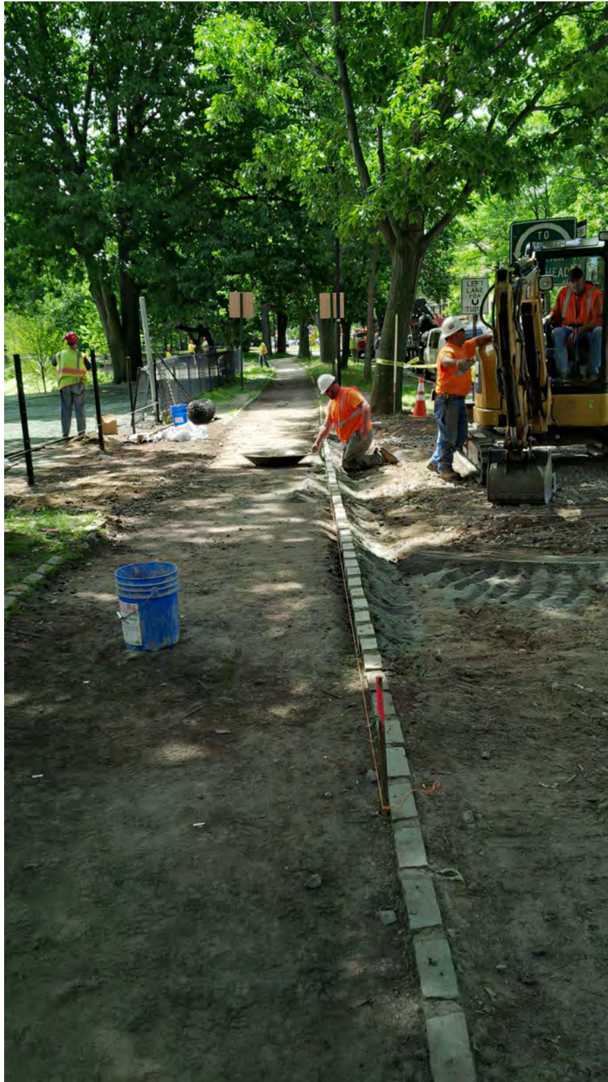
Reconstruction of impacted area – resetting the granite blocks delineating the stone dust pathway along the Fenway roadway. Note the installation of the temporary landscape protection fencing in the location of the construction access gate, which will no longer be used – mid-June 2016.
