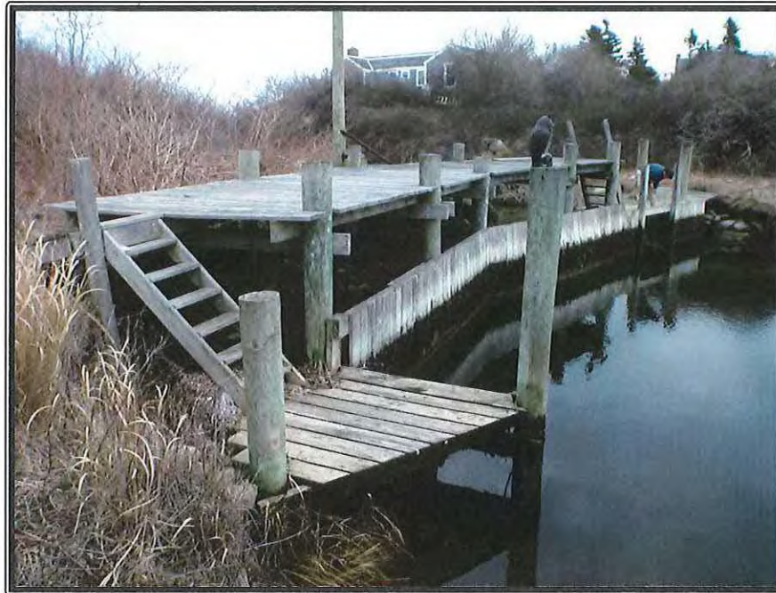
Photograph No.: 4 View to the east of the pile-supported wooden pier structure.
