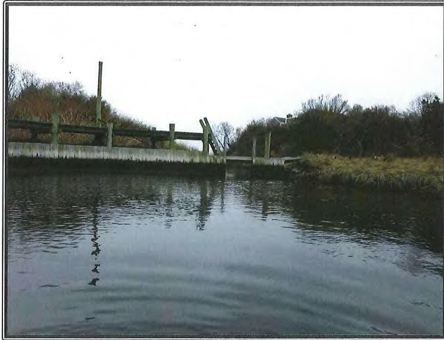
Photograph No.: 3 View to the northeast of the pile-supported wooden pier structure.
