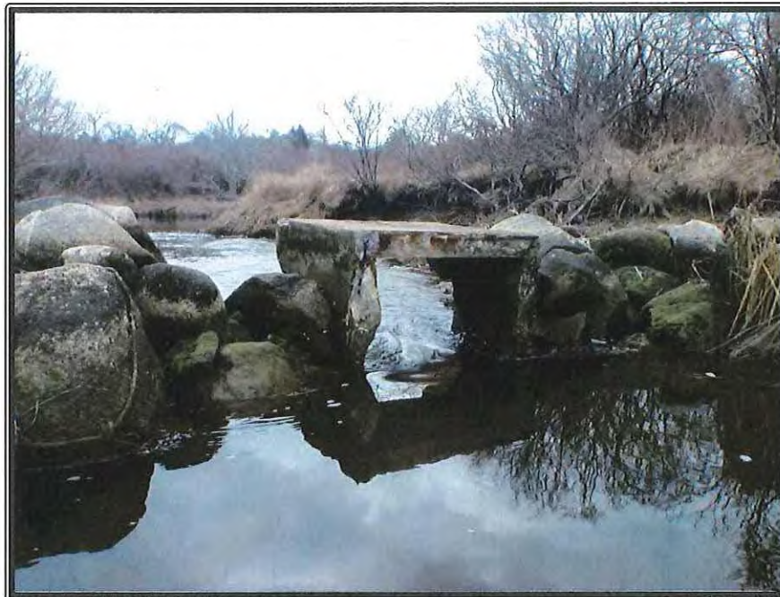
Photograph No.: 6 View to the southeast of the concrete box culvert.
