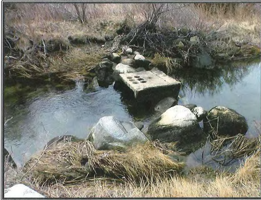
Photograph No.: 5 View to the southwest of the concrete box culvert.
