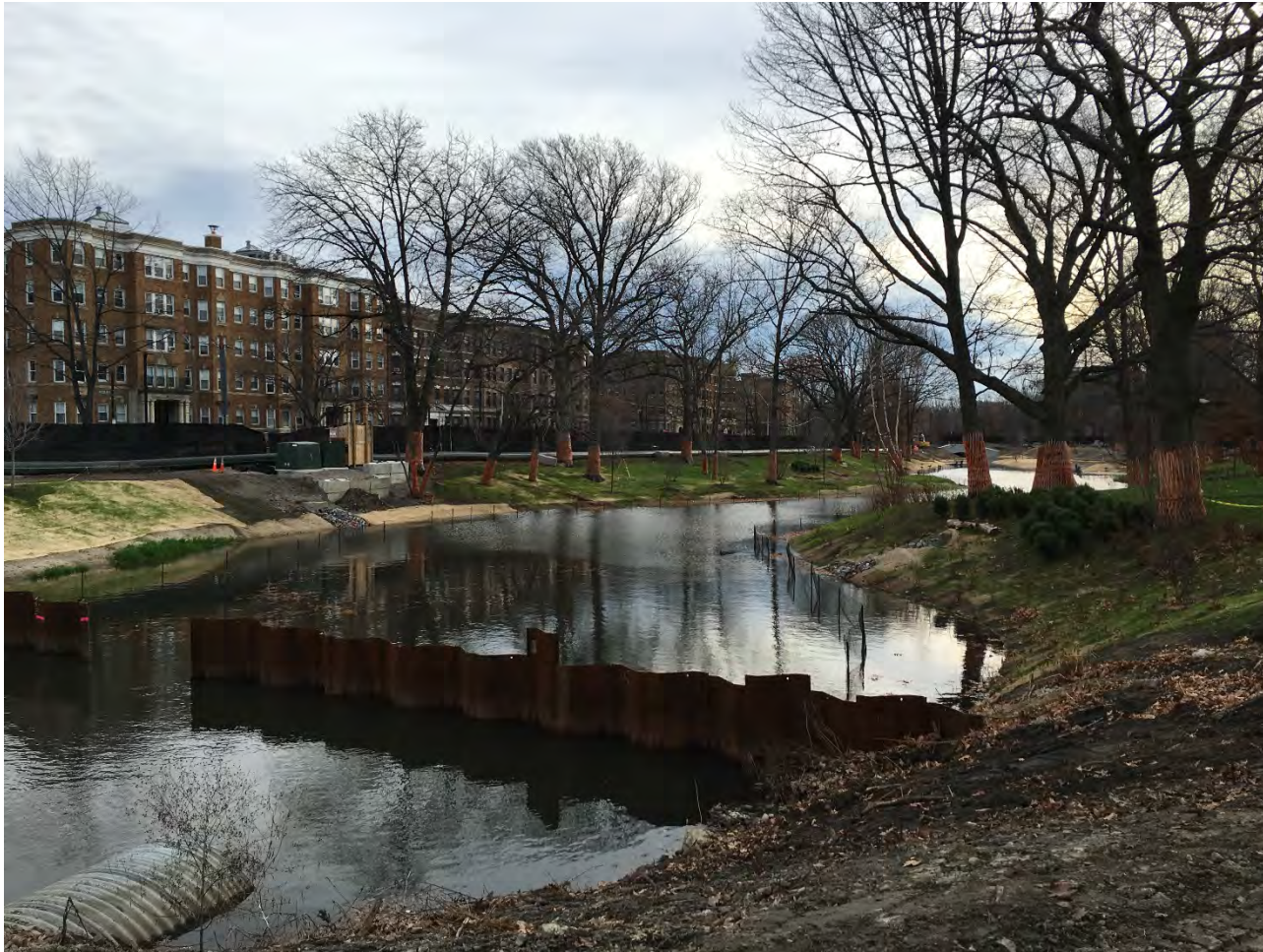
Water flowing over the steel sheeting cofferdam at Upper Fens Pond after the pumps were turned off – note the notch that was cut in the sheeting to allow water to flow slowly back into the pond – looking downstream towards Ave Louis Pasteur – 21 December 2015.
