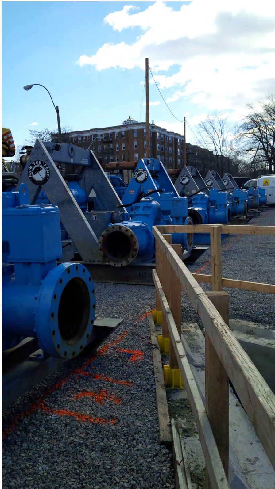
Six pumps in place for the river diversion of the Upper Fens Pond.
