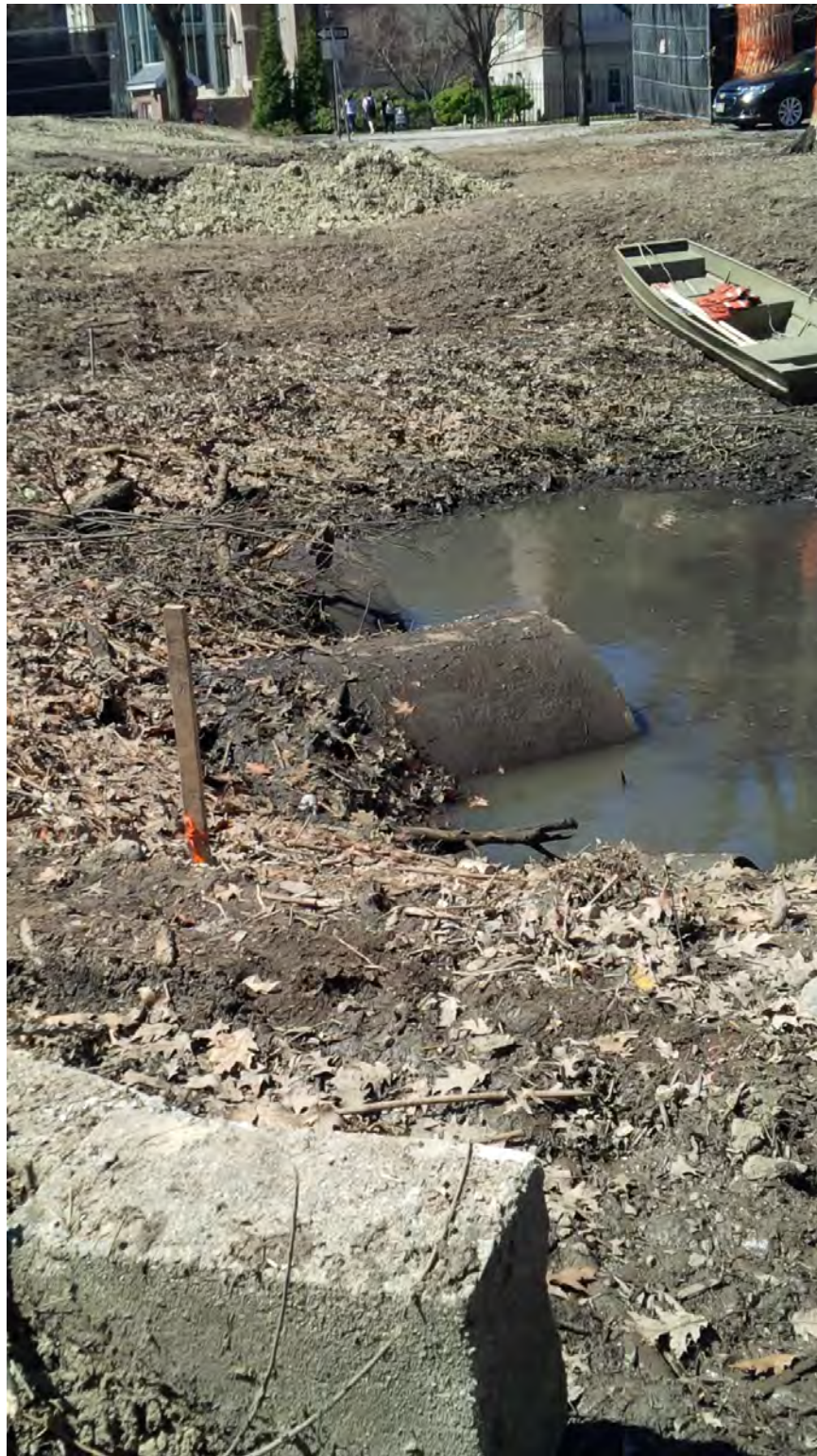
Top of the existing twin 72" culverts between the Upper Fens Pond and Avenue Louis Pasteur appear as the work area is dewatered and river flow is diverted – mid-April 2015.
