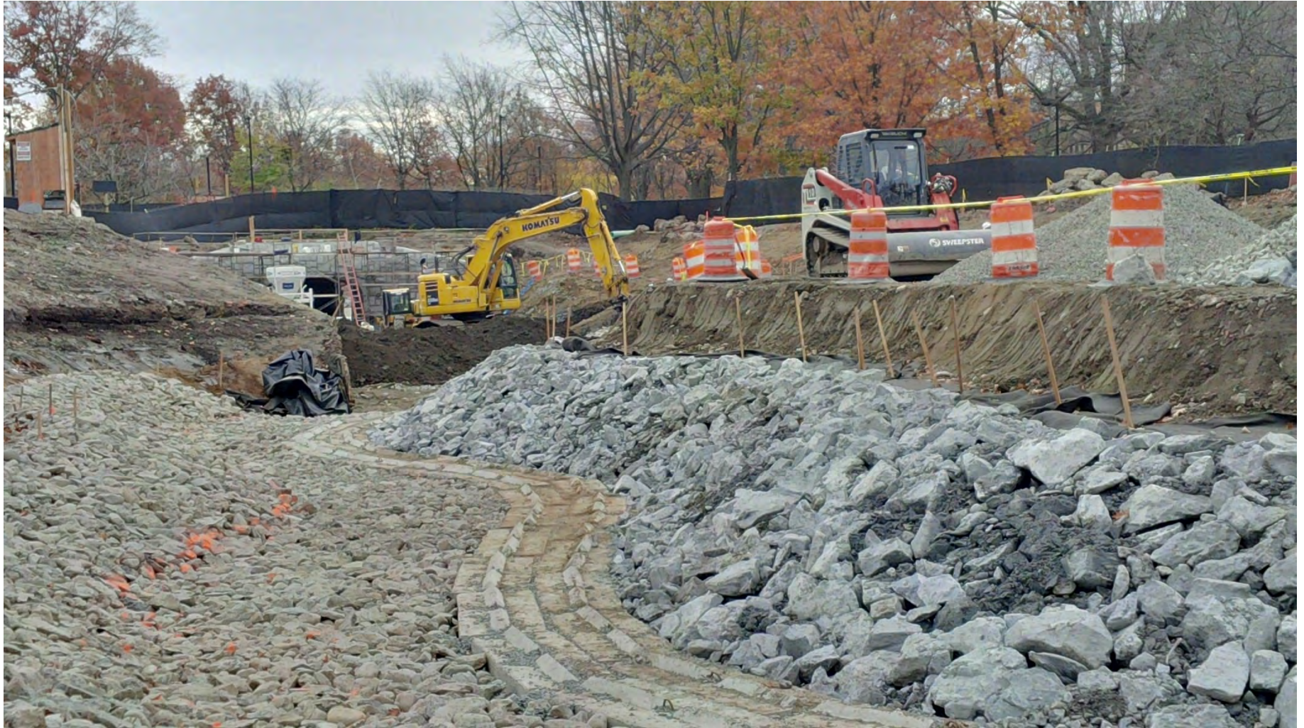
Daylighting of area between Upper Fens Pond and Avenue Louis Pasteur Culvert – note the recreation of the historic Olmstead island (foreground right) starting to take shape – early November 2015
