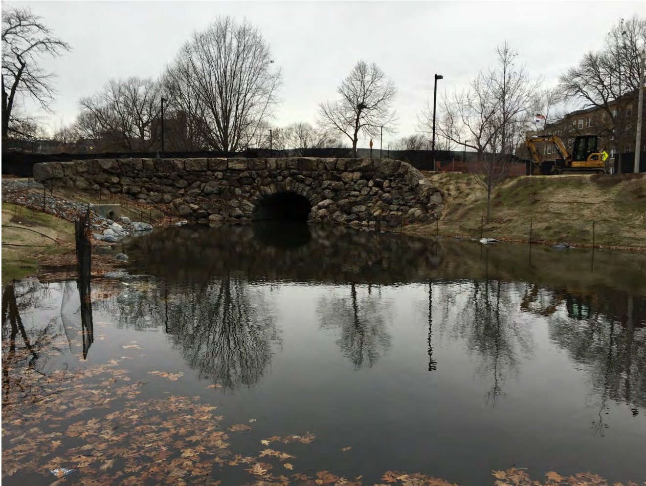
Water flowing downstream of Avenue Louis Pasteur culvert – 21 December 2015.
