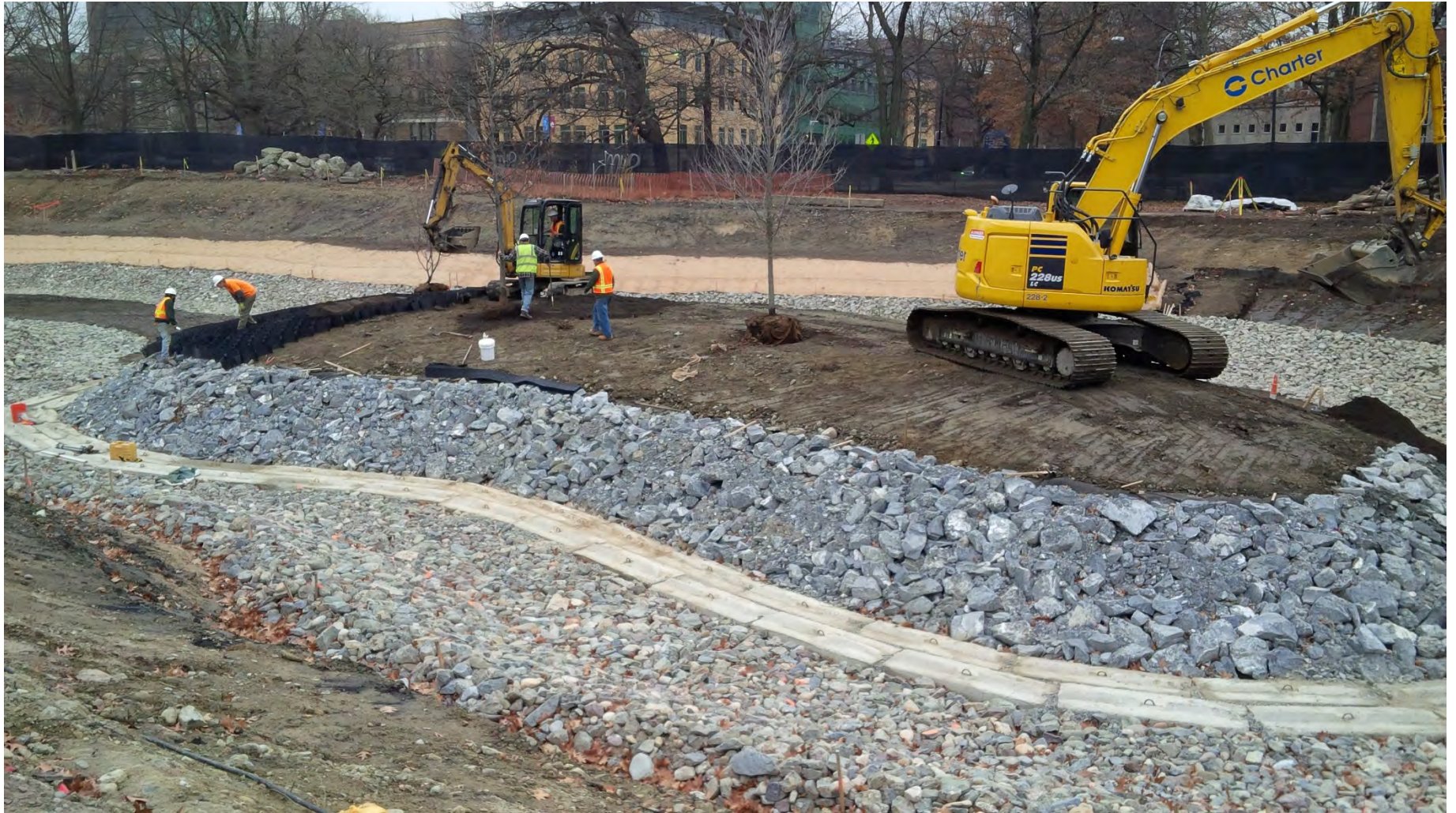
Installation of the geocells and loam and planting of the historic Olmsted Island – early December 2015.
