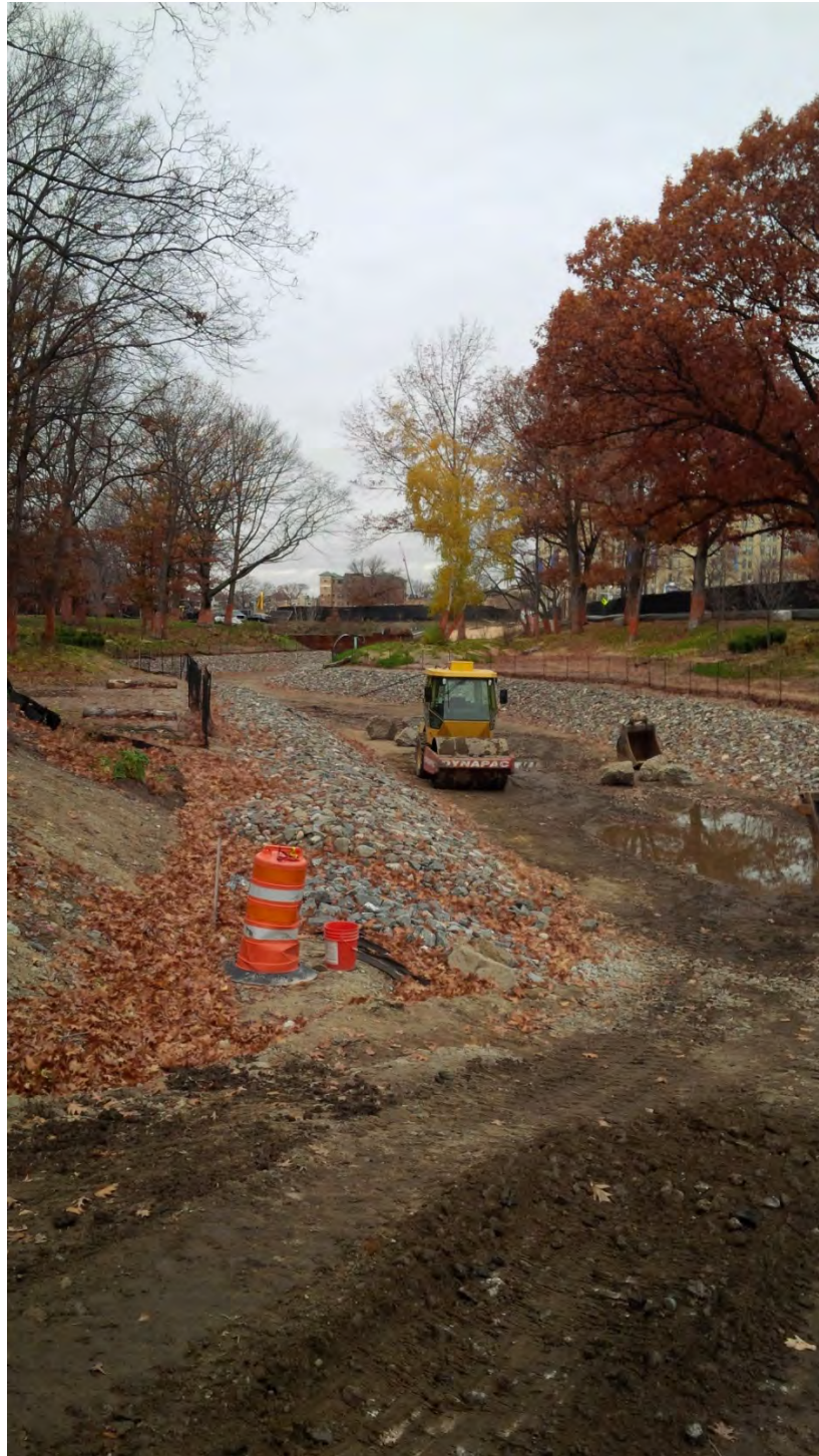
Upper Fens Pond – plantings as part of the bank restoration work in the fall planting season completed – herbivore exclusion fence and habitat boulders installed – early November 2015.
