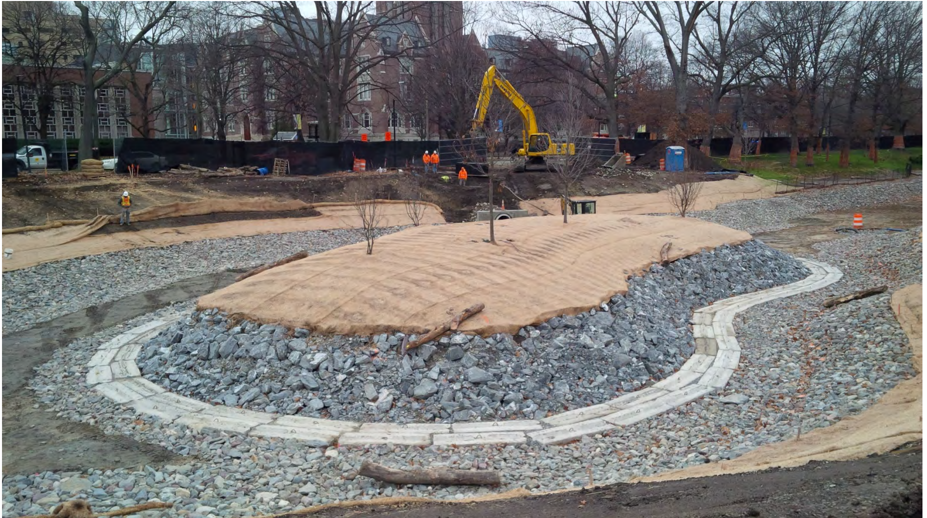
Recreated historic Olmsted Island – with new geocells, loam, and turf reinforcement mattress (TRM) installed and all trees planted – note the habitat logs installed on the island and in the constructed channel – looking cross river towards Simmons College – mid December 2015.
