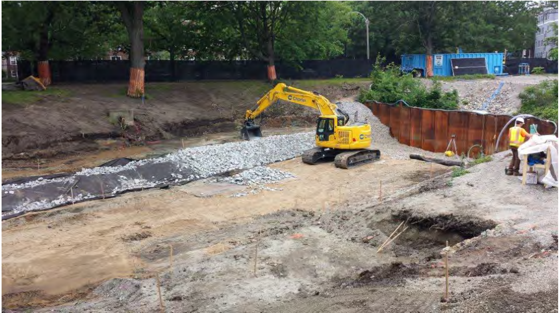
Bank stabilization/construction with stone protection at Upper Fens Pond – early June 2015.
