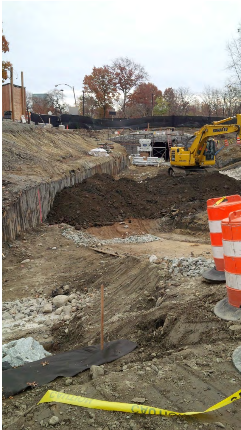
Excavation of the area between Upper Fens Pond and Avenue Louis Pasteur Culvert – note the existing timber piling on the left side which delineates the side of the existing twin 72” culverts that were recently removed as part of the daylighting efforts – early November 2015.
