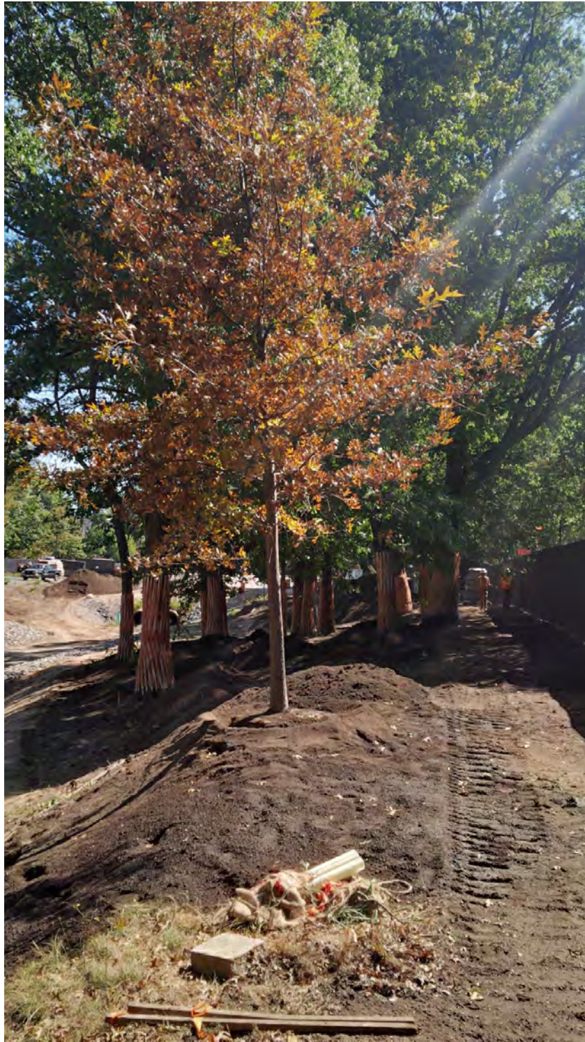
Upper Fens Pond – new tree being planted as part of the bank restoration work – late September 2015.
