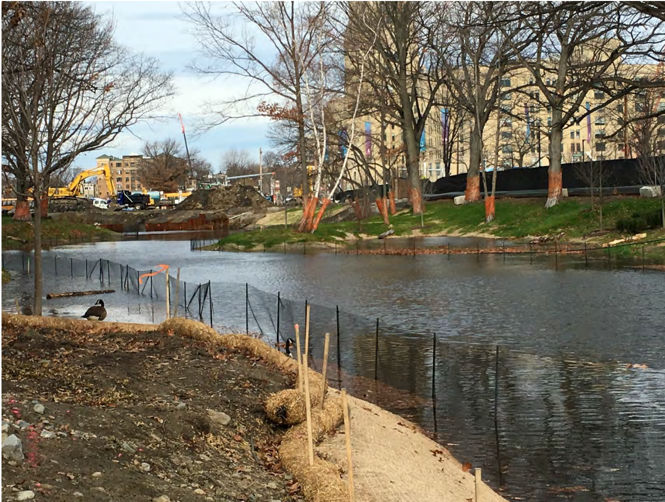
Water flowing in Upper Fens Pond after the pumps were turned off – looking upstream towards Landmark Center – 21 December 2015.
