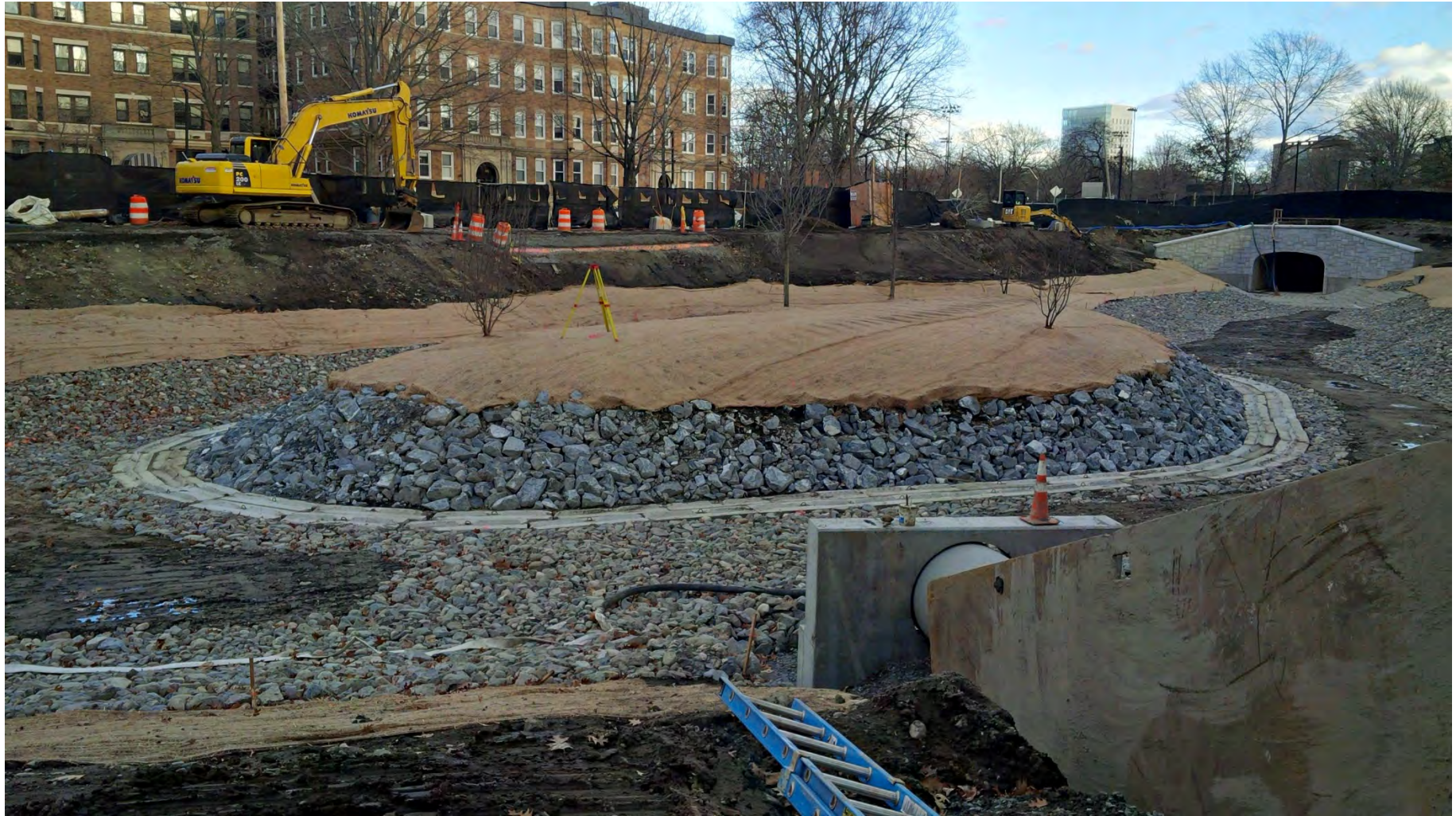
Recreated historic Olmsted Island – with new geocells, loam, and turf reinforcement mattress (TRM) installed and all trees planted – note in the foreground a new headwall and drainage piping being installed on the constructed right bank of the daylighted area – looking downstream at the Avenue Louis Pasteur culvert – mid December 2015.
