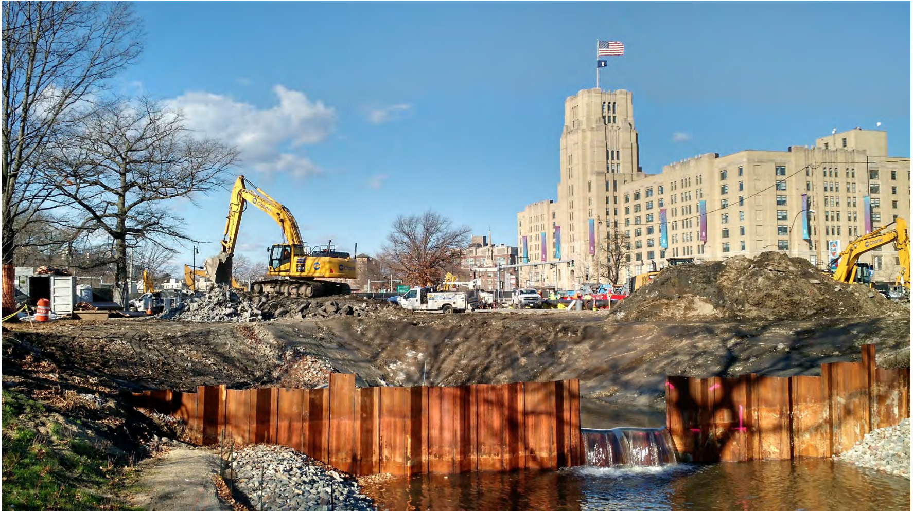
Water flowing over the steel sheeting cofferdam at Upper Fens Pond after the pumps were turned off – note the notch that was cut in the sheeting to allow water to flow slowly back into the pond – looking upstream towards Landmark Center – 19 December 2015.
