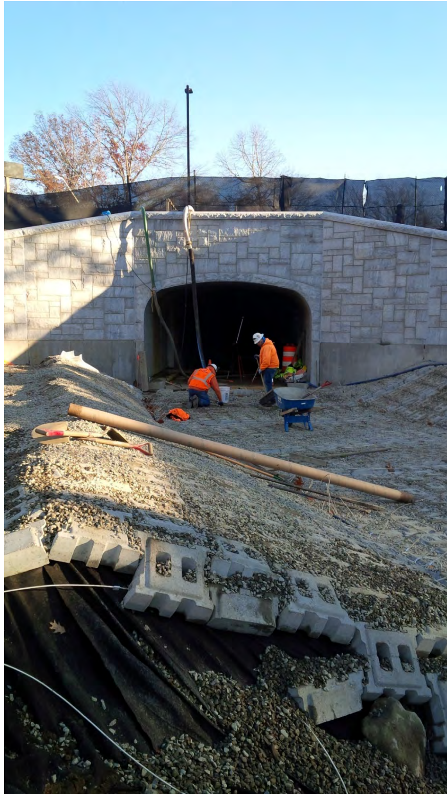
Installation of the articulated concrete blocks (ACBs) at the upstream end of the Avenue Louis Pasteur culvert – early December 2015.
