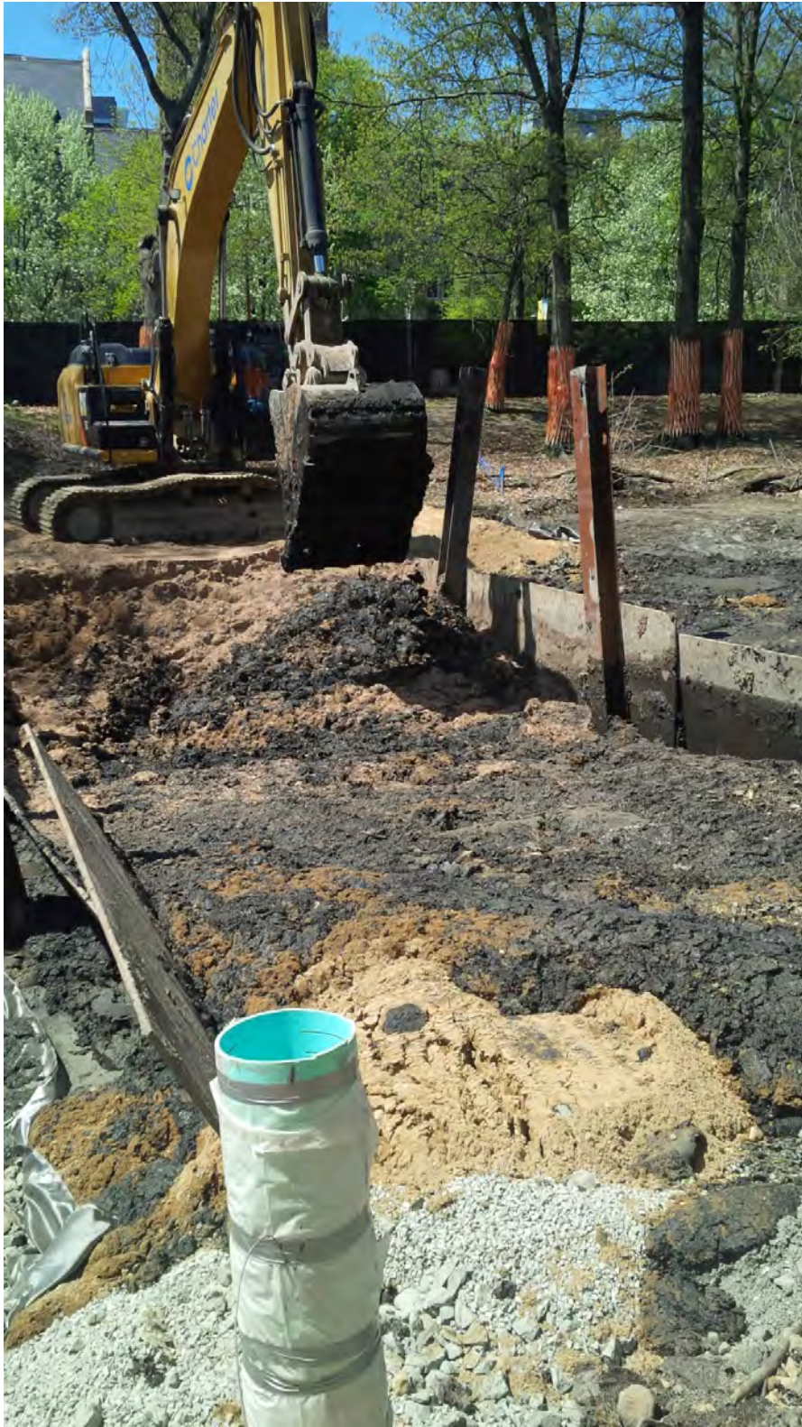
Excavator mixing saw dust into the river sediment to help solidify the material for transport off-site.
