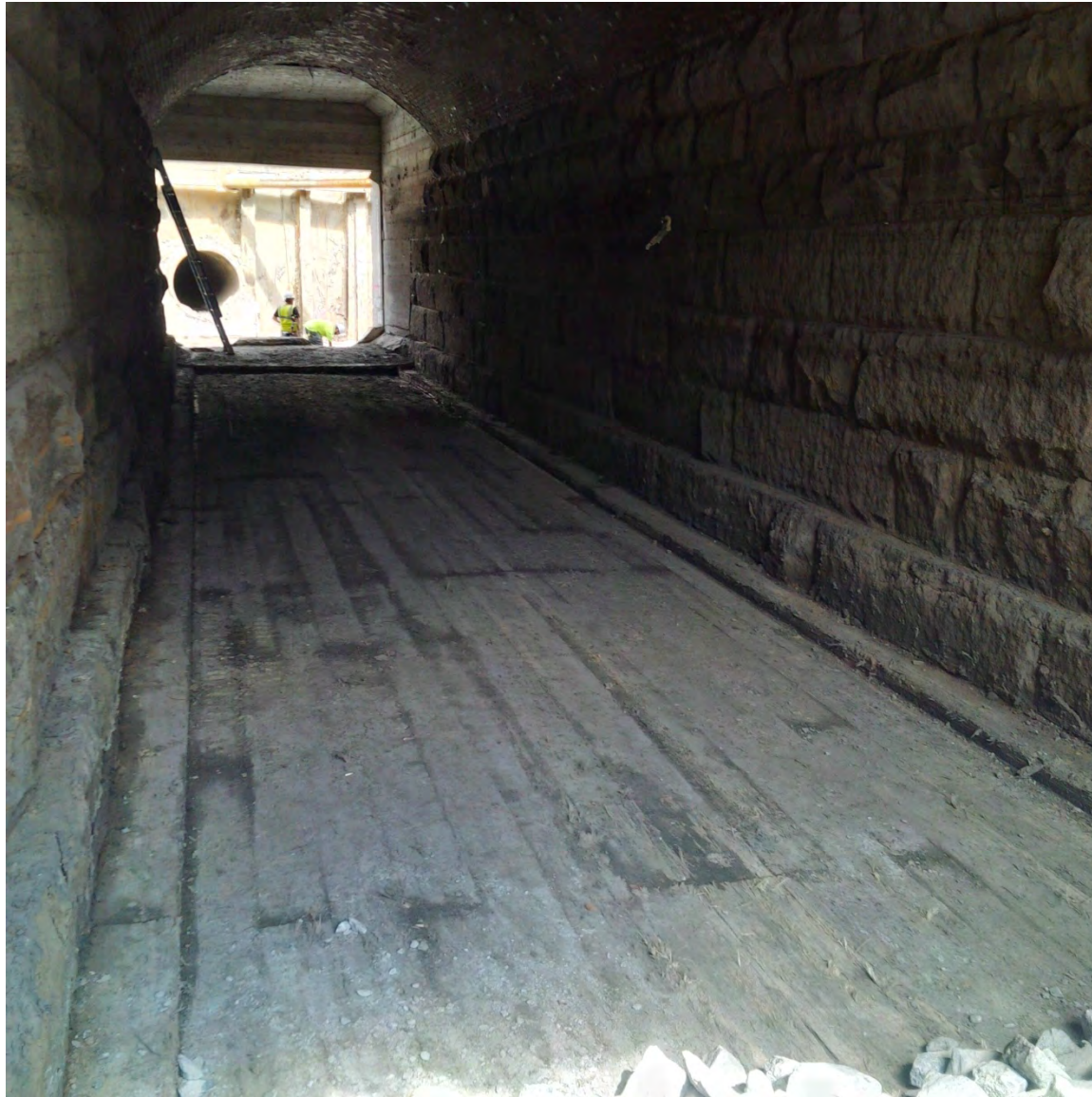
Completed sediment removal from inside the existing Avenue Louis Pasteur culvert revealed an existing timber flooring – late August 2015.
