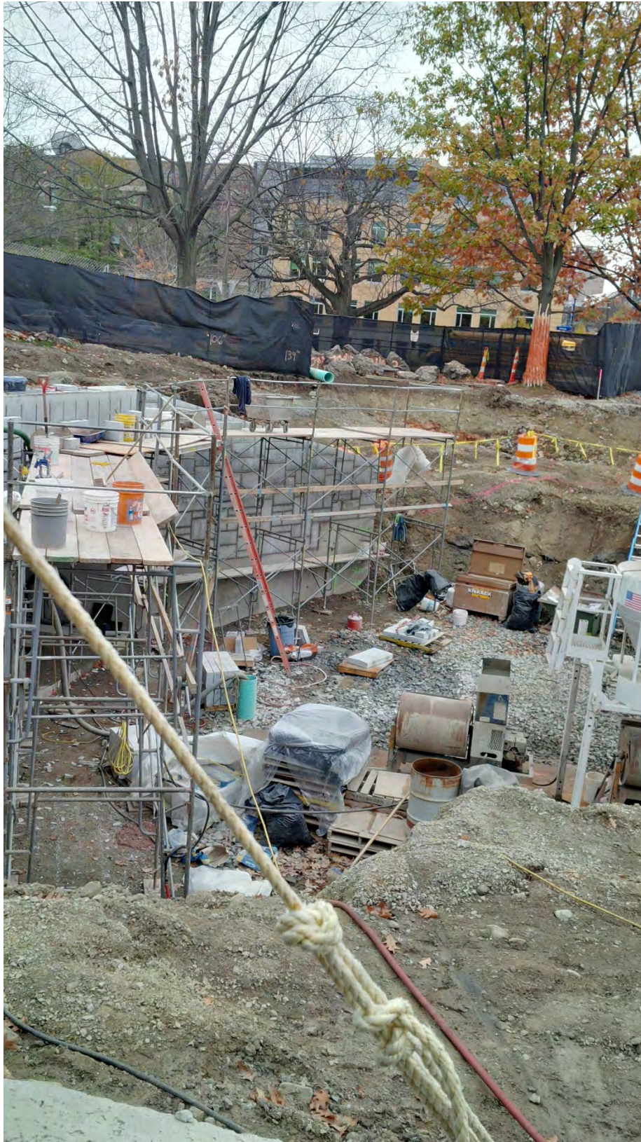
New granite veneer being installed on the façade of the new precast concrete culvert sections and new wingwalls of the Avenue Louis Pasteur Culvert extension – early November 2015.
