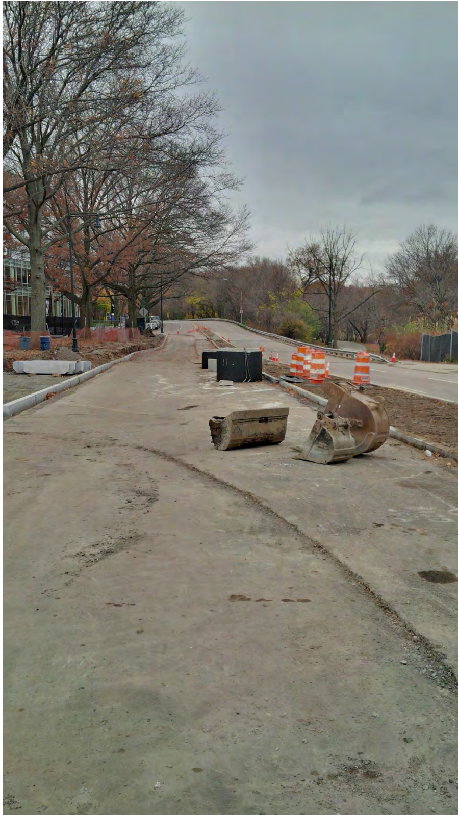
Construction of the new left turn from Riverway onto Park Drive – note the constructed new median separating existing outbound Riverway lanes (right side of median) and two new inbound lanes (left side of median) that will soon allow a left turn onto Park Drive – mid November 2015.
