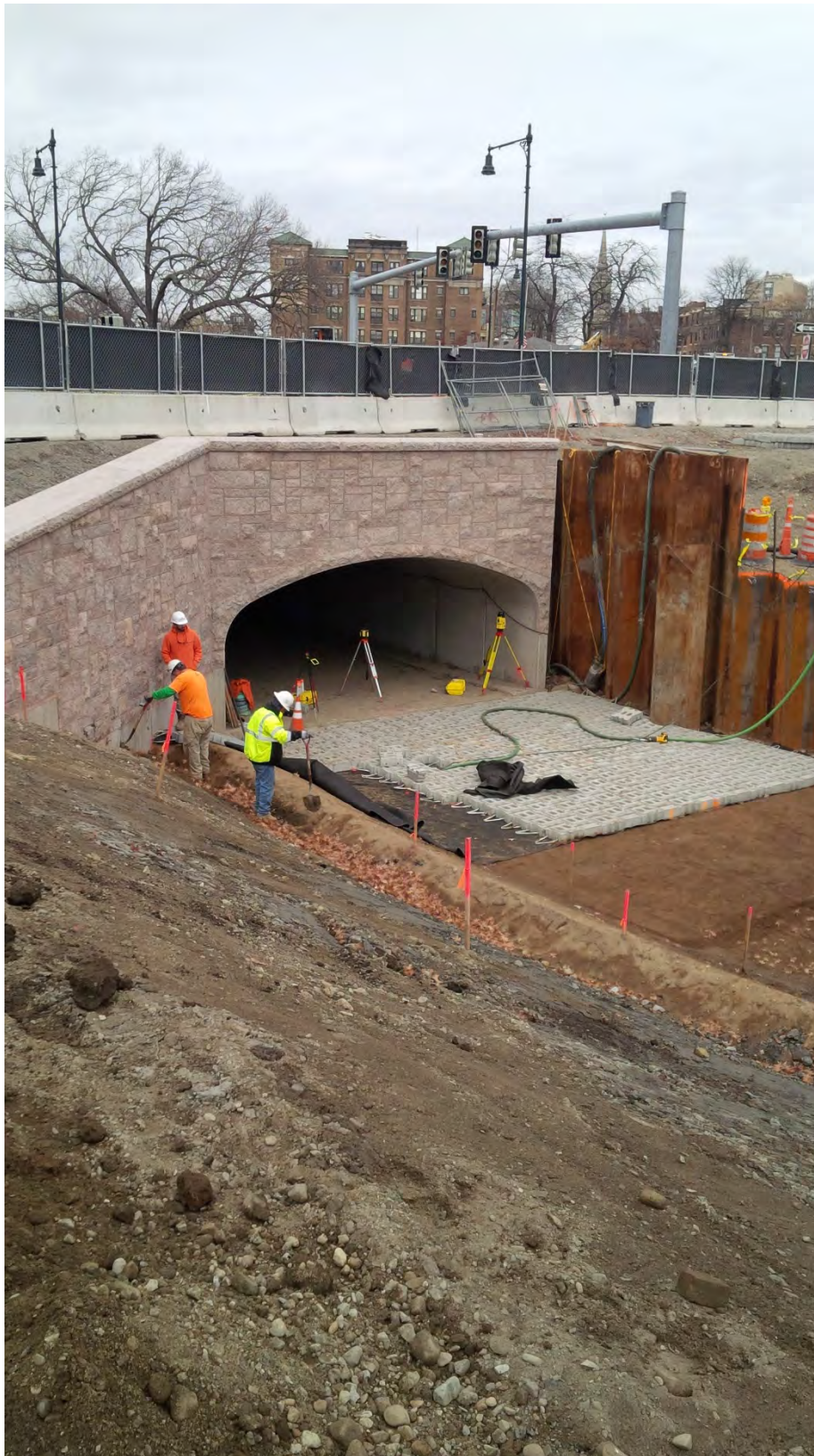
Installation of the Articulated Concrete Blocks (ACBs) for scour protection downstream of the new Riverway Culvert – mid November 2015.
