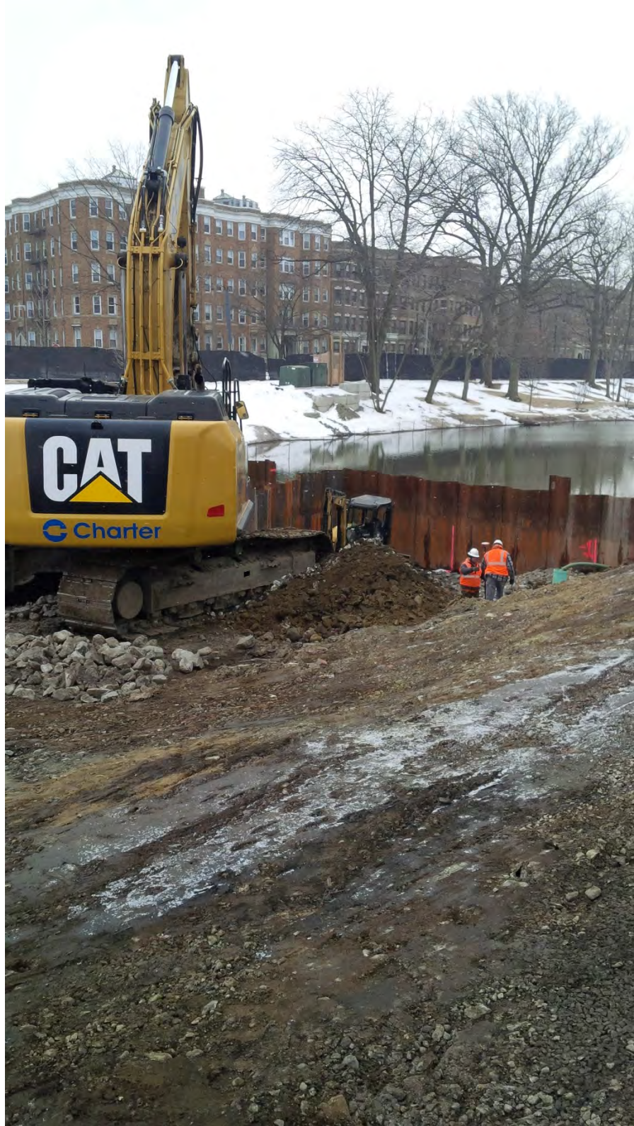
Excavating last of the material from the southside for the flood risk management channel in Jug Handle work area. Note the steel sheeting cofferdam will be lowered to allow the Muddy River to flow through the new culverts – mid February 2016.
