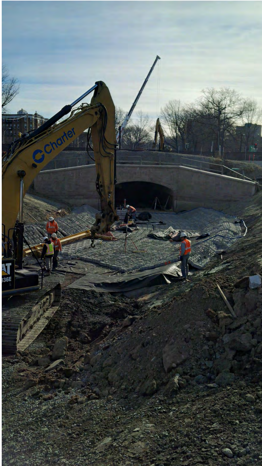
Installation of the articulated concrete blocks (ACBs) at the upstream of the Brookline Avenue culvert – early January 2016.
