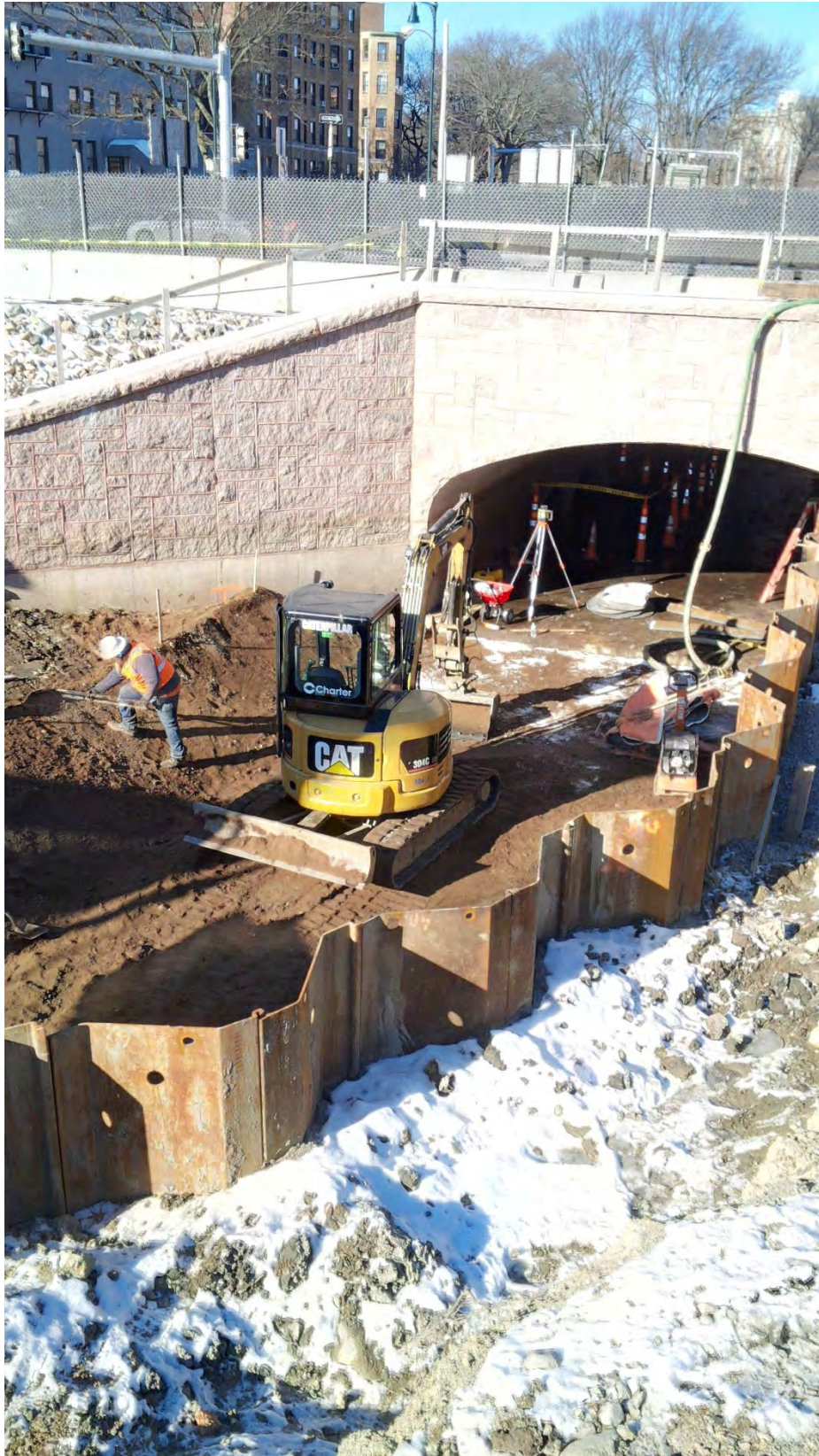
Excavating downstream of the new Brookline Avenue culvert in the Jug Handle work area – late January 2016.
