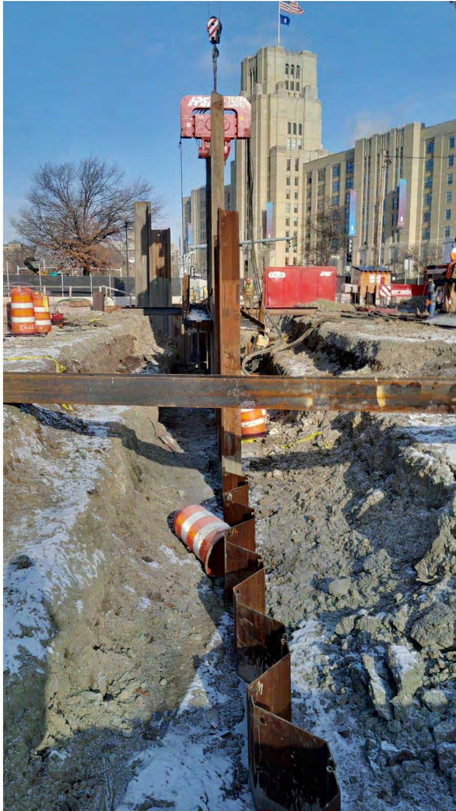
Installation of the steel sheeting support of excavation roughly in the middle of the Jug Handle work area in order to excavate for the southside of the FRM channel, while maintaining flow in the existing twin 72" culverts – mid January 2016.
