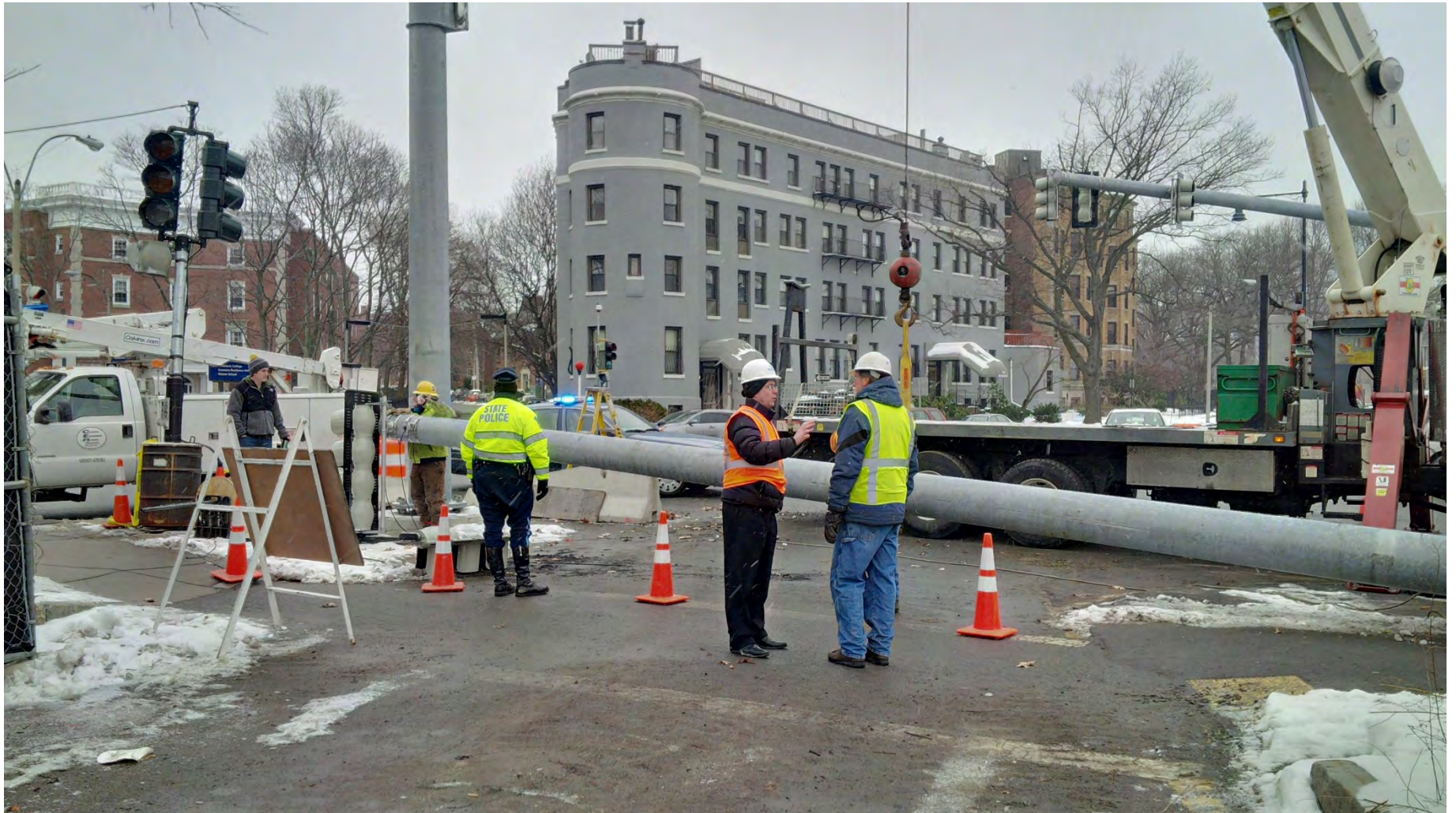
Last of the mast arm for traffic lights being installed at the corner of Fenway, Brookline Avenue, and Riverway Connector – mid February 2016.
