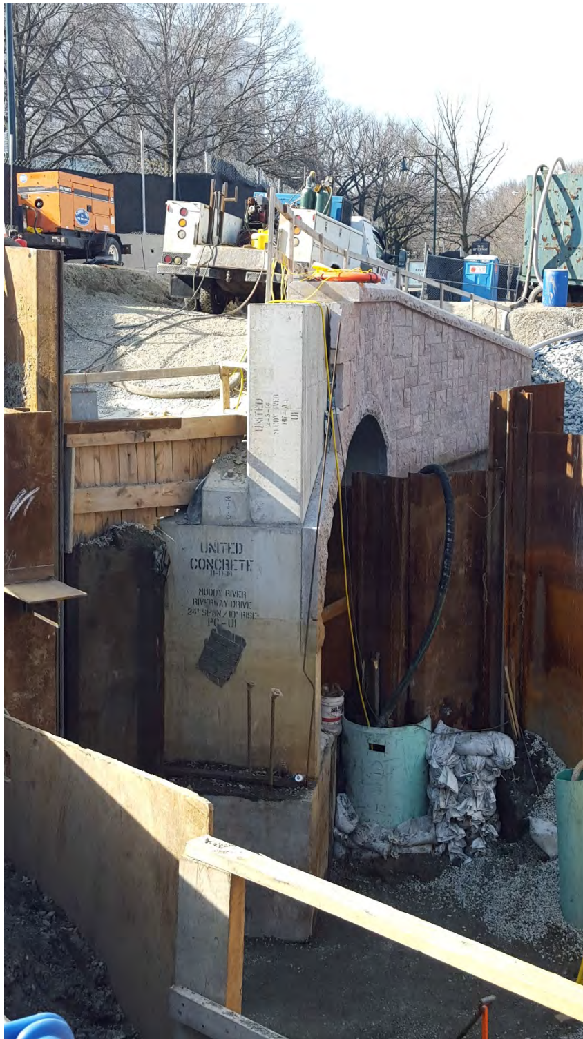
Existing Riverway Intake Structure Removed – Area ready for installation of pipe piles for the upstream northwest wing wall – late March 2016.
