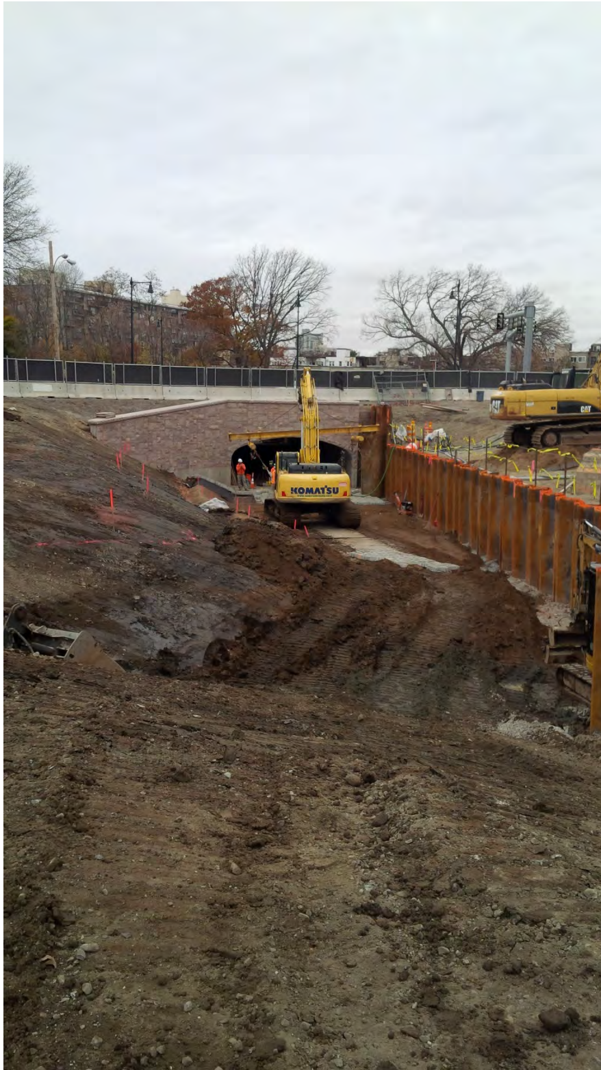
Excavation and shaping of the right (looking downstream) bank of the new river channel downstream of the new Riverway Culvert – mid November 2015.
