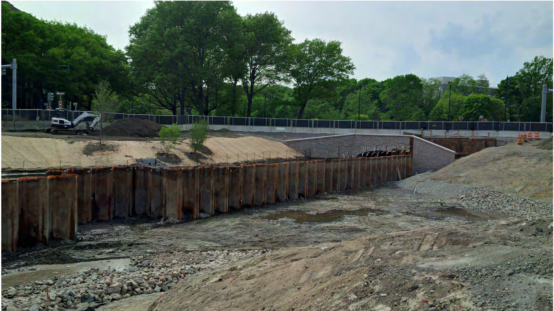
Downstream Riverway Culvert in the former Sears Parking Lot – looking upstream – note the shaping of the bank on the northside to construct the FRM channel and the beginning of planting on the southside of the channel – late May 2016.
