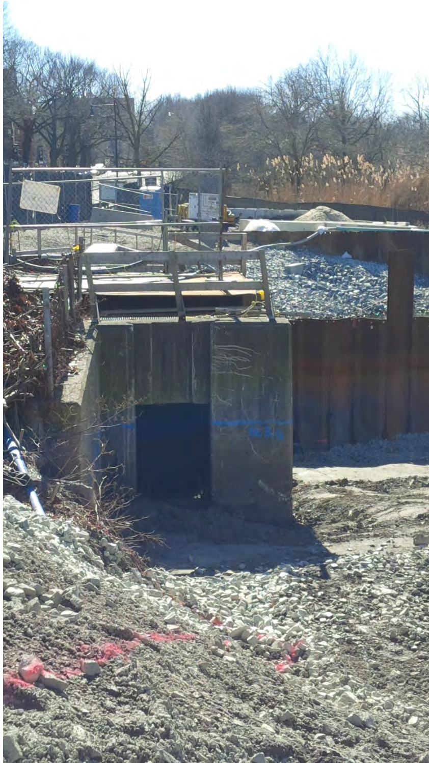
Existing Riverway Intake Structure – note elevation 5.0' marked on the structure for initial partial demolition of the structure – early March 2016.
