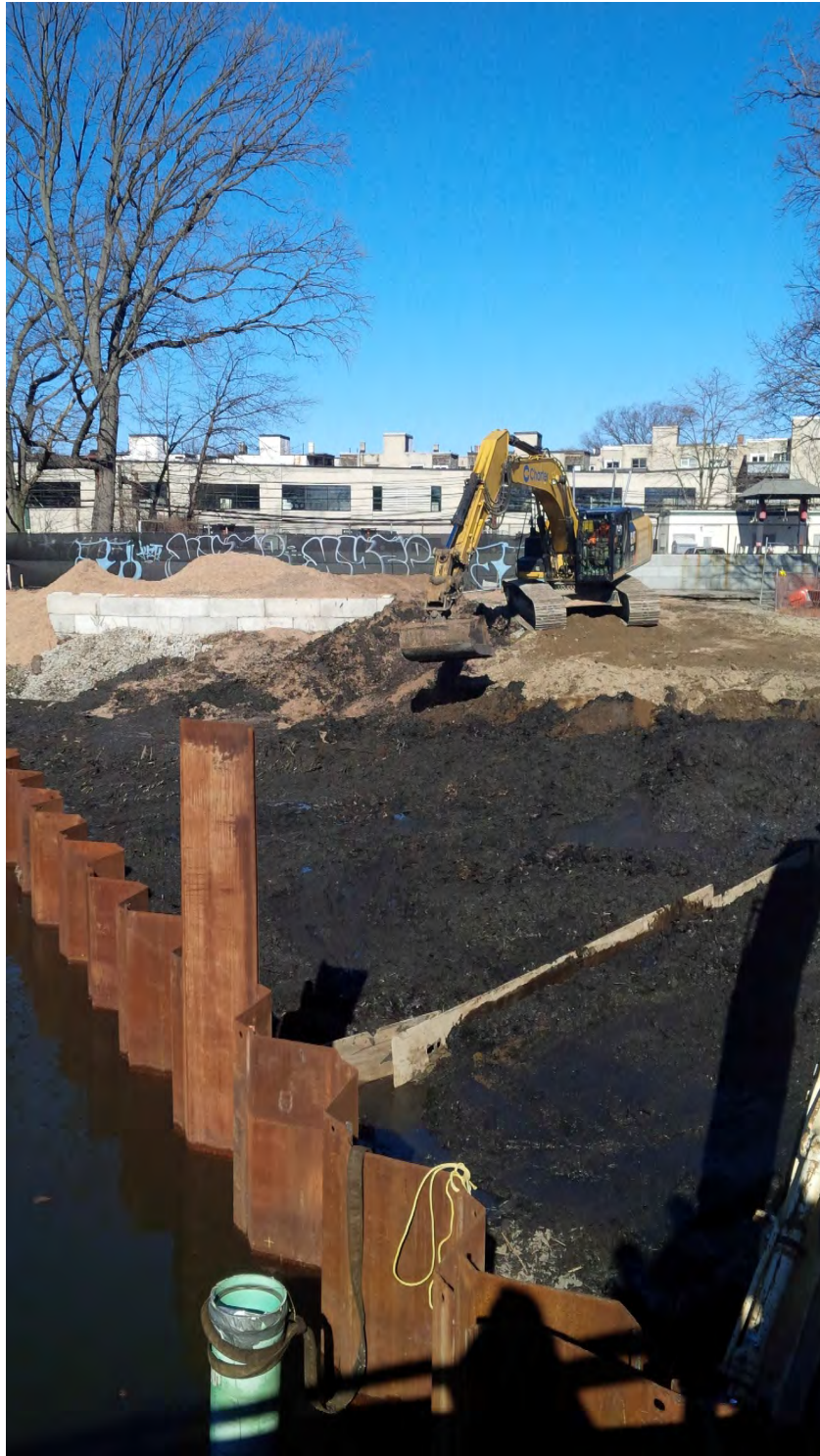
Excavator mixing saw dust into the river sediment to help solidify the material for transport off-site – upstream of the existing Riverway Intake Structure – mid February 2016.
