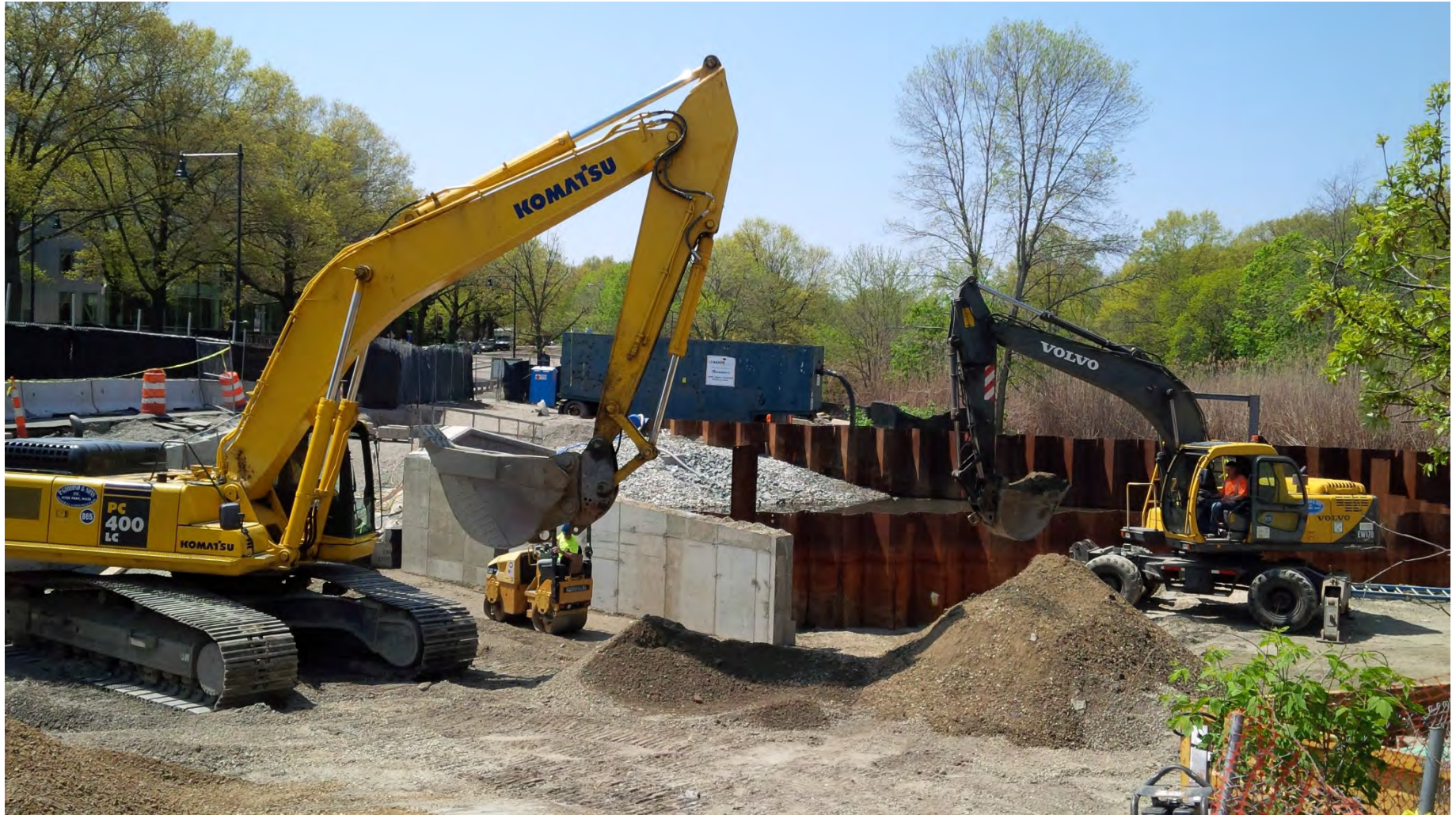
Upstream Riverway Culvert – northwest wing wall cast and backfilling behind the headwall – mid-May 2016.
