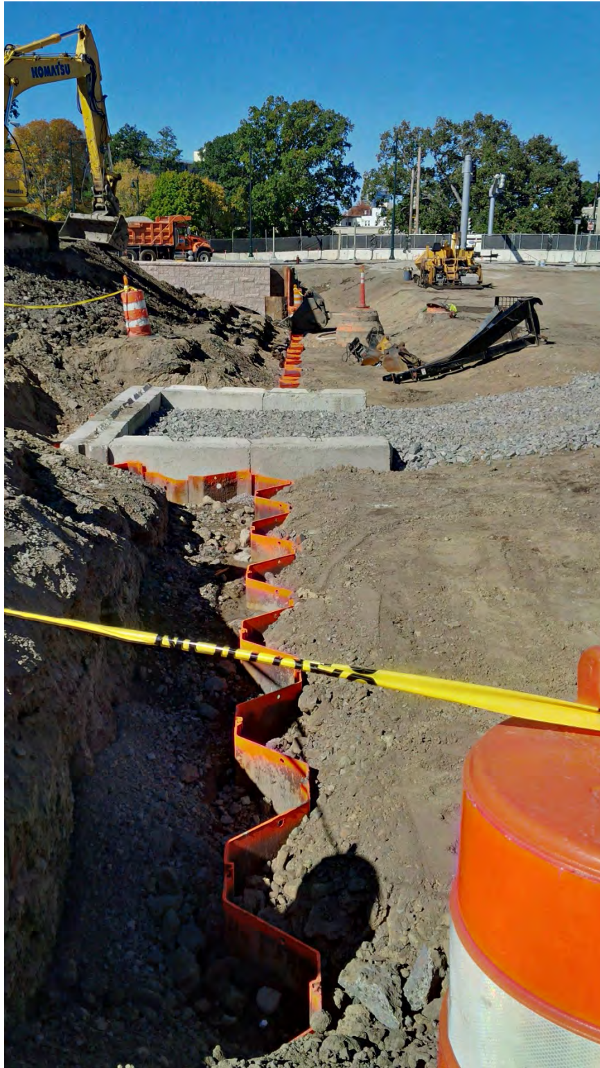
Steel sheeting installed for the river diversion in the pre-excavated trench in the former Sears Parking Lot – note the box-out for the existing storm drainage system – mid October 2015.
