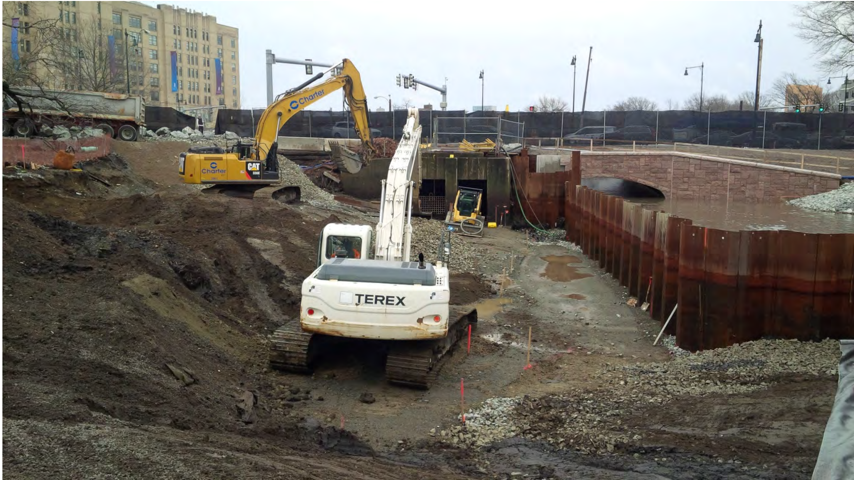
Excavating the sediment to construct the floor risk management (FRM) channel on the left side (looking downstream) of the river. Note the existing Riverway Intake Structure and the new Riverway Culvert in the background – late February 2016.
