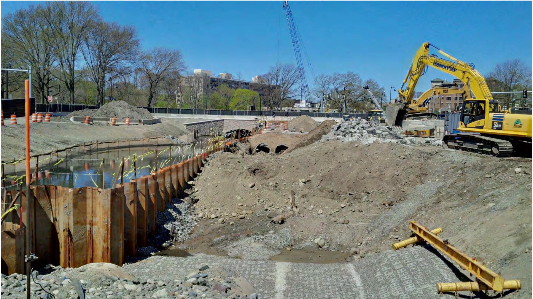
Excavation and removal of the existing twin 72" culverts in the former Sears Parking Lot – looking upstream at the new Riverway Culvert – note the articulated concrete blocks (ACBs) on the constructed channel bottom near Brookline Avenue (nearside) and the existing twin 72" culverts (farside) – late April 2016.
