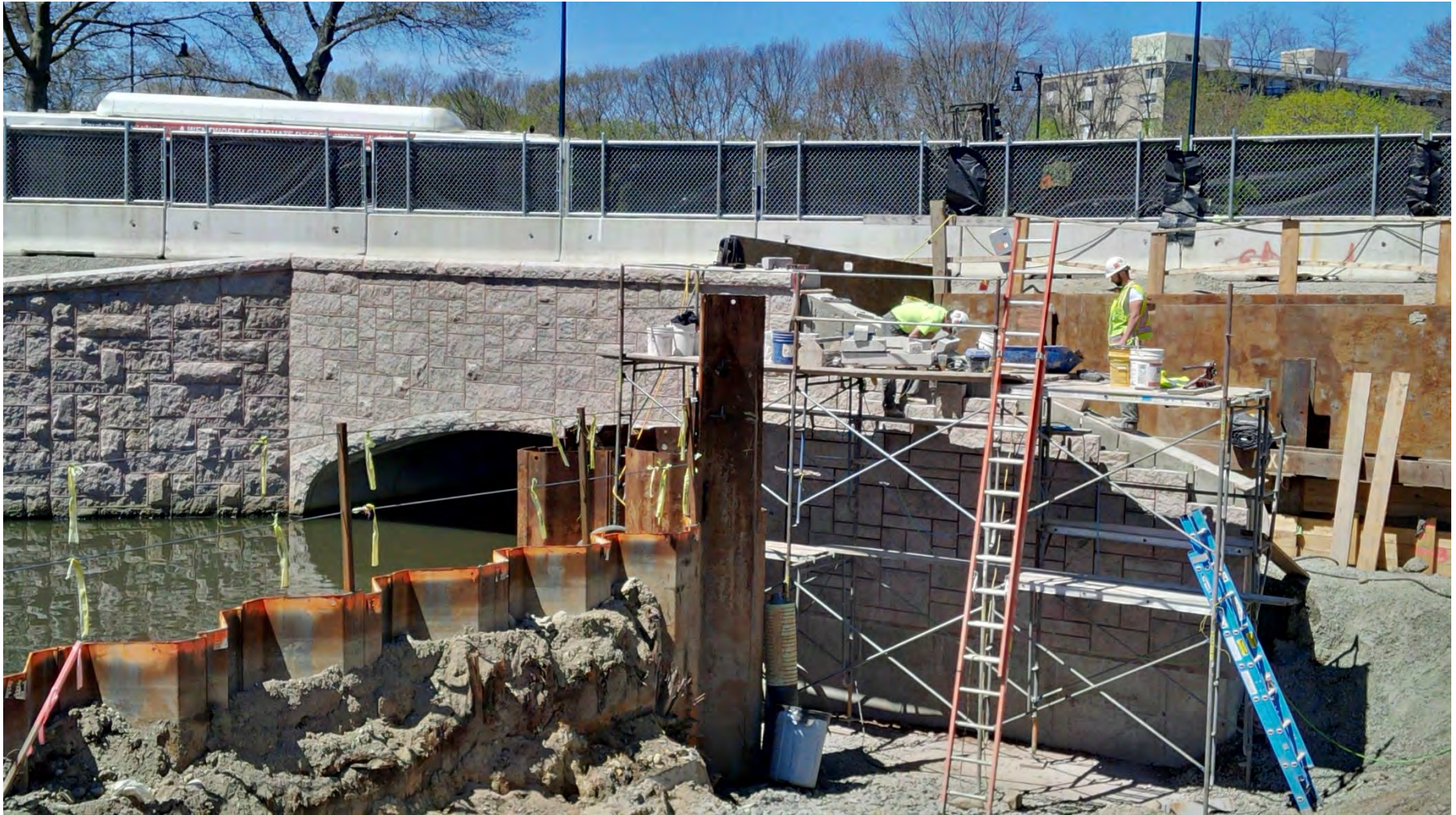
Downstream of Riverway Culvert – granite veneer being installed on the constructed northeast wing wall – late April 2016.
