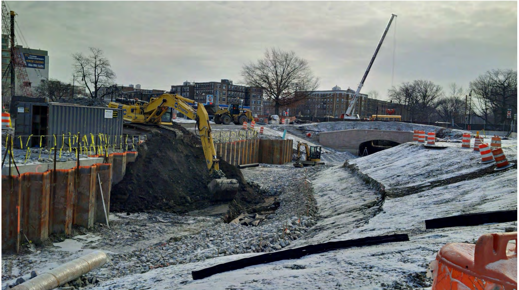
Excavating the last of the material from the southside of the former Sears Parking Lot to form the new flood risk management channel – mid January 2016.
