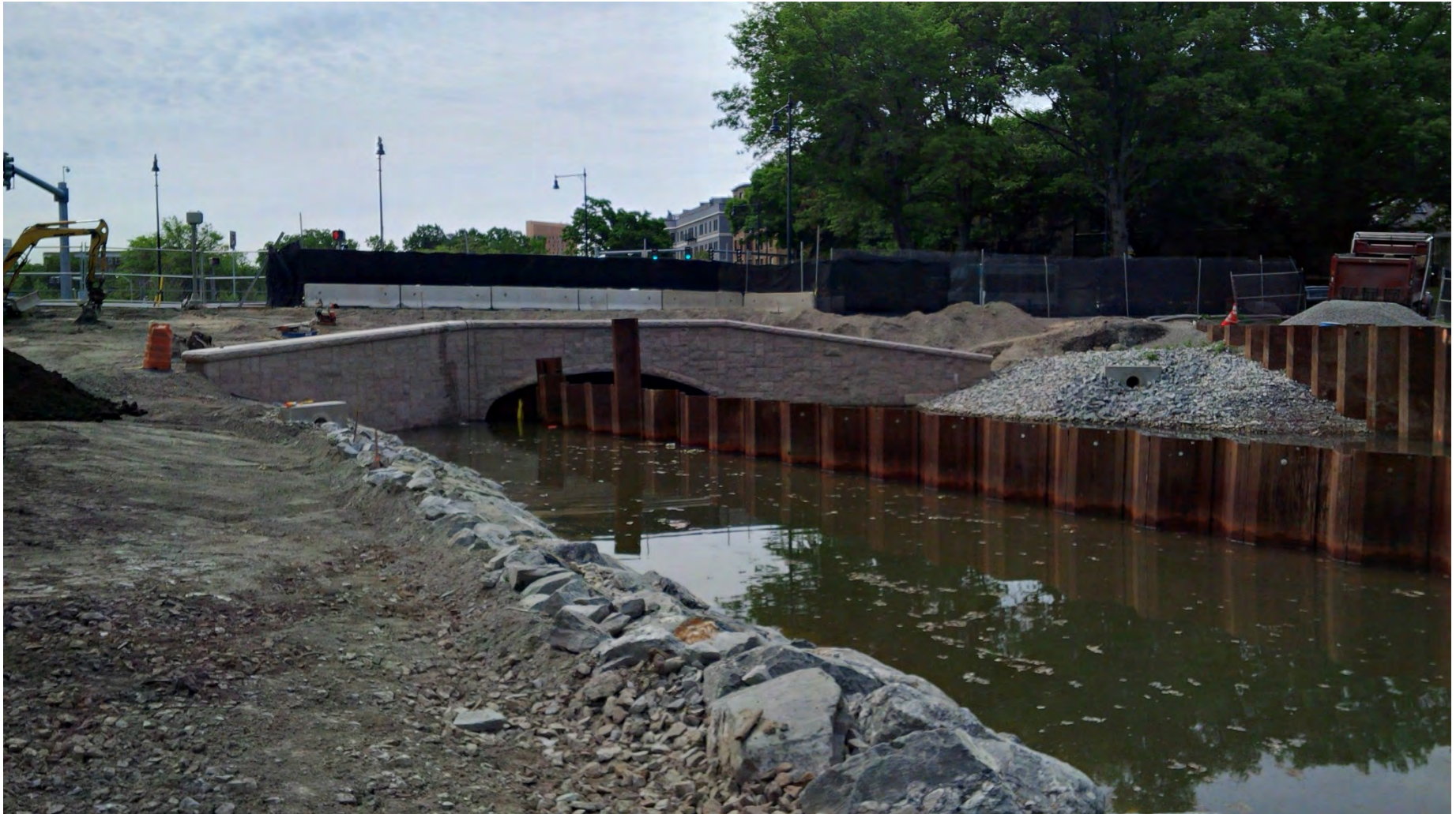
Upstream Riverway Culvert – river pumped into the left side, looking downstream, (northside) of the FRM channel in anticipation of extracting the river diversion steel sheeting; continued backfilling behind the wing wall; and beginning of loam and planting on the upland bank – mid June 2016.
