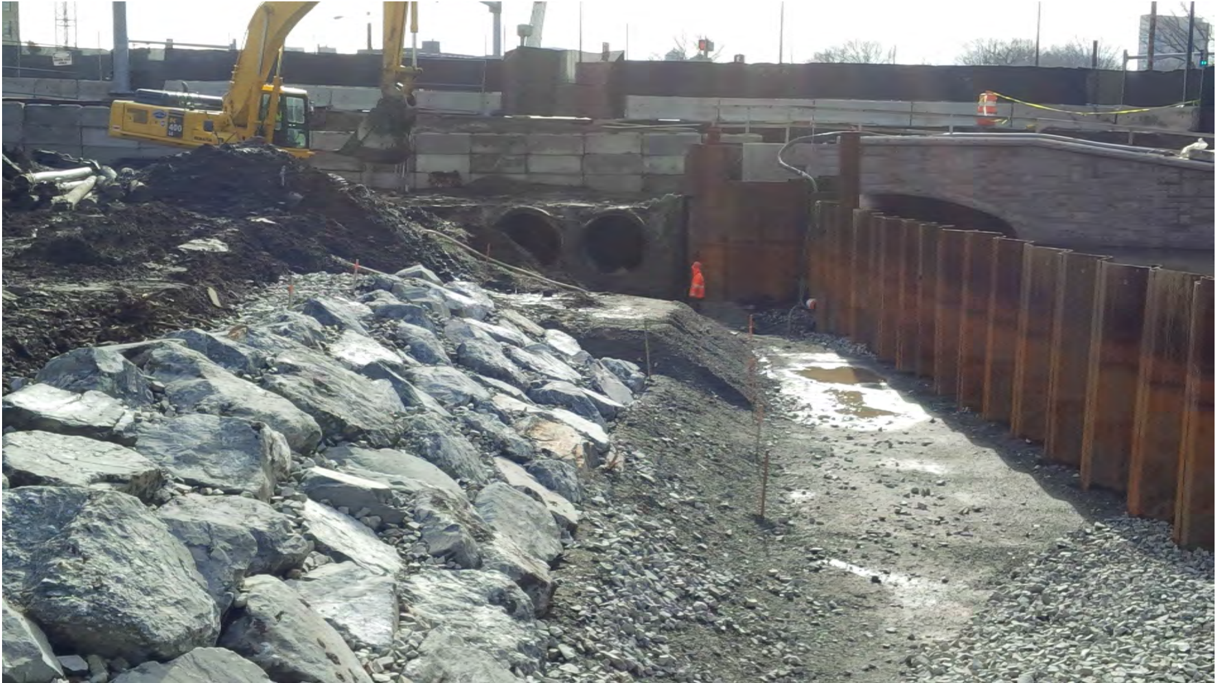
Partial removal of the existing Riverway Intake Structure – down to the existing twin 72” culverts. Note also the part of the new FRM channel and bank is constructed – mid March 2016.
