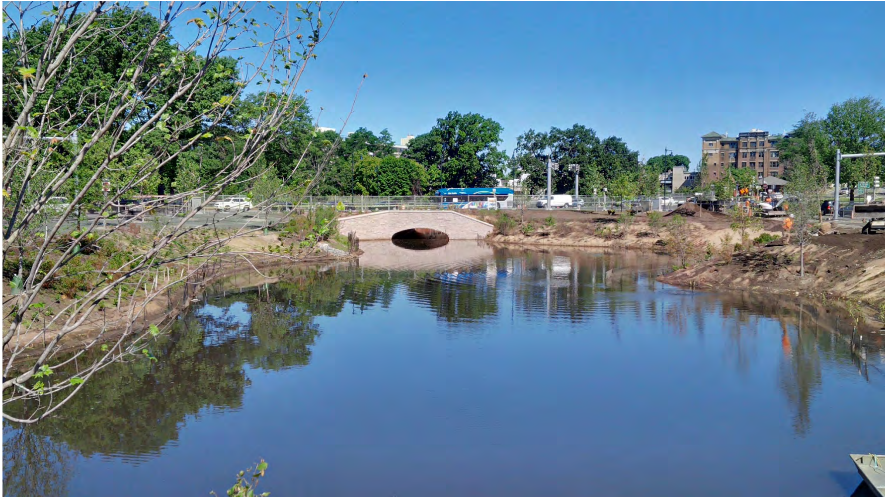
View of downstream of the new Riverway Culvert at the former Sears Parking Lot, with river diversion sheeting removed and plantings on the banks of the constructed FRM channel – 30 June 2016.
