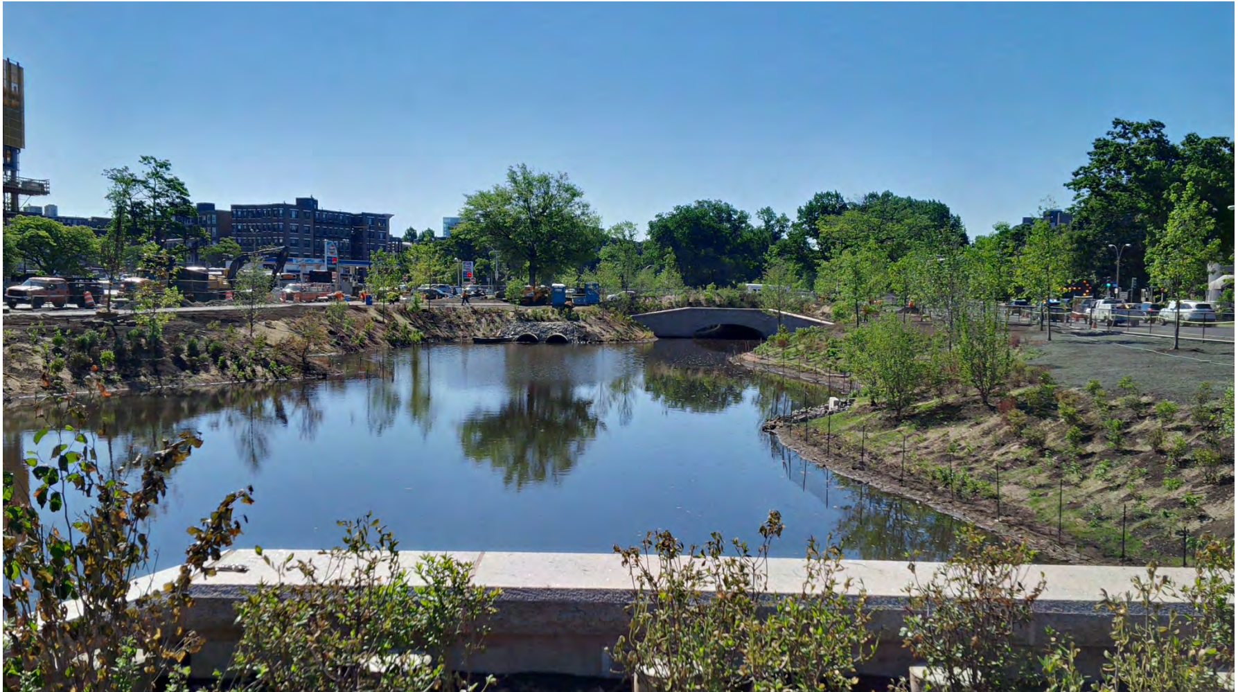
View of upstream of the new Brookline Avenue Culvert at the former Sears Parking Lot, with river diversion sheeting removed and plantings on the banks of the constructed FRM channel – 30 June 2016.
