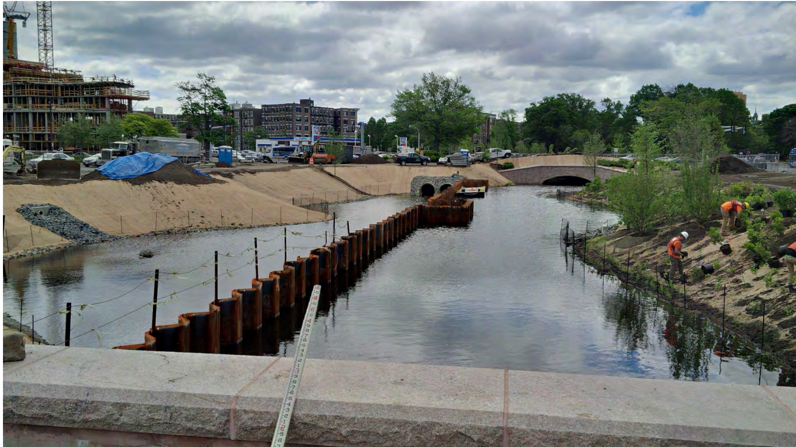
Former Sears Parking Lot – looking downstream at the new Brookline Avenue Culvert – filling of the left side, looking downstream, of the FRM channel once the lower portion of the channel was constructed; note the continued planting on the right side (southside) of the bank of the channel – early June 2016.
