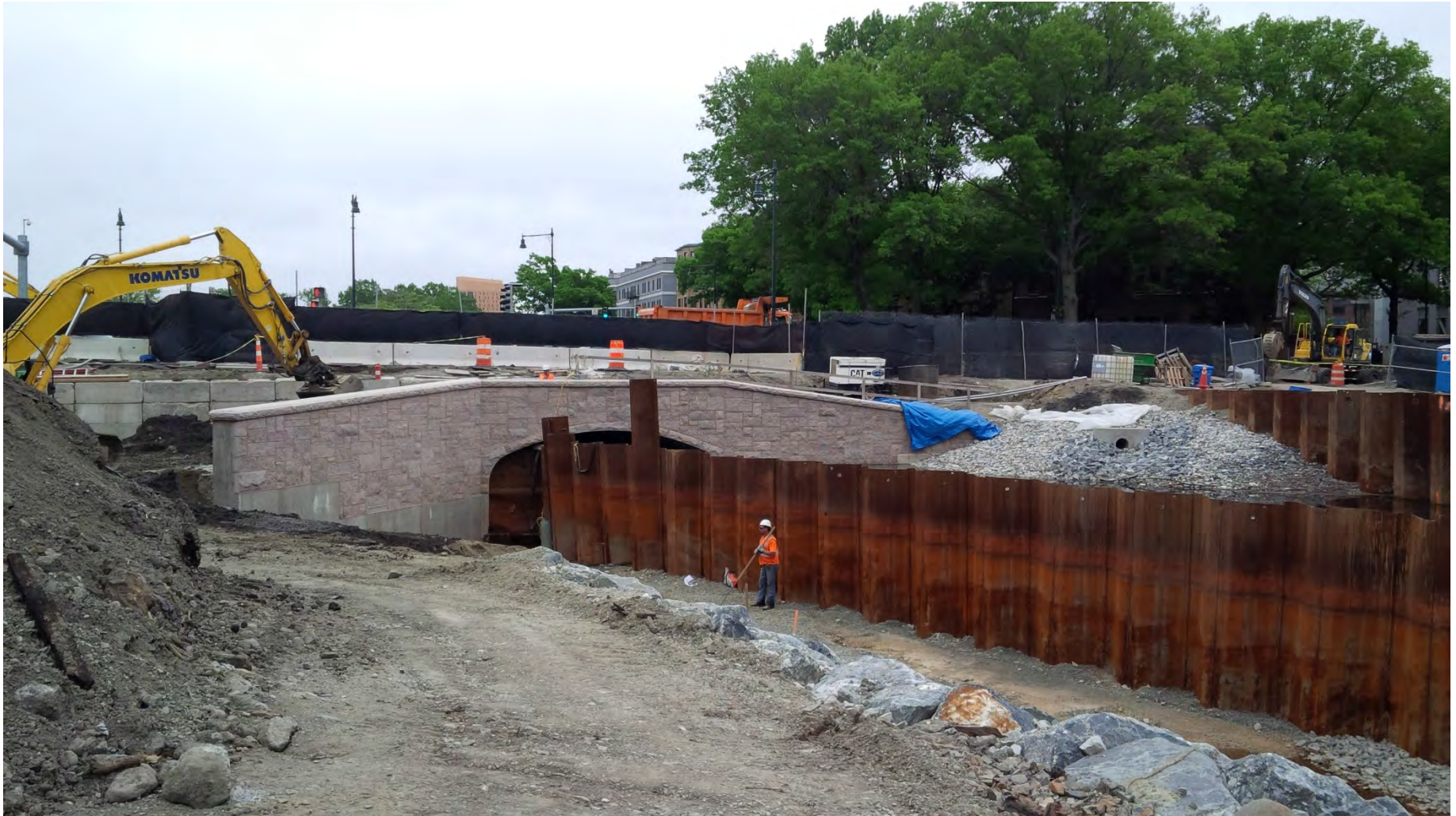
Upstream Riverway Culvert – granite veneer installed and continued backfilling behind the wing wall and shaping of the Flood Risk Management (FRM) channel on the northside – early June 2016.
