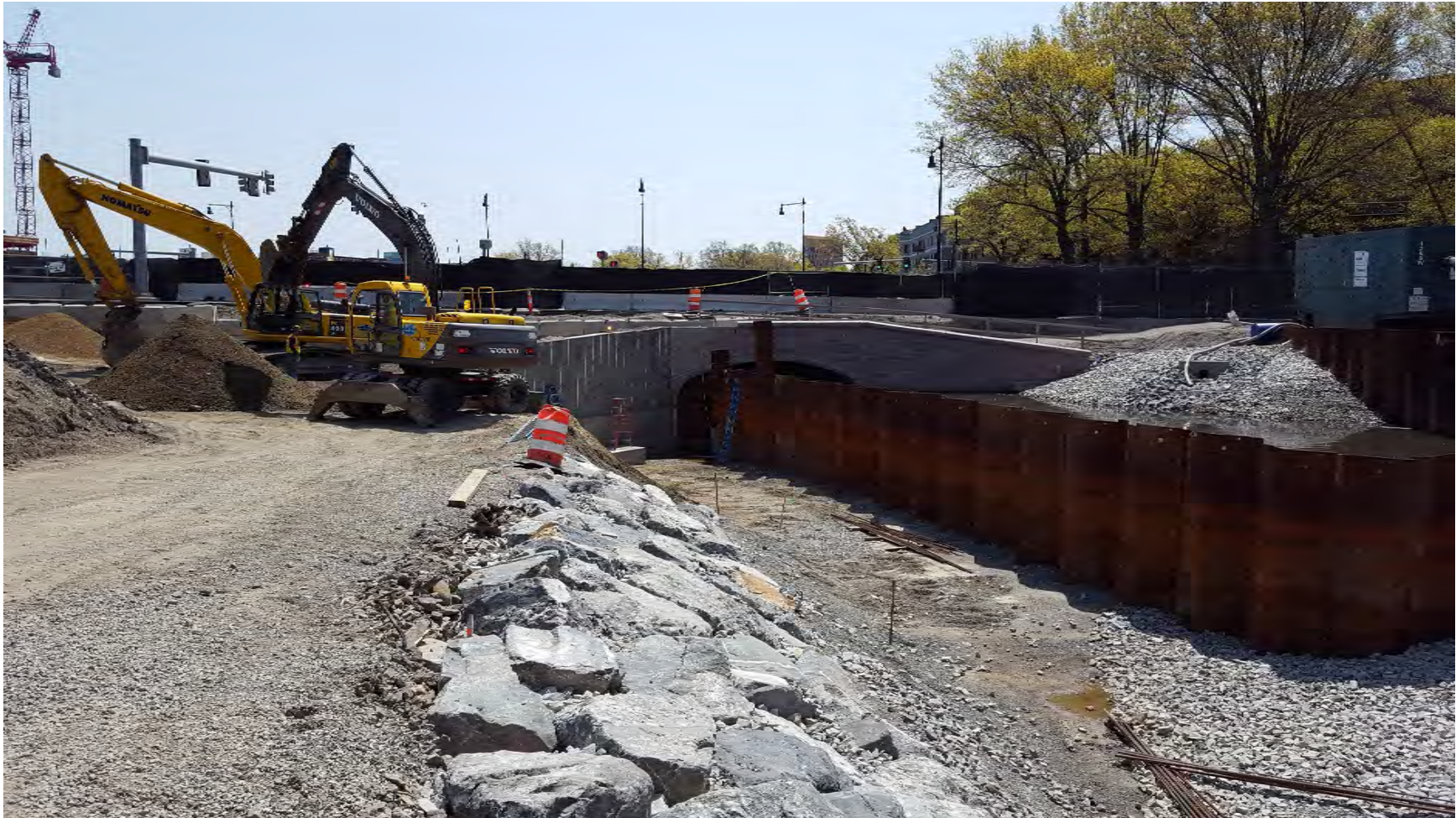
Upstream Riverway Culvert – northwest wing wall cast and ready for granite veneer installation and continued shaping of the flood risk management (FRM) channel – mid-May 2016.
