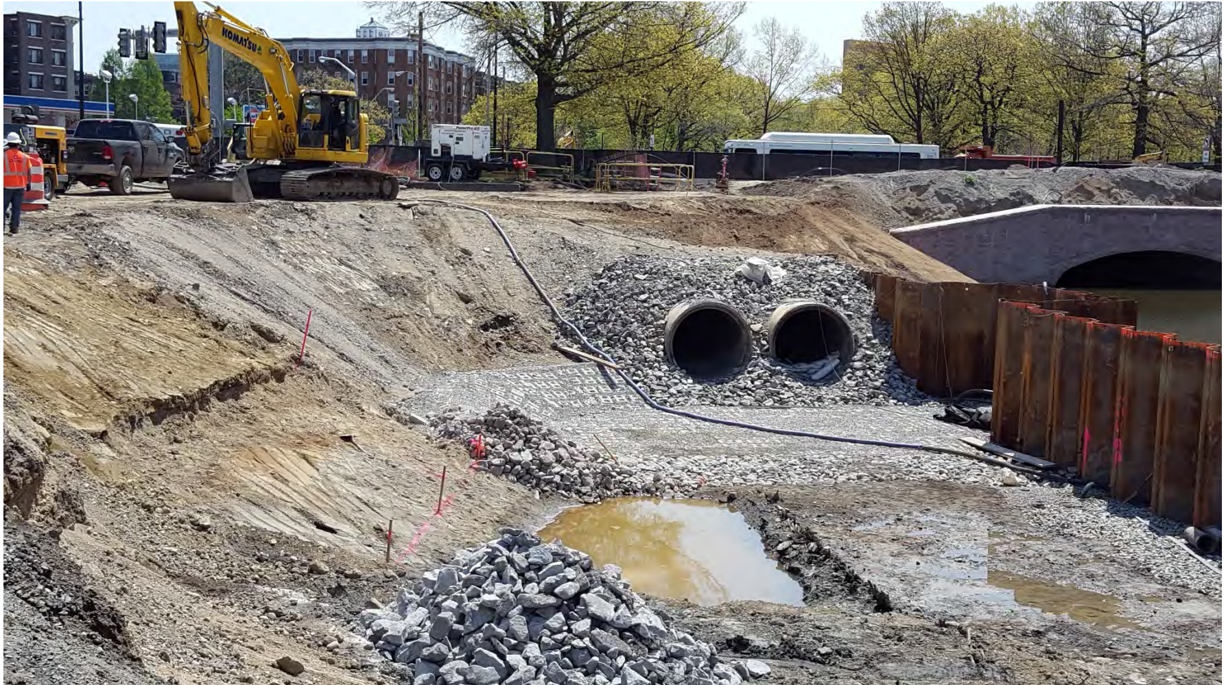
Sections of the existing twin 72" culverts that will remain as part of an overflow connection which ties into the existing underground Brookline Avenue Gatehouse and Conduit – note the new Brookline Avenue Culvert on the right side – mid-May 2016.
