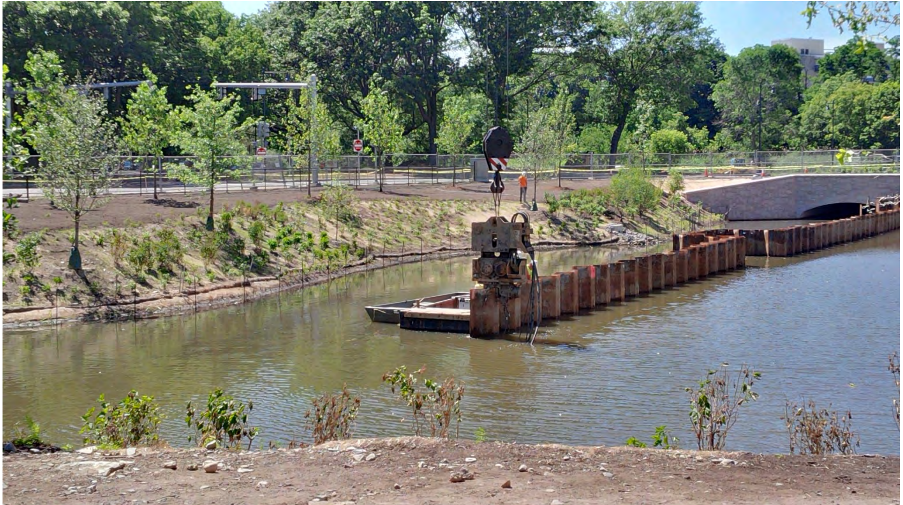
Sections of river diversion steel sheeting removed – view looking at the downstream of the new Riverway Culvert in the former Sears Parking Lot – 21 June 2016.
