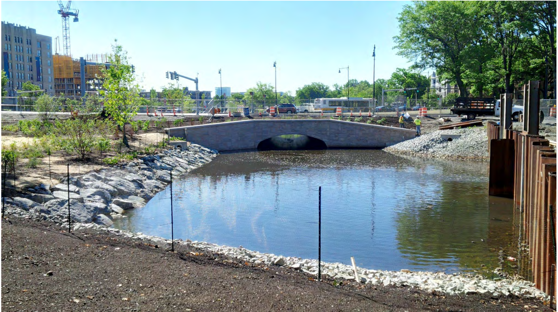
View of upstream of the new Riverway Culvert, with river diversion sheeting removed and plantings on the banks of the constructed FRM channel – 30 June 2016.
