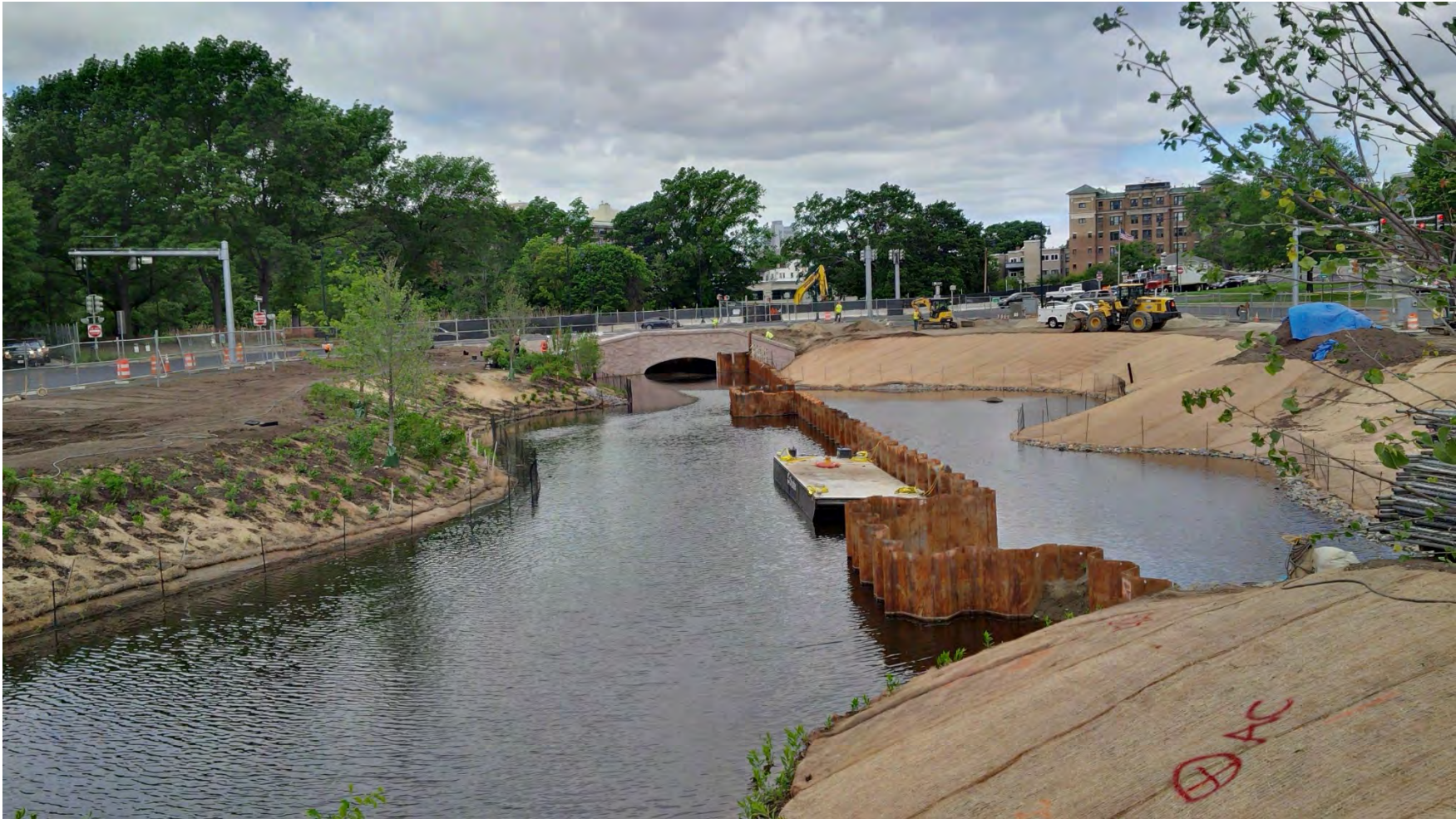
Former Sears Parking Lot – looking upstream at the new Riverway Culvert – filling of the northside of the FRM channel once the lower portion of the channel was constructed; note the continued planting on the southside of the bank of the channel – early June 2016.
