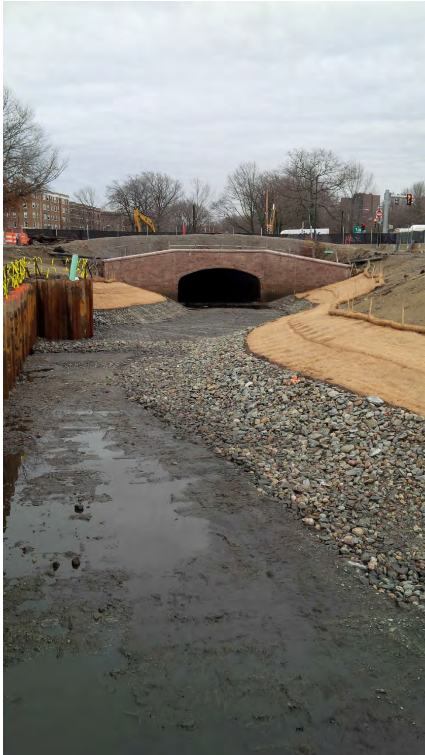
Southside of the flood risk management completed, to include ACB's for channel scour protection, and stone protection, geocells, and turf reinforcement mattress for bank protection – looking at the upstream Brookline Avenue culvert – early February 2016.
