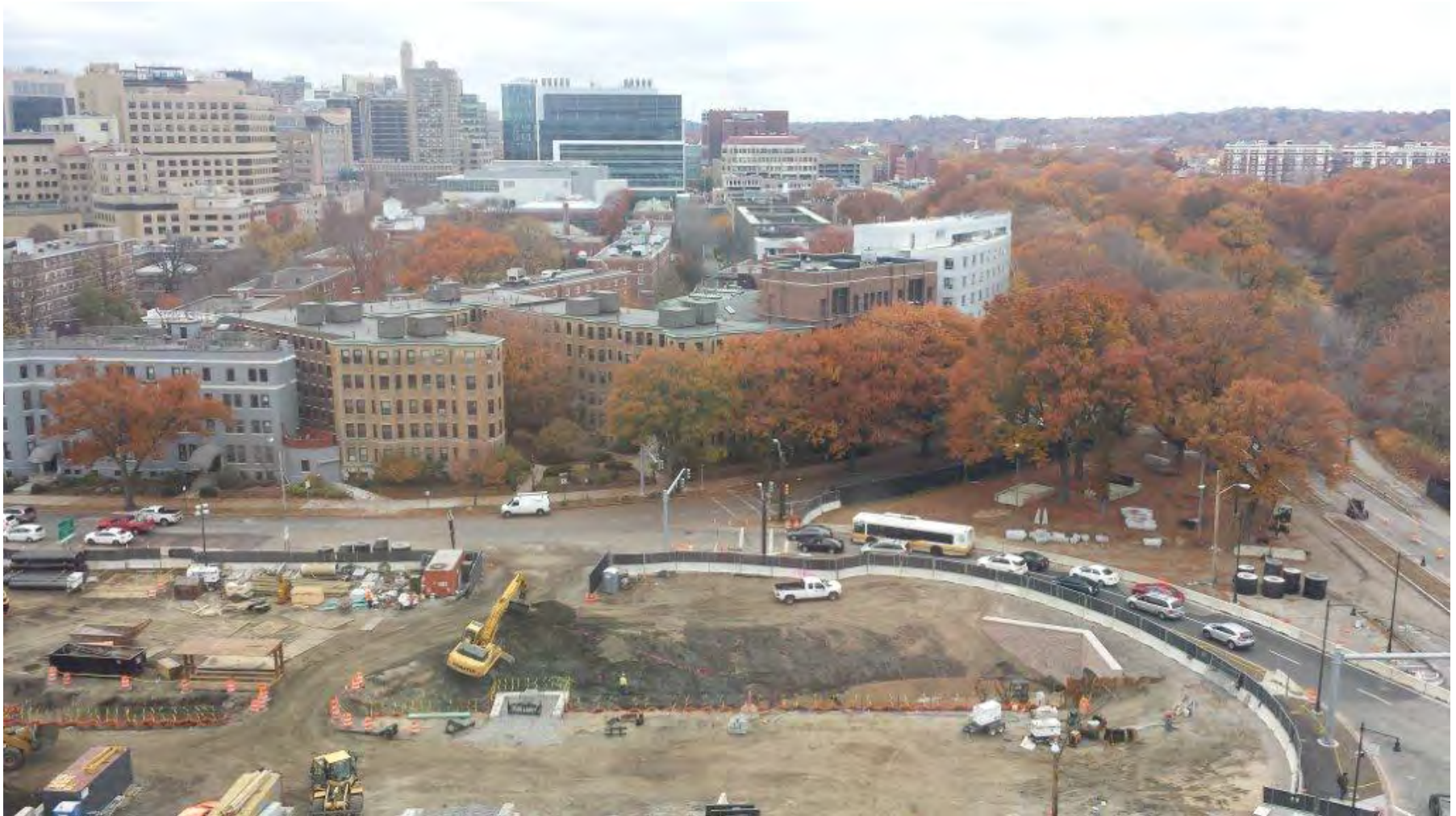
Overview of the former Sears Parking Lot – note the excavation downstream of the new Riverway Culvert to construct the new river channel to return the Muddy River to its natural state – early November 2015.
