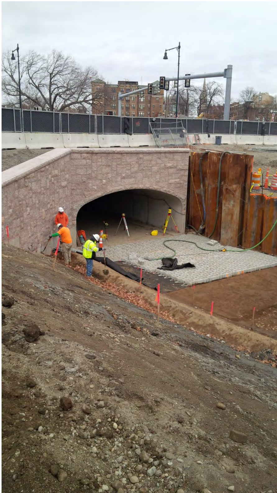
Installation of the Articulated Concrete Blocks (ACBs) for scour protection downstream of the new Riverway Culvert – mid November 2015.
