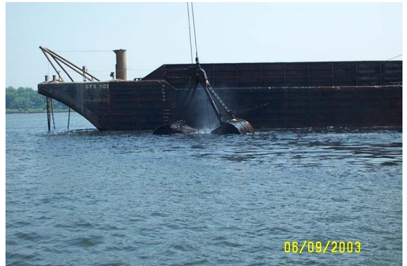
18. Closed bucket entering water (06/09/2003)
