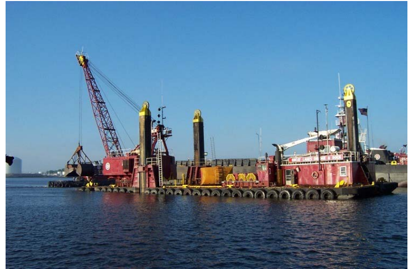
14. Dredge 51 over cell 4R (07/10/2003)
