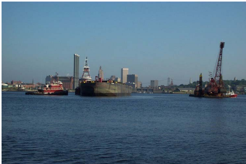
32. Disposal into Cell 3R with ongoing construction of Cell 4R (07/10/2003)
