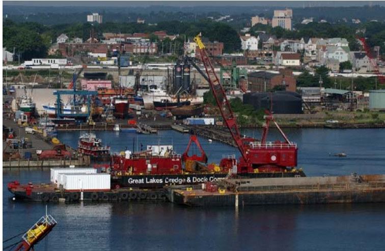
1. Dredge 55 – Construction of Cell 6/7R off of the State Pier (07/30/2003)
