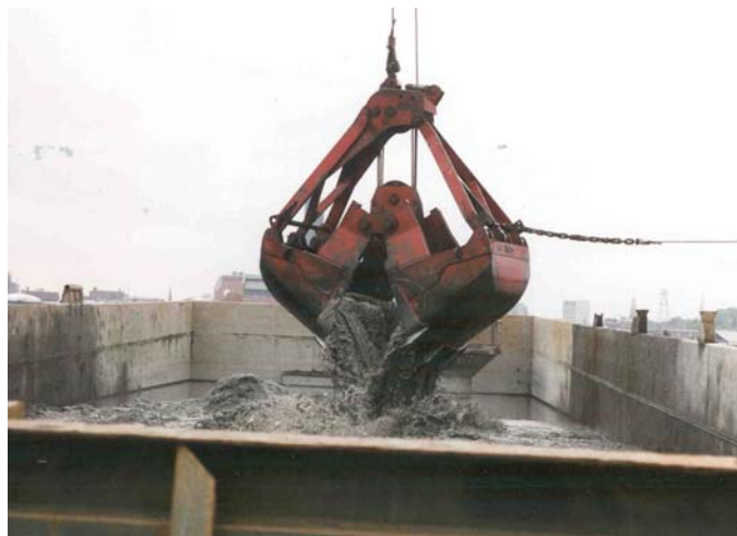
19. Open bucket removing native material in Cell 3R (05/20/2003)
