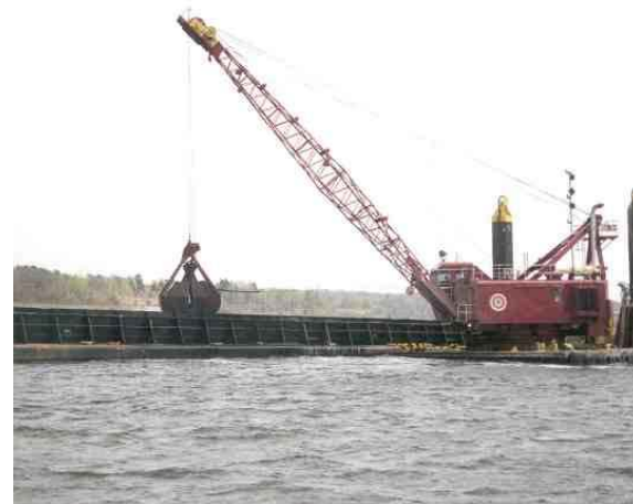
22. Closed bucket removing surficial material over Cell 3R (05/05/2003)
