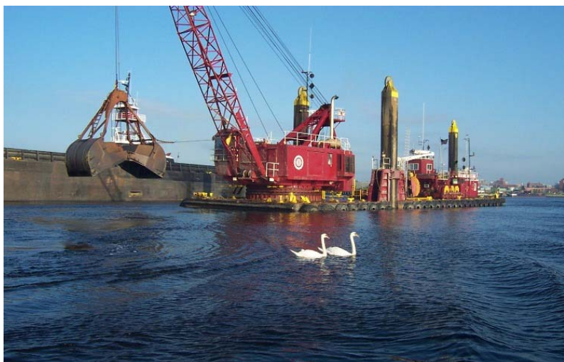
11. Dredge 51 – Construction of Cell 4R (07/10/2003)
