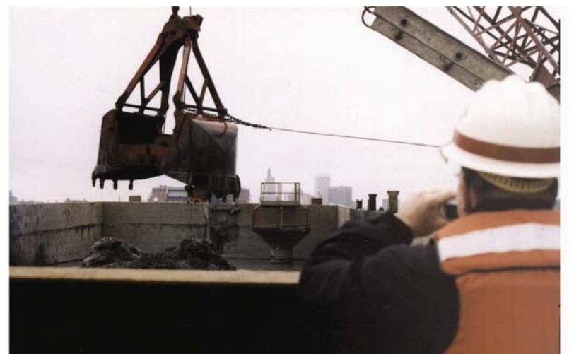
20. Open bucket removing native material in Cell 3R (05/20/2003)
