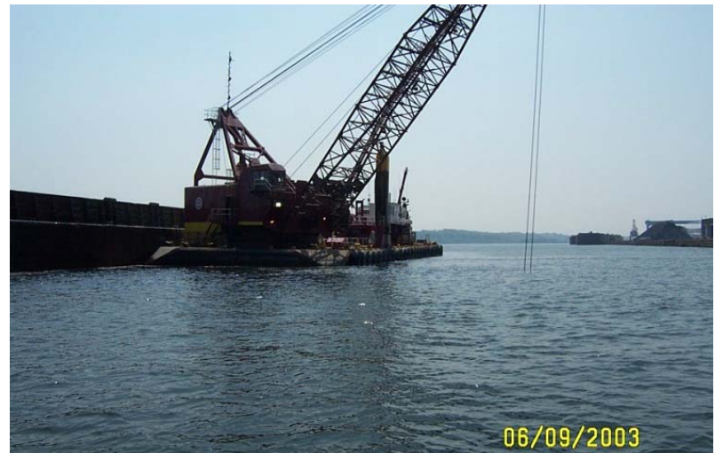
16. Dredge 54 – Construction of Cell 4R (06/09/2003)
