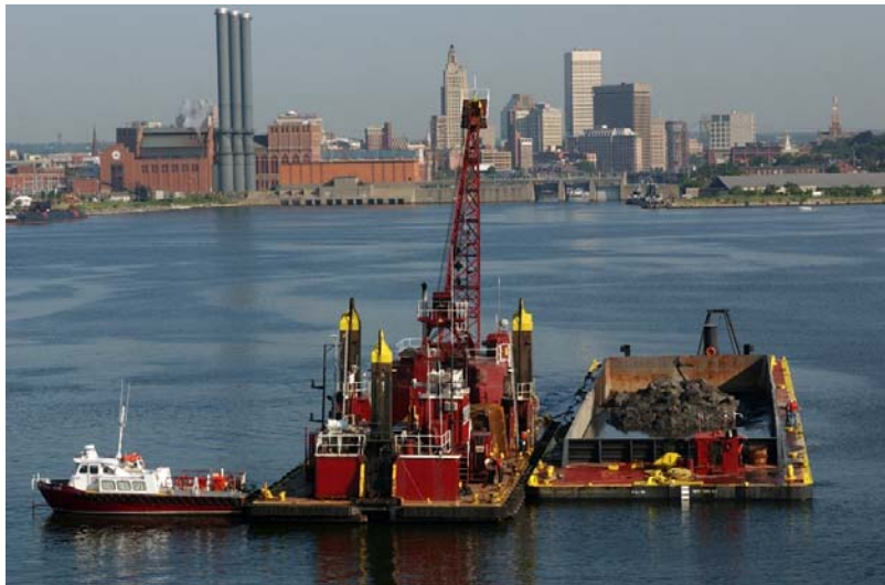
3. Dredge 51 – Construction of Cell 5R (07/30/2003)
