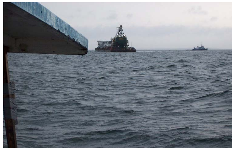
12. Anchoring of Dredge??? (07/07/2003)
