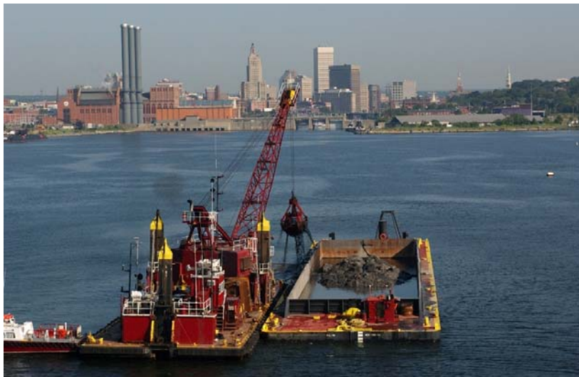
9. Dredge 51 – Construction of Cell 5R (07/30/2003)
