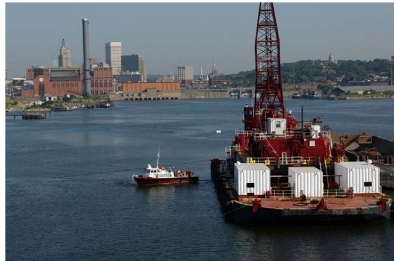
10. Dredge 55 over Cell 6/7R, note hurricane barrier in background (07/30/2003)
