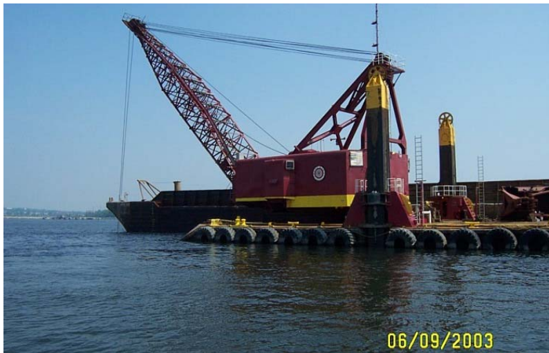
15. Dredge 54 – Construction of Cell 4R (06/09/2003)
