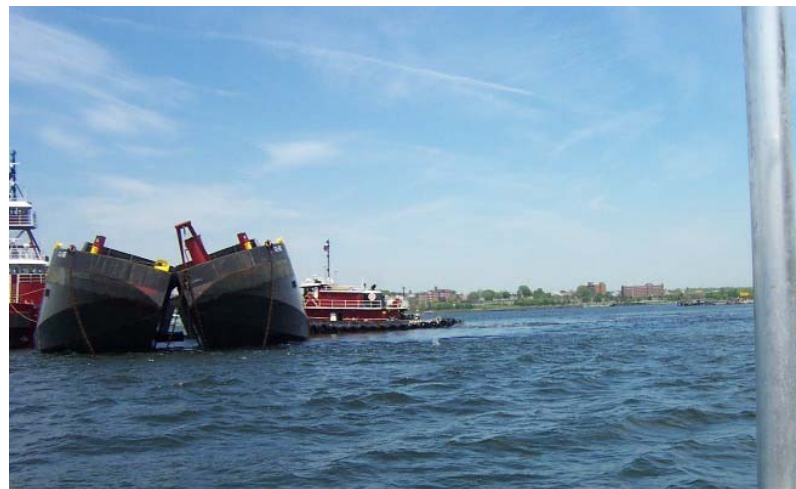
43. Scow fully open over Cell 1R (05/20/2003)
