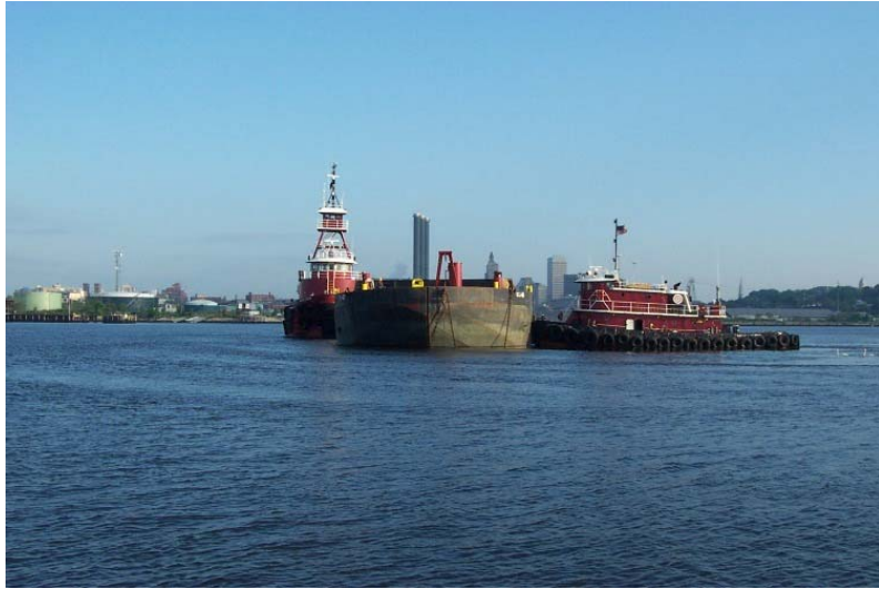
28. Positioning loaded scow over Cell 3R (07/10/2003)
