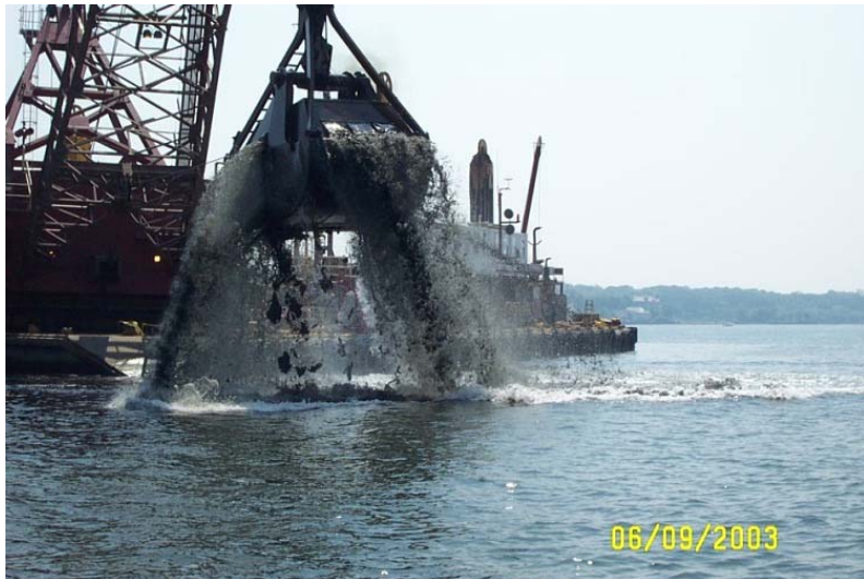
17. Closed bucket removing surficial material over Cell 4R (06/09/2003)
