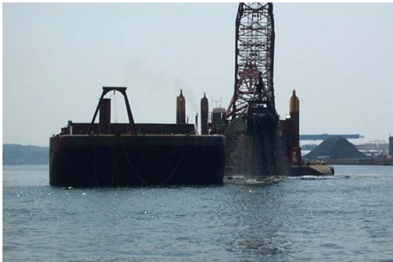
21. Construction of Cell 4R (06/09/2003)
