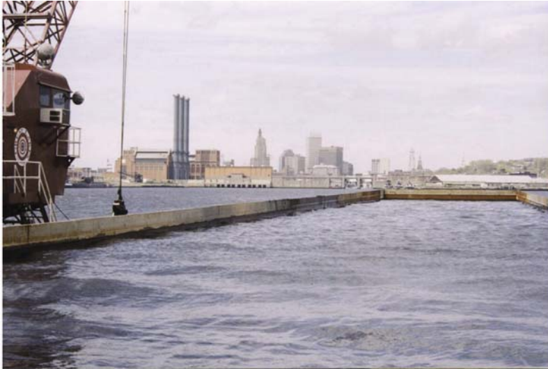
44. Dredging surficial material over Cell 3R (note high water content) (05/20/2003)
