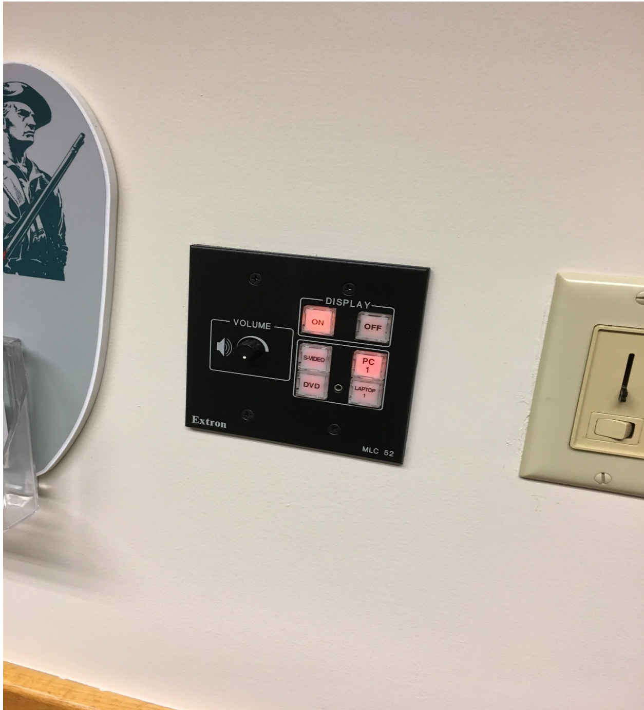
Informational Photo Number 3: Control Panel
