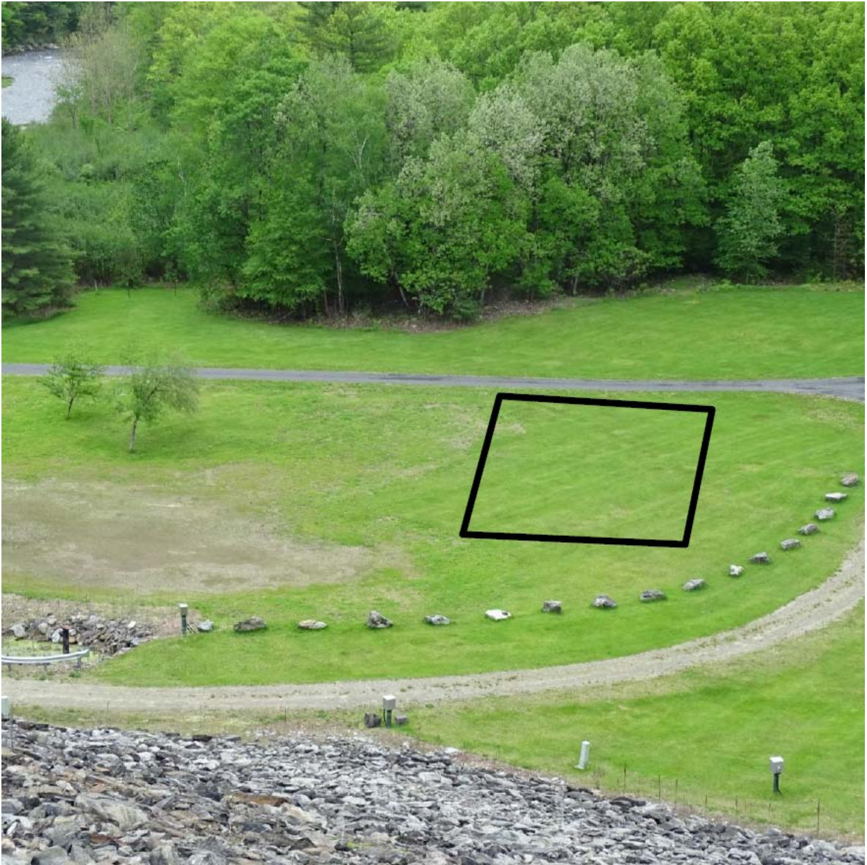
Figure 3: Approximate location of Site B as viewed from the top of Townshend Dam.
