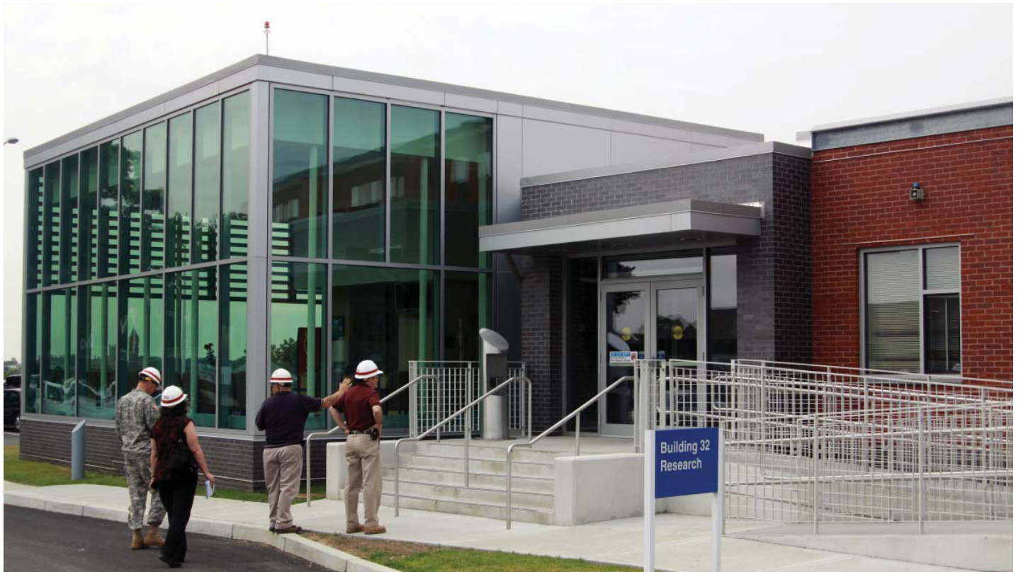
The New England District recently completed this research building at the Veterans Administration Hospital in Providence, R.I.
