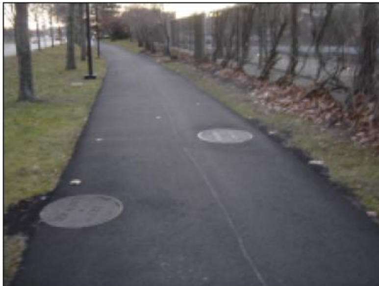
Figure 3.3-6 Utility Structures Along Southwest Corridor Park
