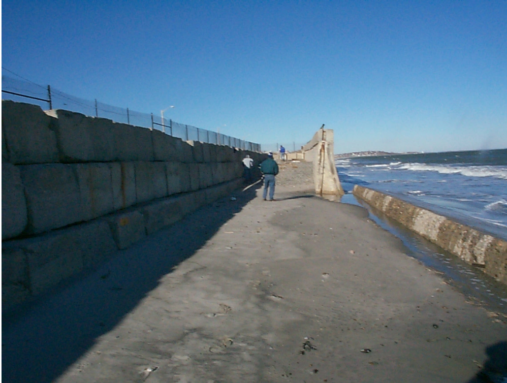
Figure 3 Collapsed Wall Section
