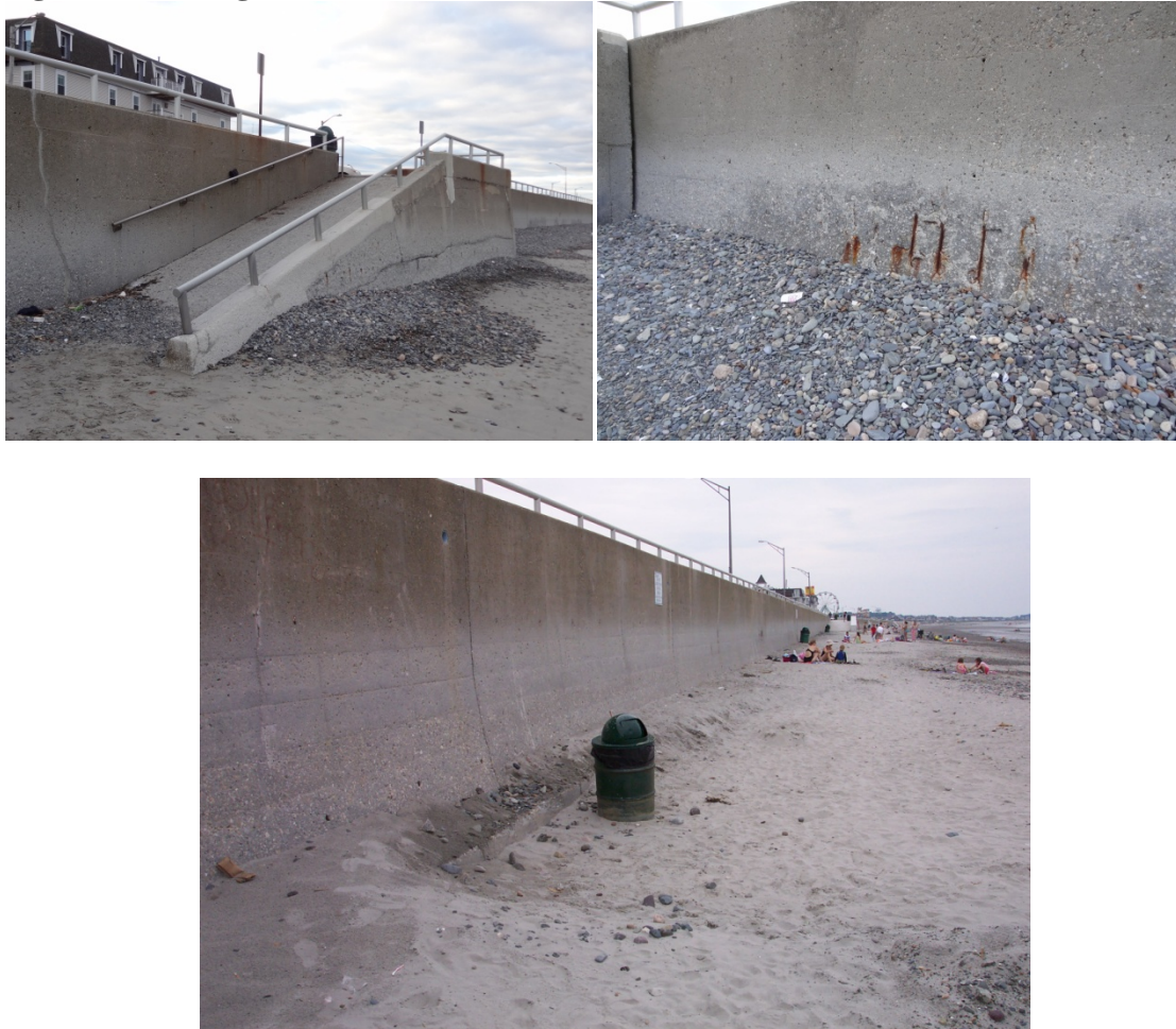
Figure 2 –Damaged Seawall Sections
