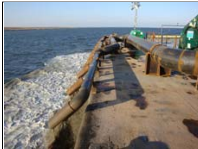
Figure 2.2-5. Spill barge dispersing material along the footprint of the cross dikes.
