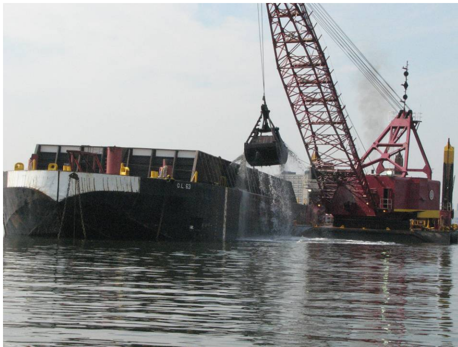
Figure 7. Dredging Operations during Removal of Material over the Main Ship Channel CAD Cell.
