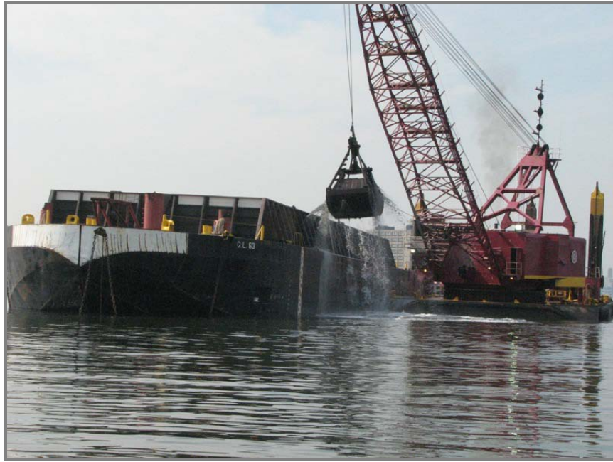
Figure 2. Dredging Operations During Removal of Material Over the Main Ship Channel CAD Cell.
