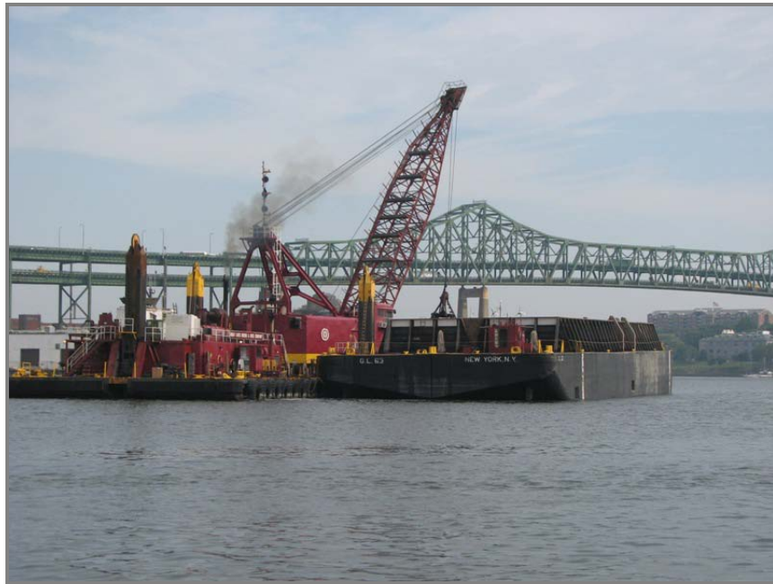
Figure 6. Dredge 54 Operated by Great Lakes Dredge and Dock Company and Scow During Dredging of Silty Layer Over the Main Ship Channel CAD Cell.
