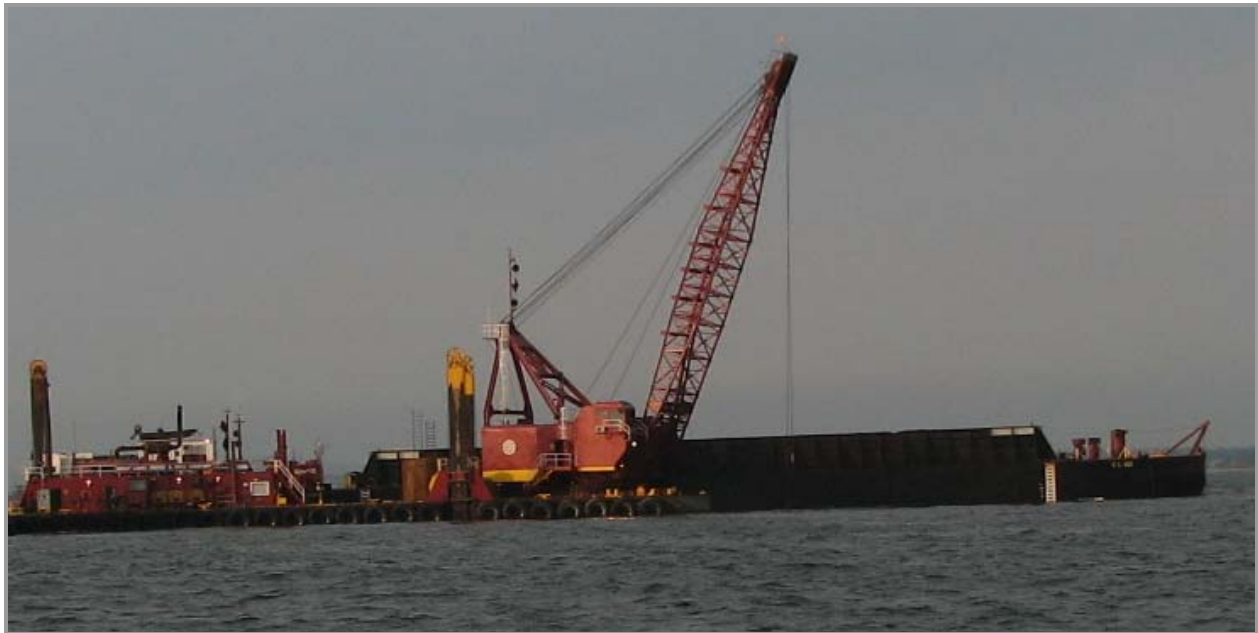
Figure 7. Dredge 54 Operated by Great Lakes Dredge and Dock Company and Scow During Dredging of Maintenance Material in the Lower Harbor.
