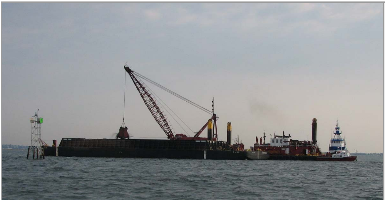
Figure 3. Dredging Operations of Maintenance Material in the Lower Harbor.
