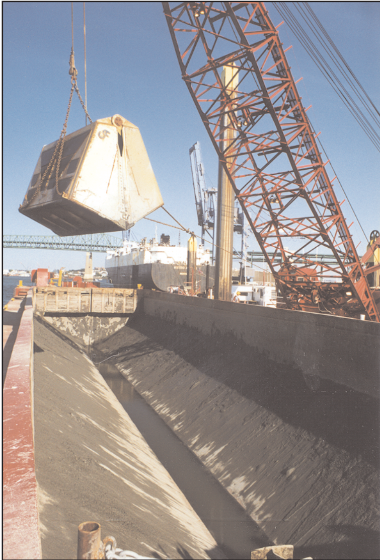
Photo 1 Cable Arm Environmental Bucket in Use in the Mystic River
