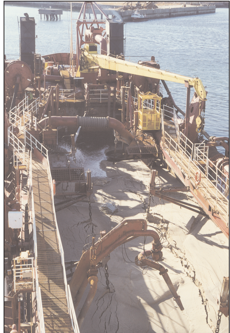
Photo 17 Hopper Dredge Discharging Capping Sand Over Cell M12
