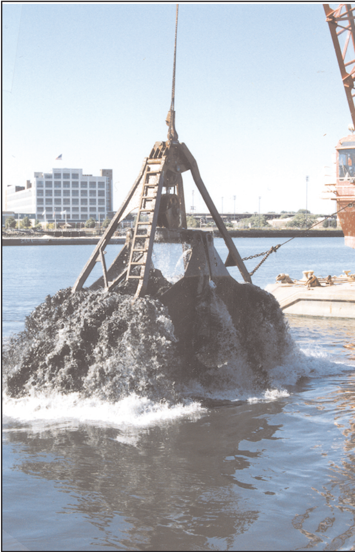
Photo 31 Bucket Exiting Water During Improvement Dredging
