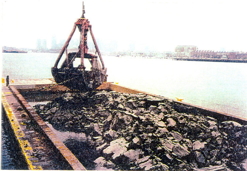
FIGURE 5 Dredging of Parent Material (Clay) at the Inner Confluence Cell with the Open Toothed Bucket
