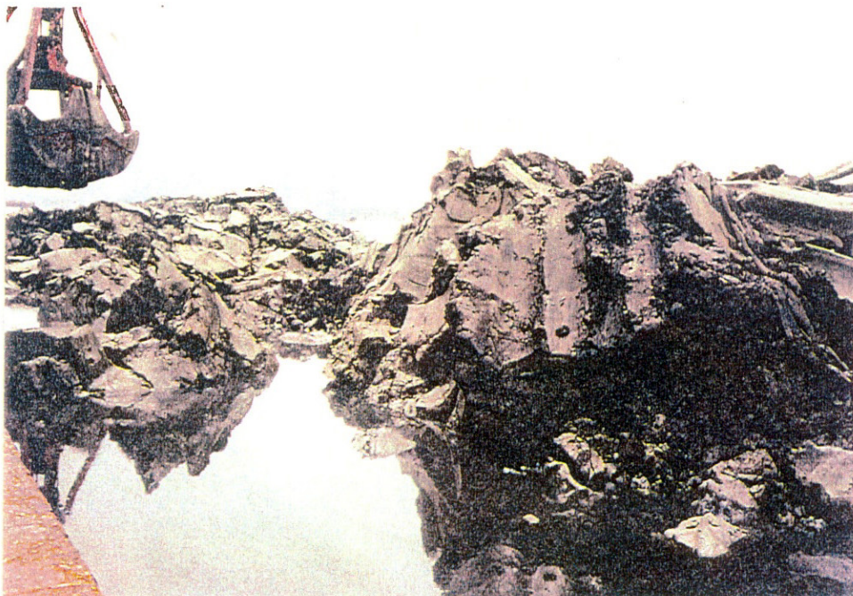
FIGURE 15 Parent Material (Clay) Removed from the Inner Confluence Cell with Traces of Surface Silts
