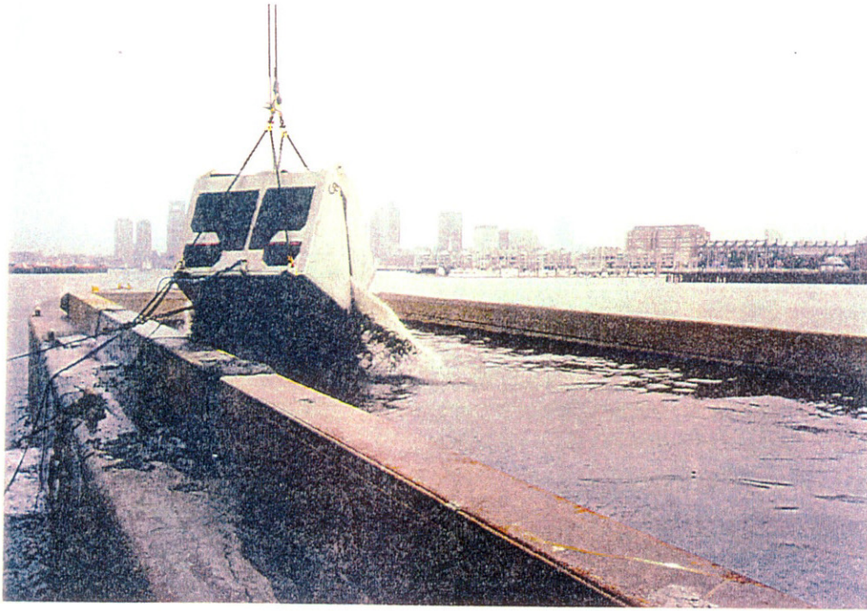
FIGURE 4 Dredging Surface Silts at the Inner Confluence Cell with the Environmental Bucket
