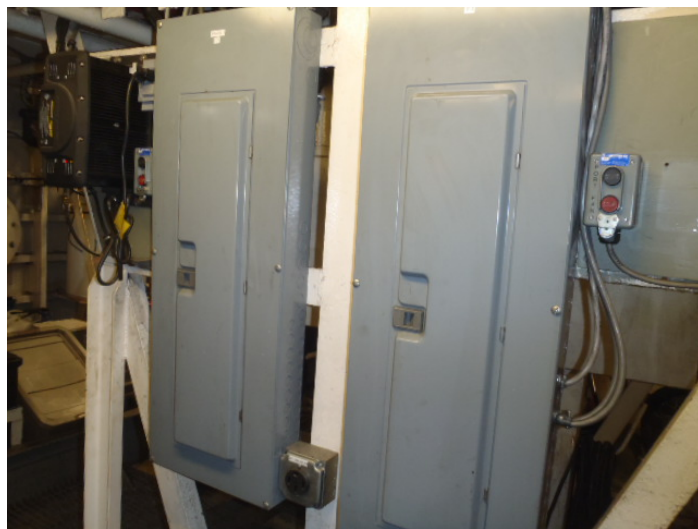
Generator panel and general service breaker boxes
