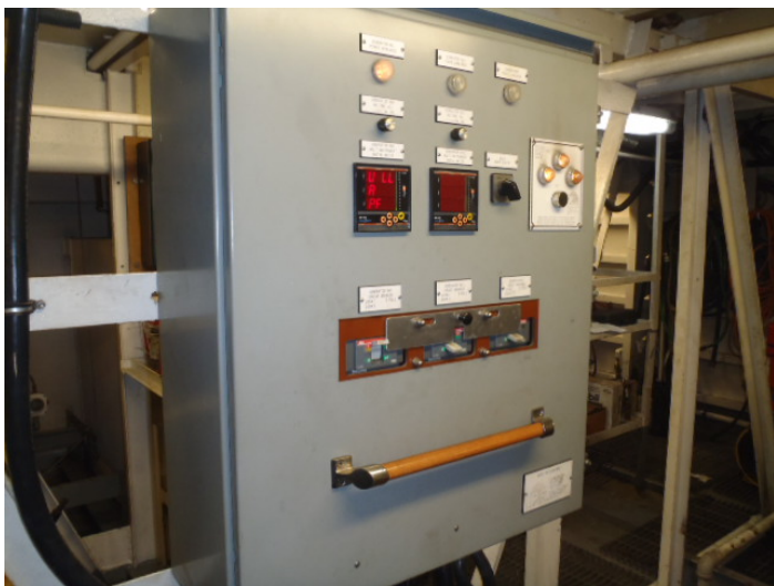
Generator panel and general service breaker boxes
