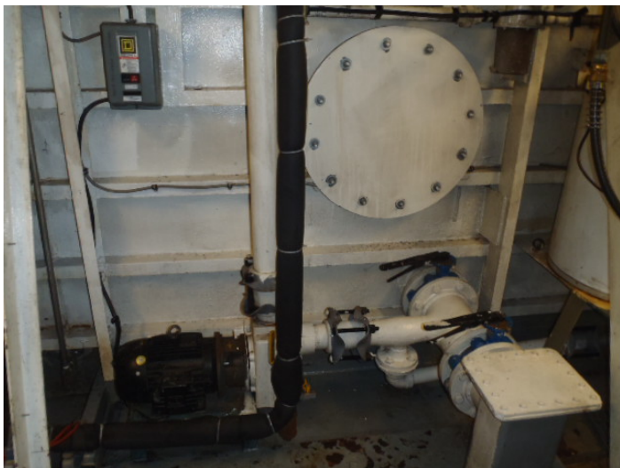
Pump and sea water intake – hatch to side sponson
