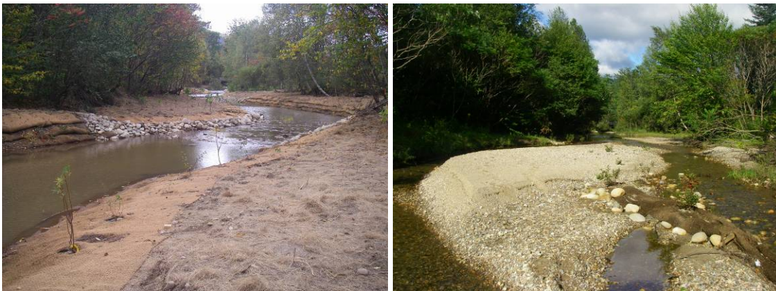
These photographs show the view looking upstream from Station 5+40. They demonstrate the dramatic changes to the channel planform, grade, and cross-sectional geometry between September of 2007 and September of 2009.
