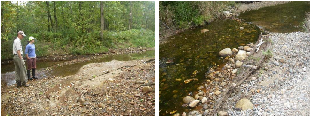
These photographs show examples of where remnants of bank construction using coir cloth were impeding the natural flow of water and sediment in Barkers Brook. MDOT staff removed the fabric in these and other similar areas in September of 2009.
