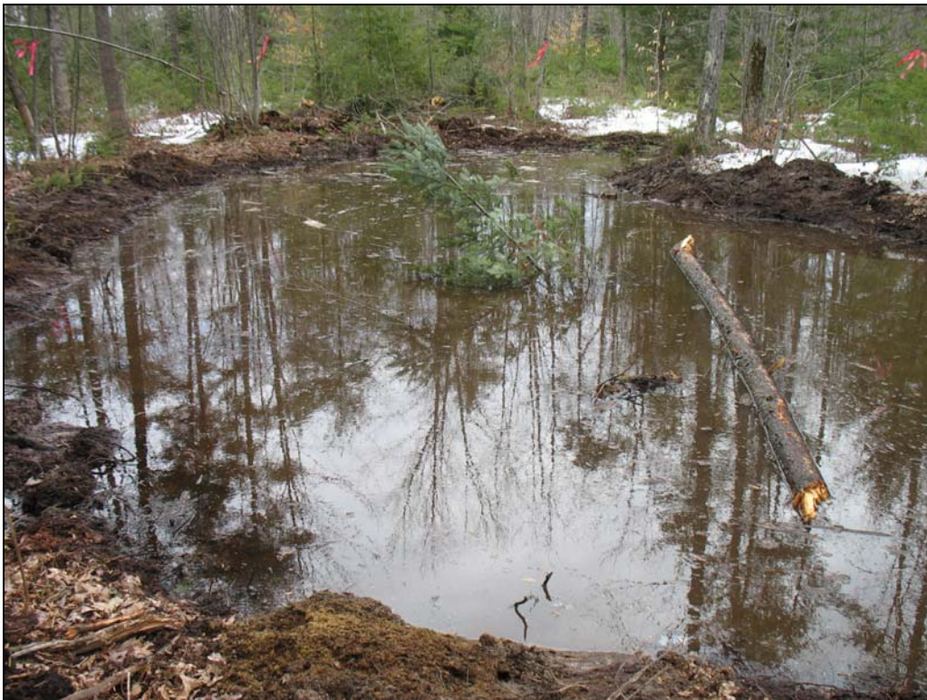
Photolocation 29 (Year of construction). Facing north across a portion of vernal pool 3, 18-March-2007.
