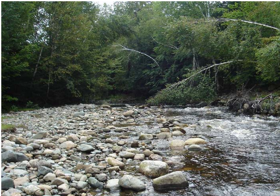
Transect 4 (Station 270, Project Area) looking upstream, August 2006, post-construction. Flow is concentrated in new channel at right of photo. Recently deepened pool is at top of photo.
