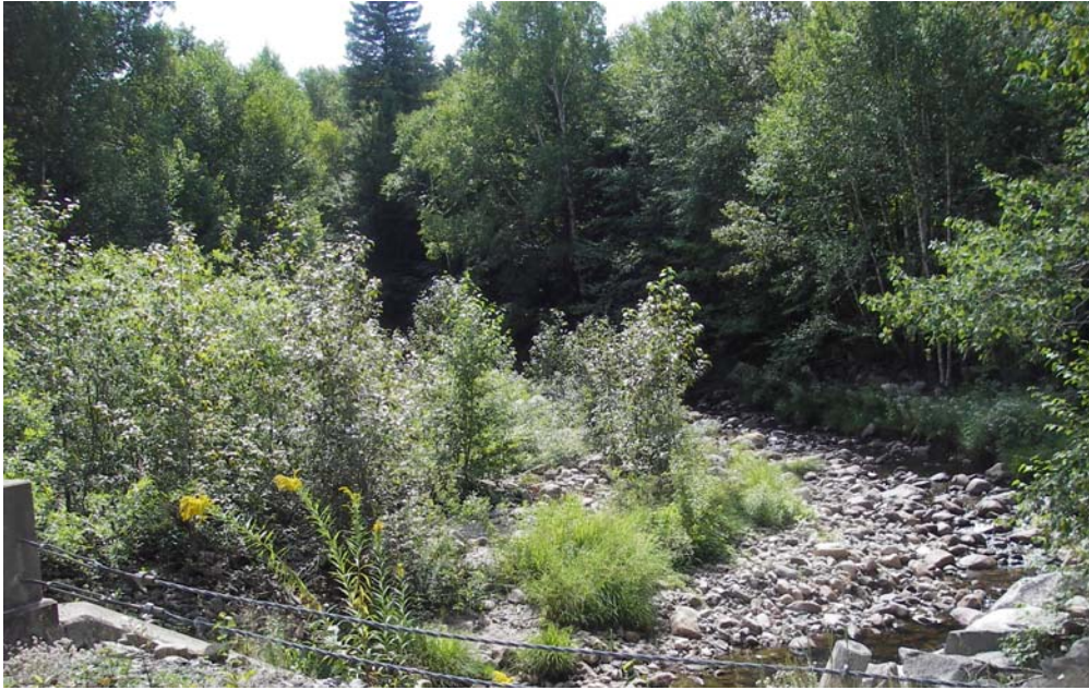
Upstream view from South Shore Drive Bridge prior to restoration, July 2005. 4
