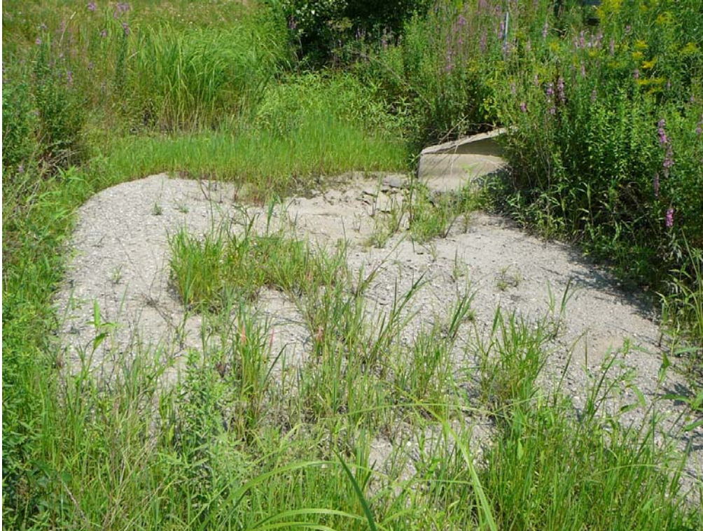
Gravel and sand within sediment forebay of detention basin/constructed wetland
