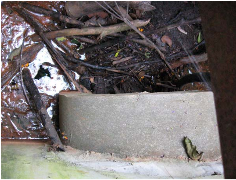
Interior of outlet structure; note: pipe clogged 3-4 inches with debris
