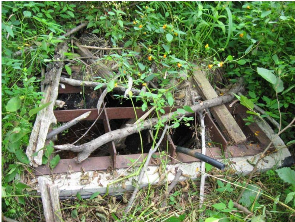
Upstream side of mitigation site outlet structure, dammed by beavers
