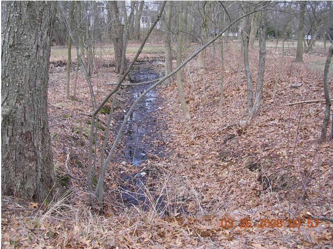
Figure 10-9: Main ditch, looking downstream from cart path crossing toward Fuller Brook.
