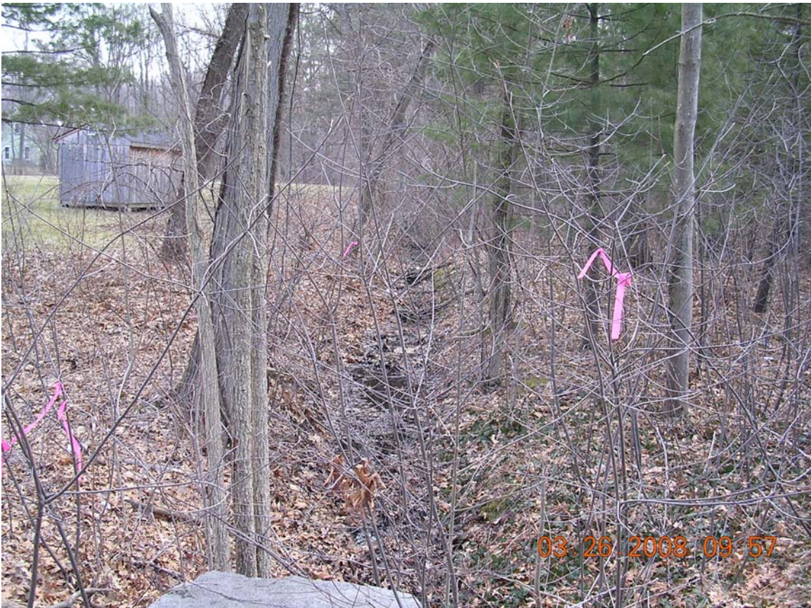
Figure 10-8 Main ditch, looking upstream from Cart Path crossing.
