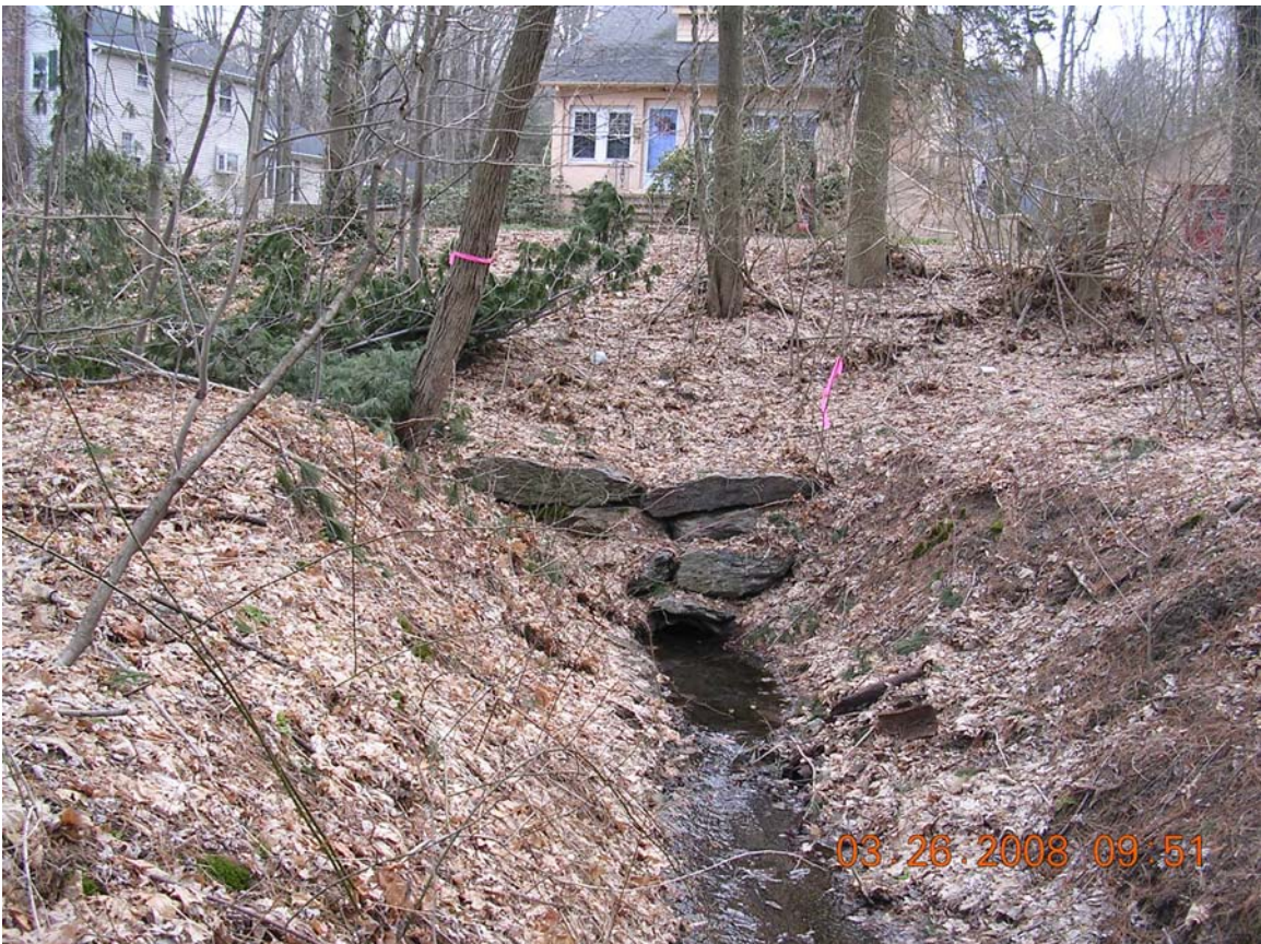
Figure 10-2 The main drainage ditch emerges under Seaver St., looking upstream.
