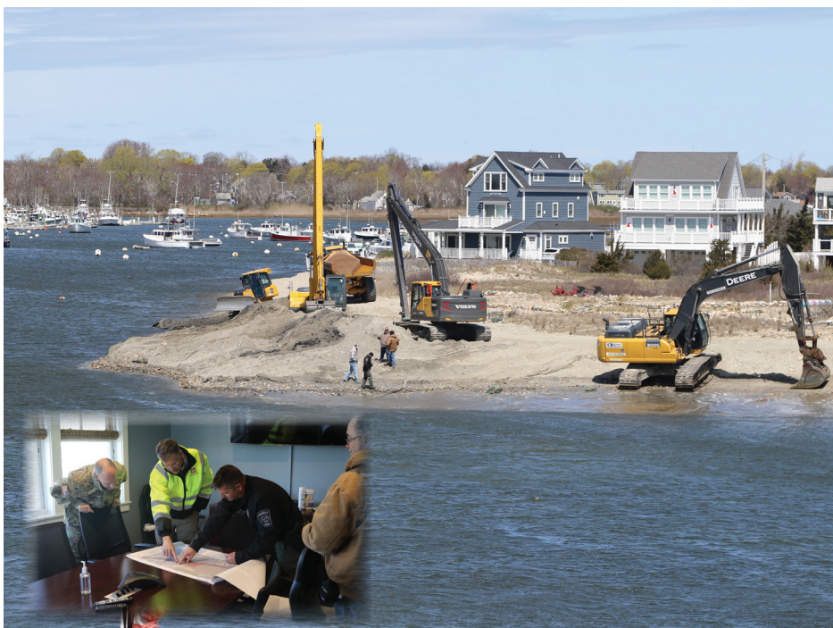
Inset: Lt. Col. Michael Carvelli (left) looks at a map with Scott Acone, Mike DiMeo and Bill Kavanaugh. Above: Landside excavators from Mississippi River Valley Division remove material from Green Harbor Beach.
