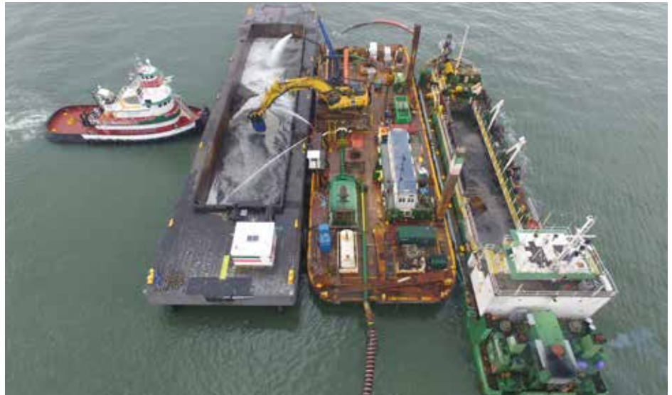
District contractor Cashman Dredging performs work on the Housatonic River.
