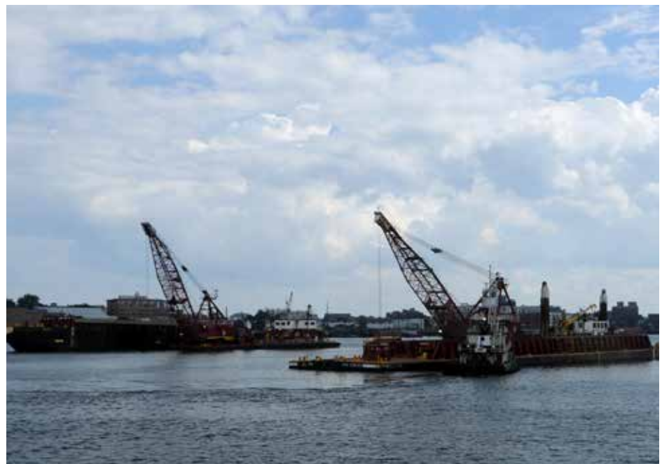
Dredges performing work in Boston Harbor.
