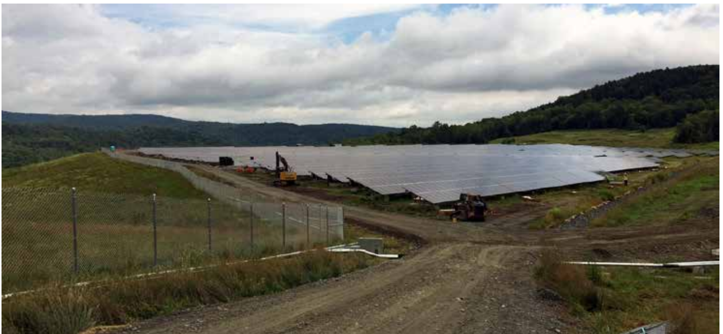
The 43-acre cap at the Elizabeth Mine has been re-utilized by a private firm for a solar array providing enough electricity for about 1,200 homes annually.
