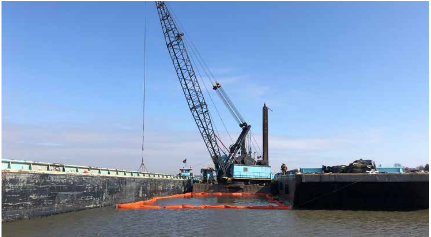
A dredge excavates material from the North Cove Federal Navigation project.
