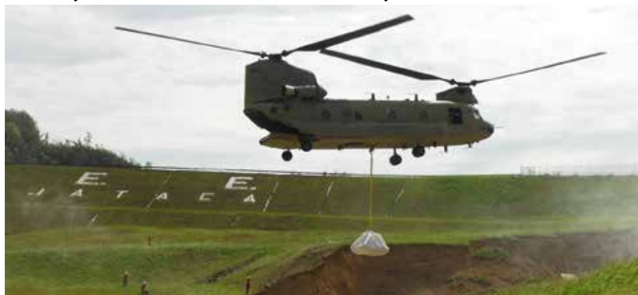
The Army National Guard places sandbags at the Guajataca Dam.
