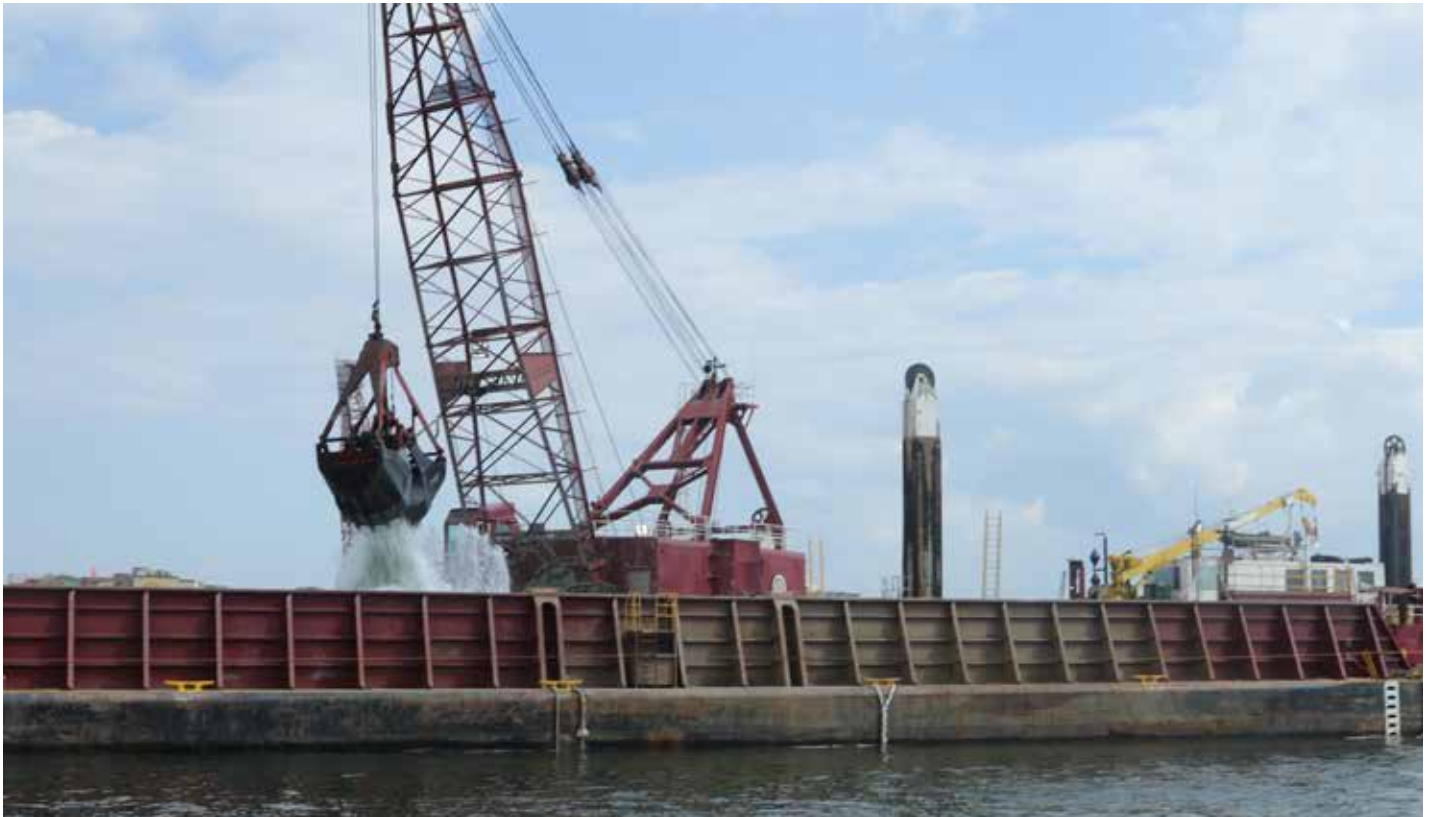
A clamshell dredge performs maintenance work in Boston Harbor.
